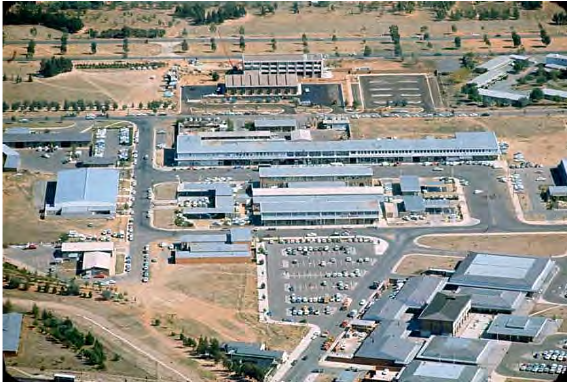
Dickson Centre in the early 1970s, looking westward – (Photo courtesy ACT Heritage Library, Department of Capital Territory Collection)
