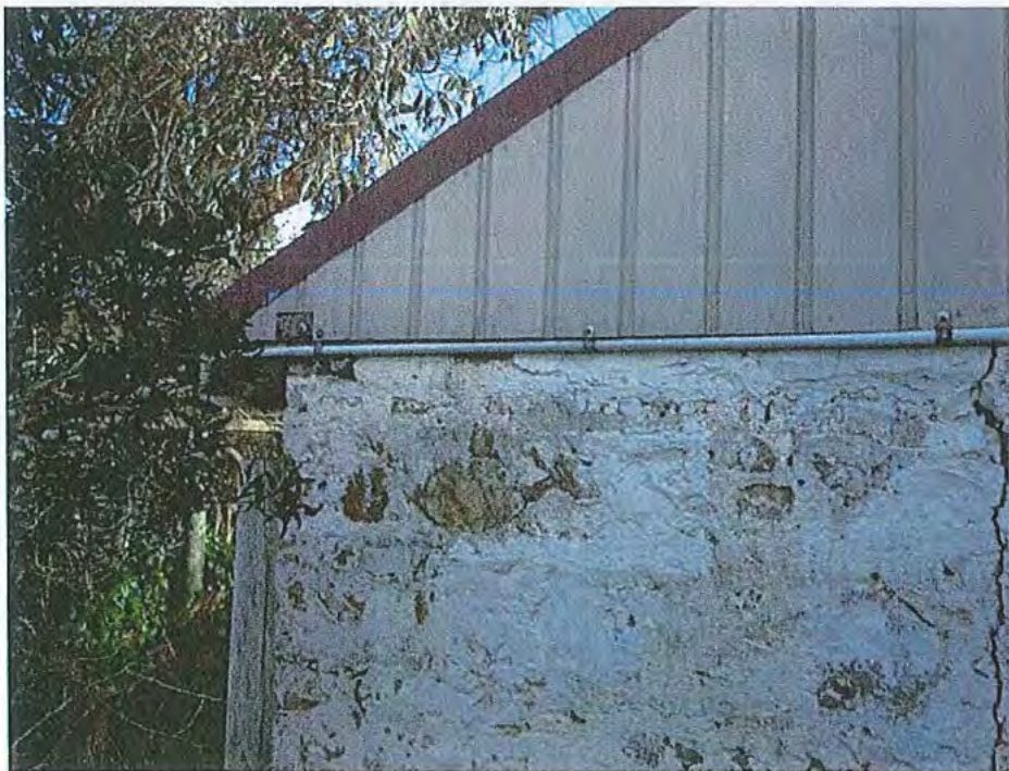
Photo4: East end gable
