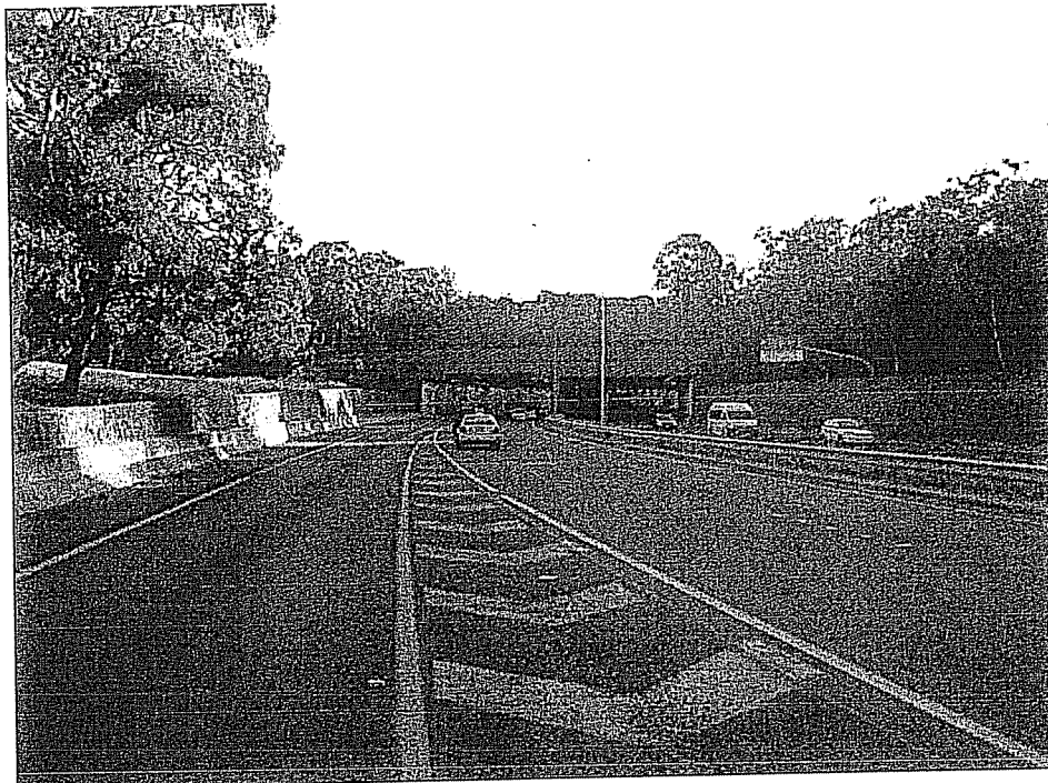
Figure 2: Westbound view from SSD
