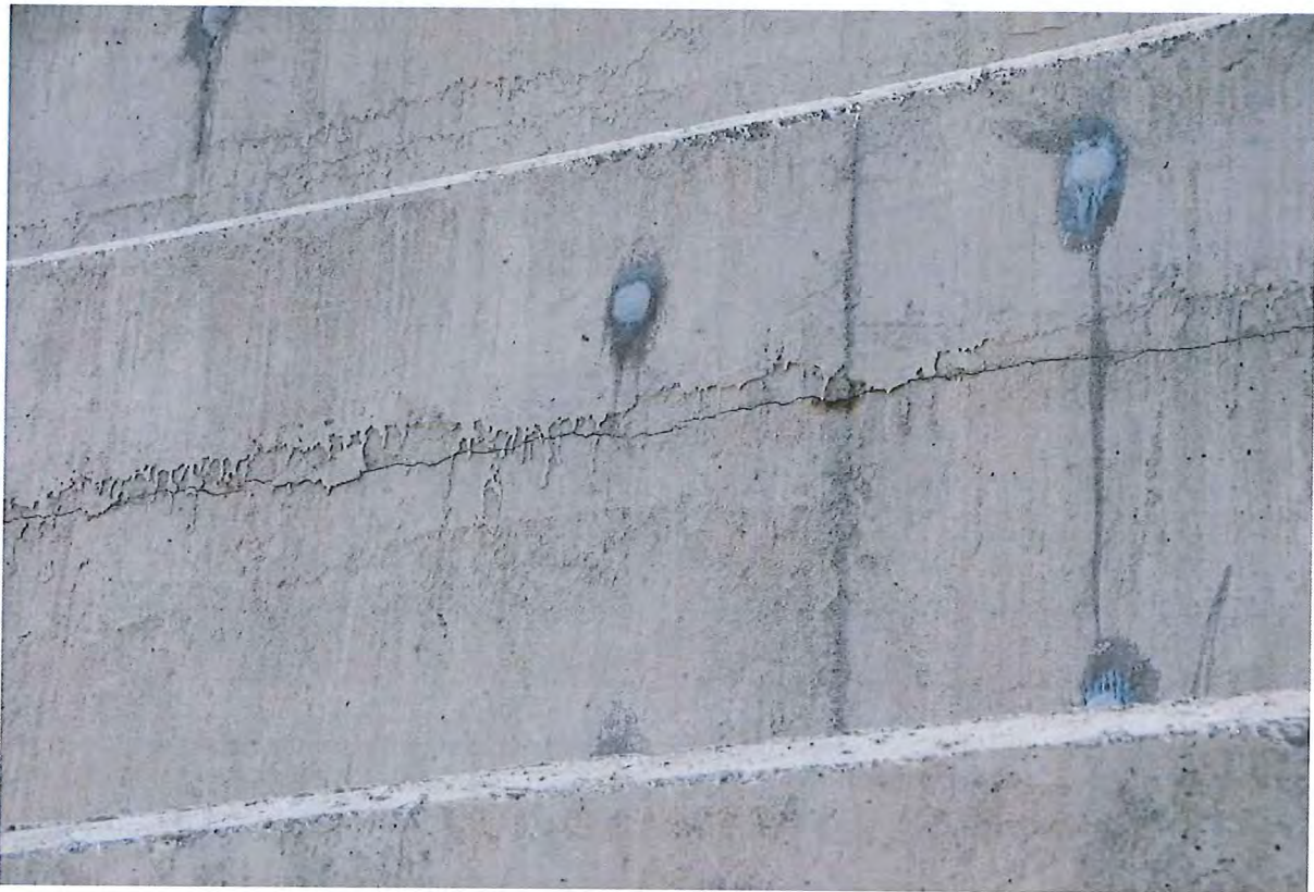
Photograph 5.5 The higher of the two horizontal cracks on the downstream face, which seems to be along an RCC lift joint. It is on the vertical face of the step at RL 485.3.
