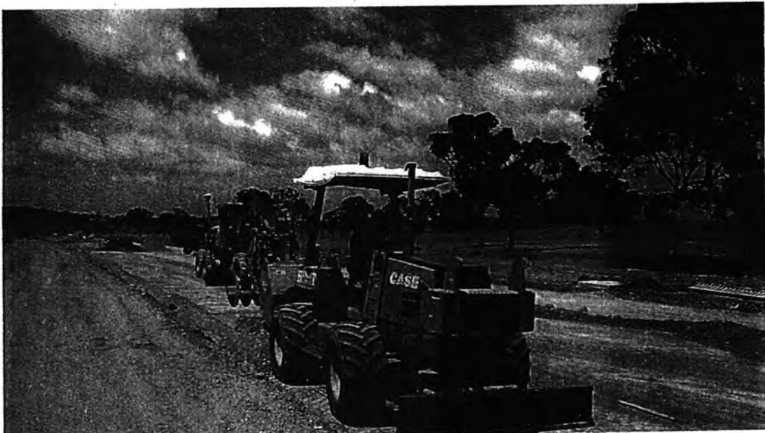
Image 02: Trenching for subsoils east of Road 04 Intersection
