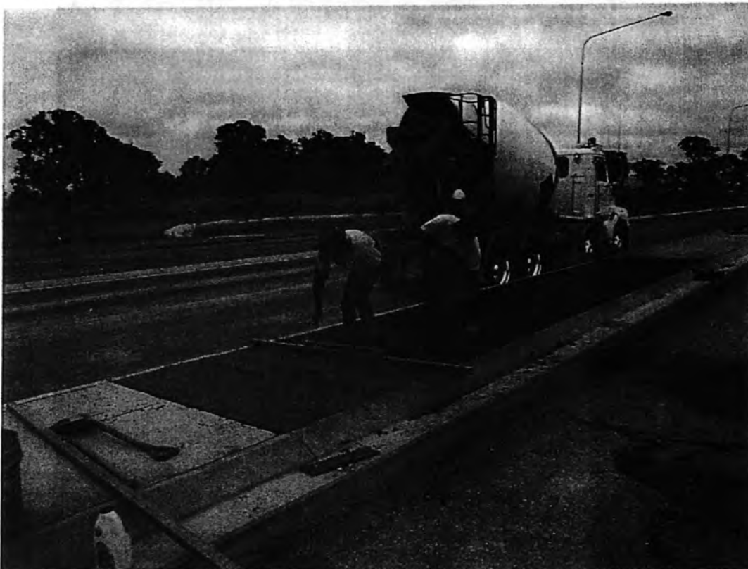
Image 04: Placement of concrete for islands west of Mirrabei Dr.
