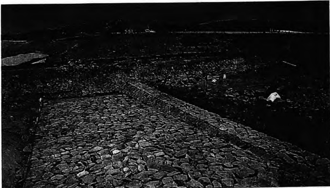
Image 03: Stone pitching at western side of bridge
