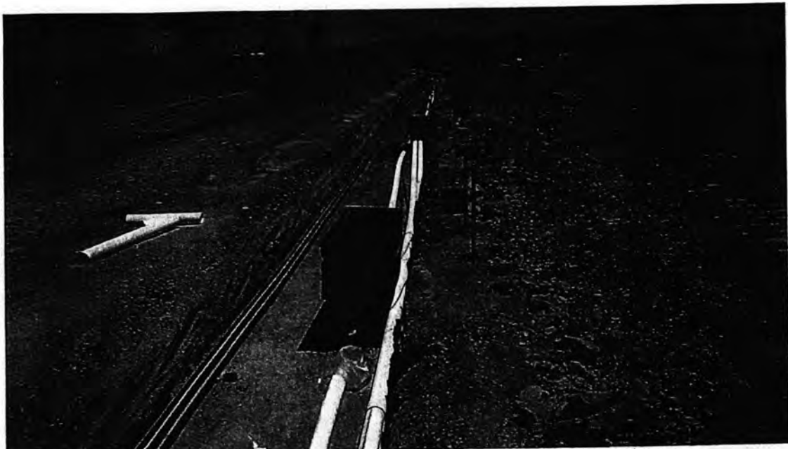
Image 04: Gas pipe and NBN conduits, CH 1200
