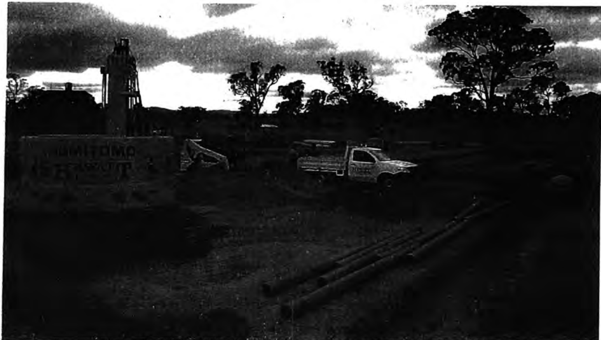
Image 02: Traffic light conduits being placed at Mirrabai Dr Intersection
