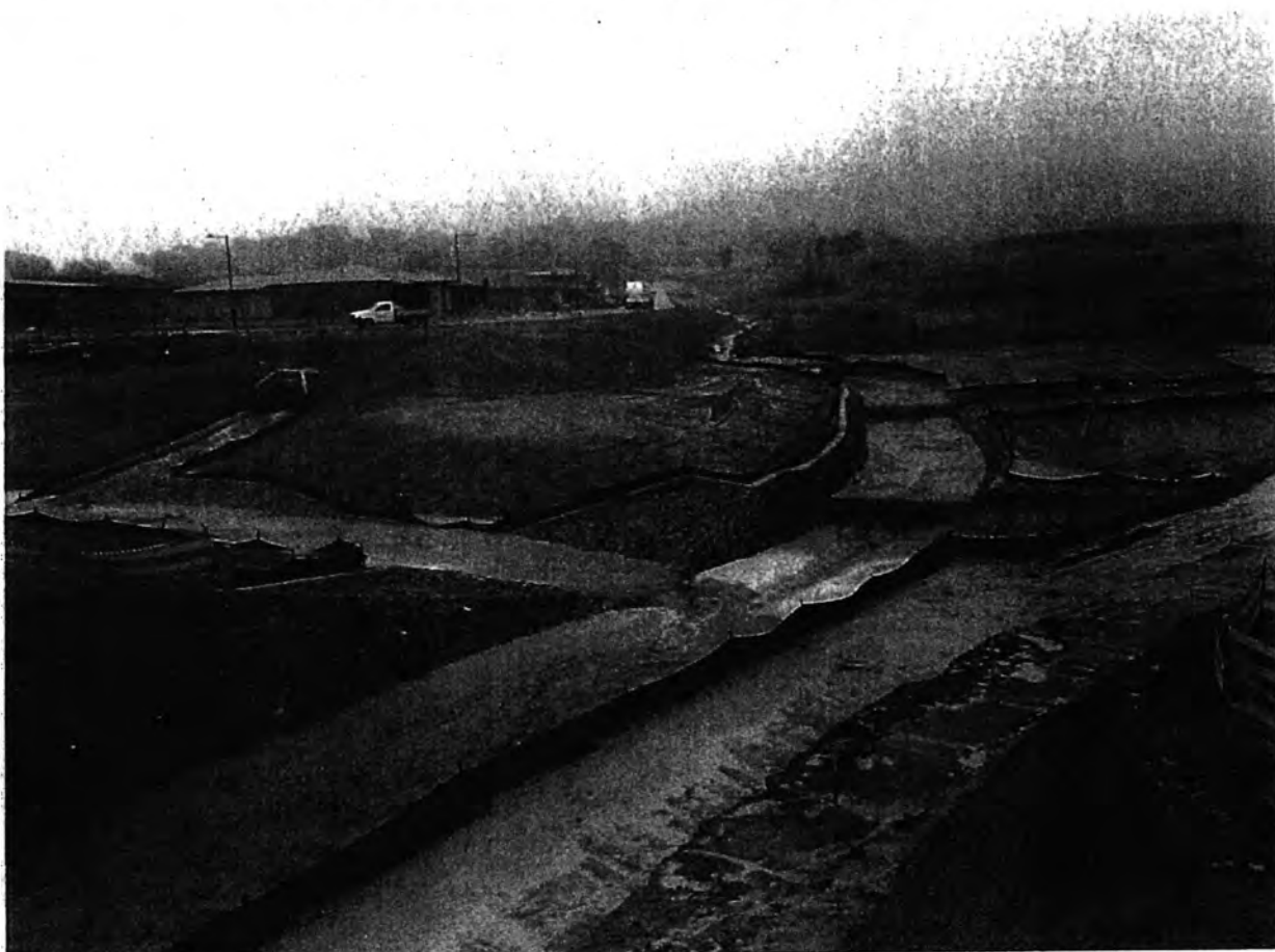
Image 02: Stone-pitching on Casey side of bridge (during rain event, 19.02.2014)
