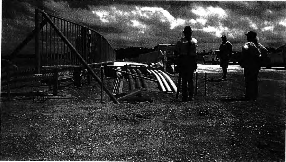
Image 01: Dry-fitting of pedestrian fencing at bridge
