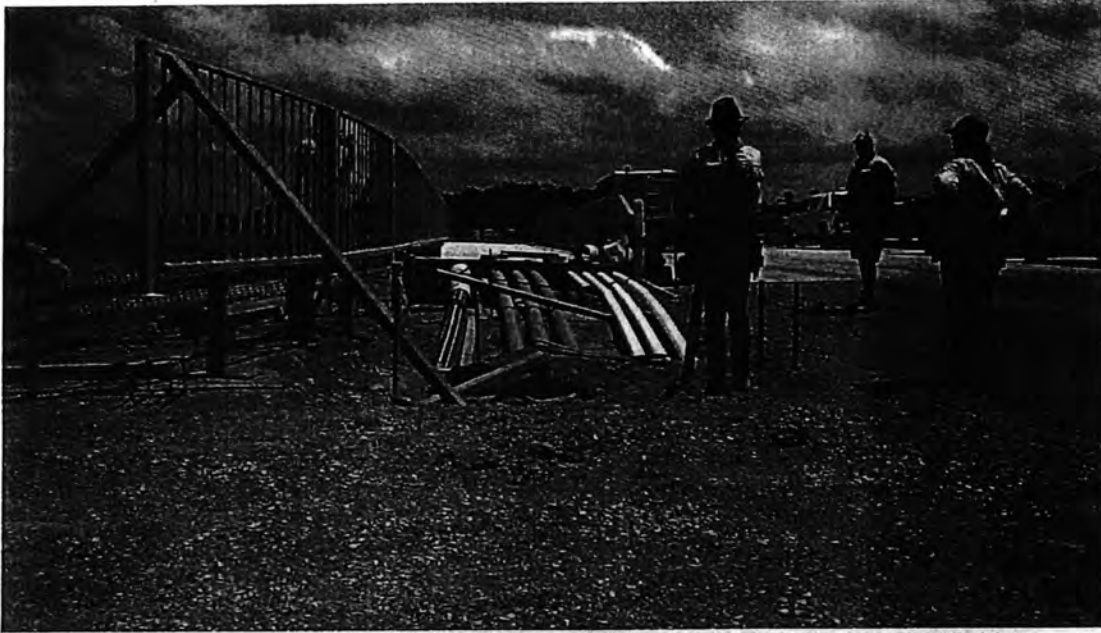
Image 03: Level issues with the transition of footpath and pedestrian handrail at bridge (RF1097A)
