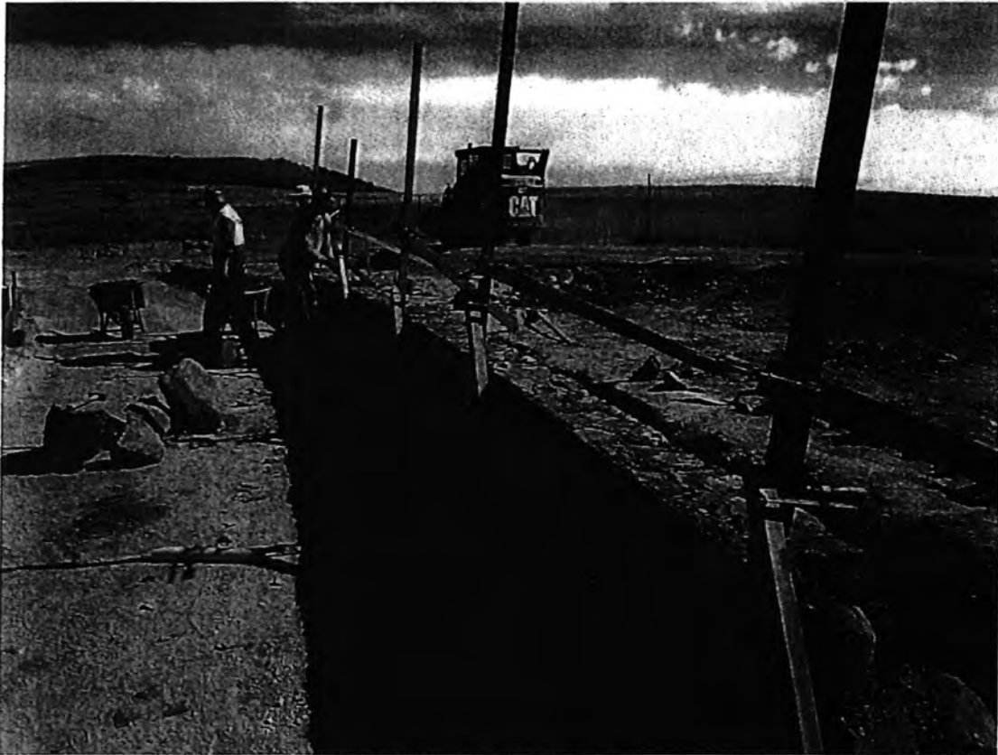
Constructing the equestrian/dhared path retaining wall
