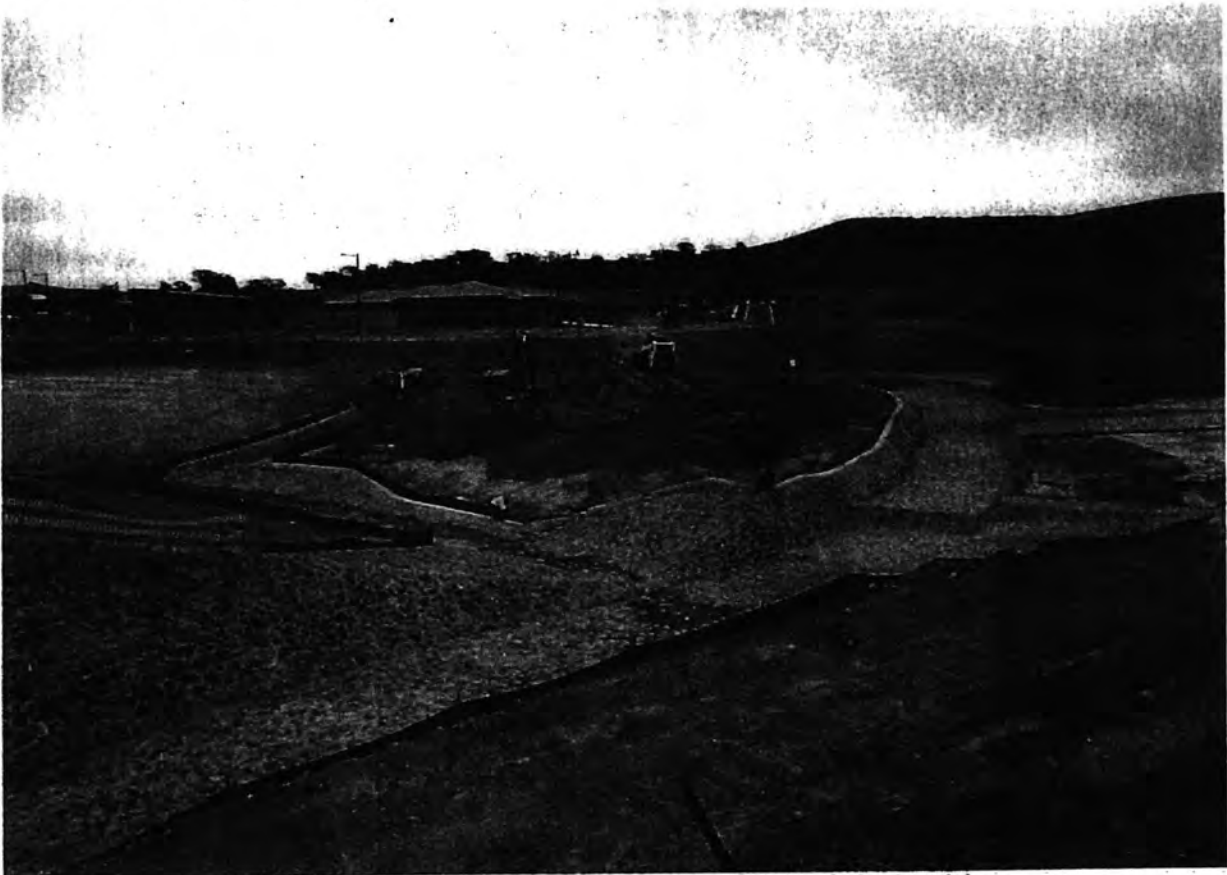
Image 01: Stone-pitching on Casey side of bridge (prior to rain)
