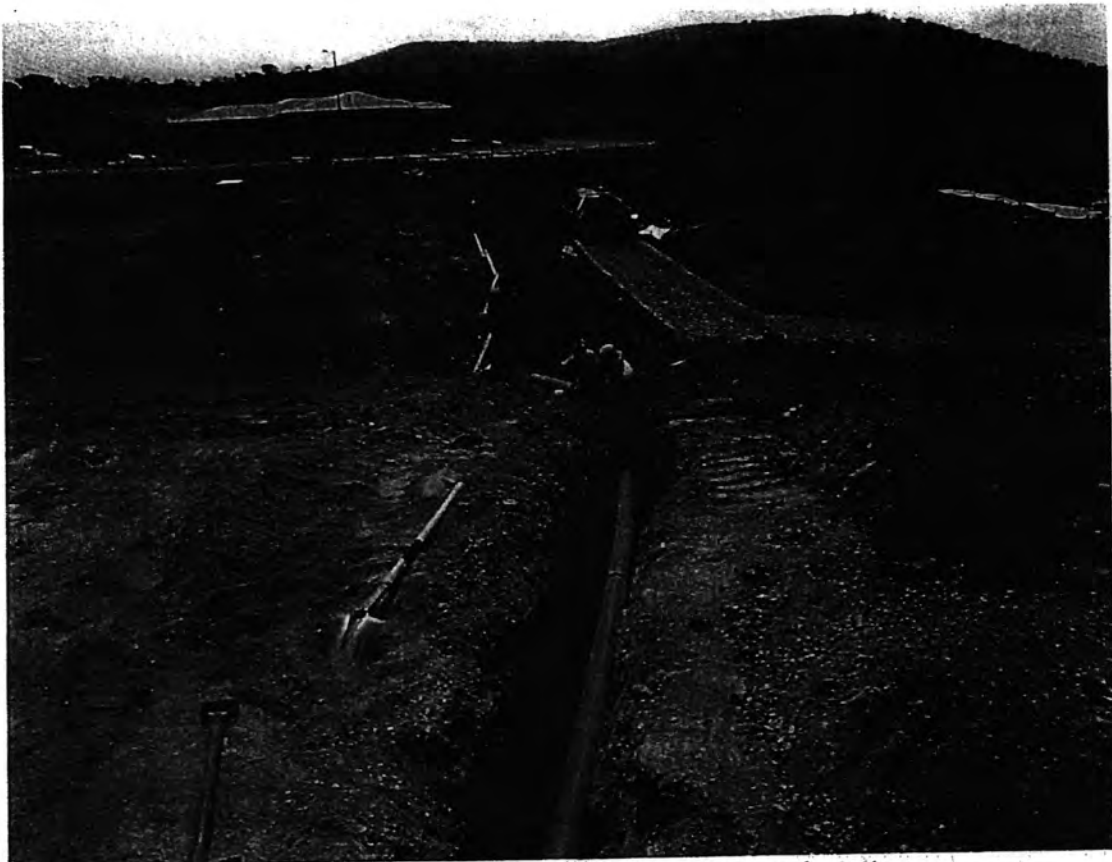
Installation of conduits for street light power supply from Casey sub station
