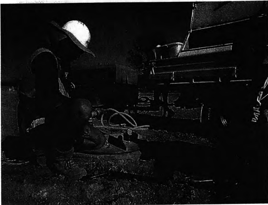
Sewer manhole vacuum test at S19
