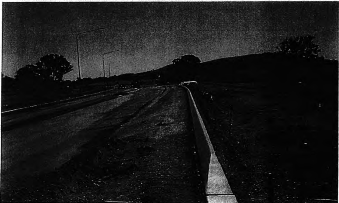
Mountable Kerb at HPD1 interface with HPD2
