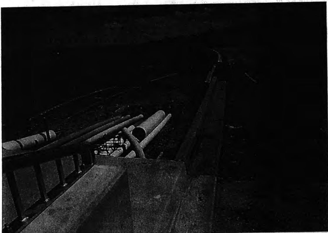
Kerb transition from bridge SFK at CH410
