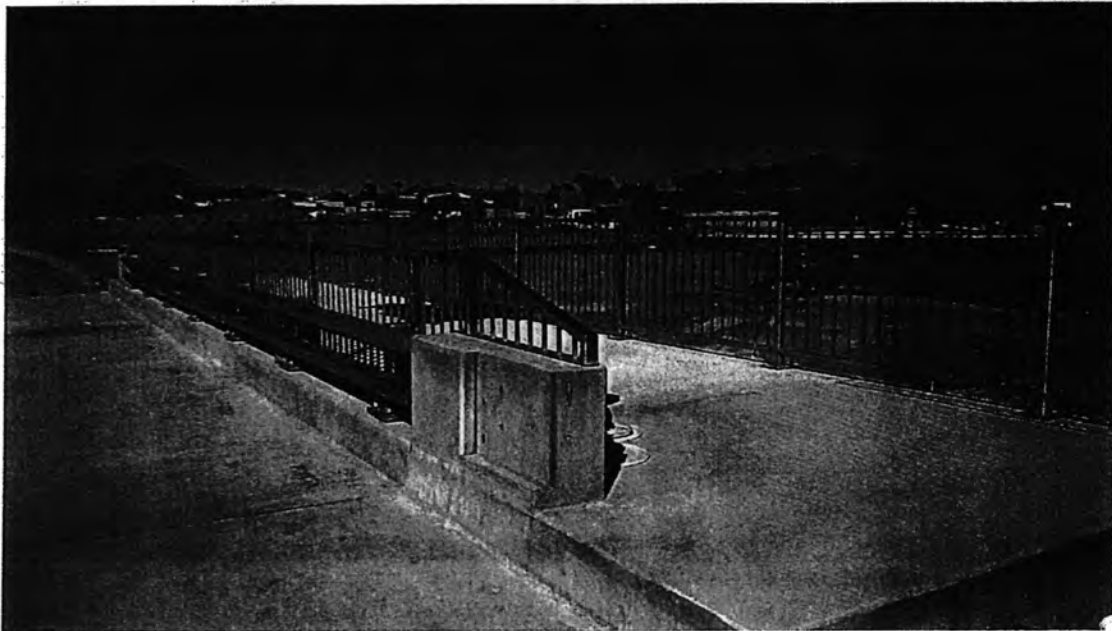
Image 02: Guardrail and handrail installation on bridge
