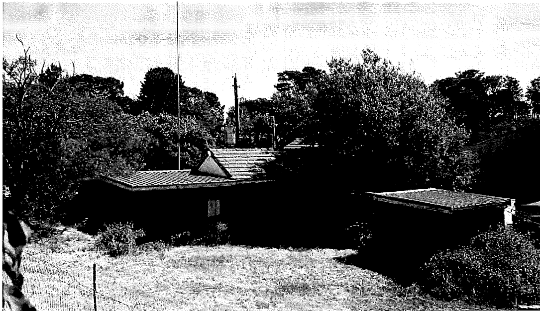
Figure 81 East and north elevations, showing the extent of the additions. The only portion of the original two-roomed structure, not enclosed by additions is indicated by the arrow.
