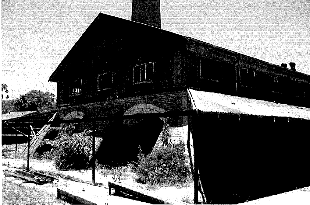
Figure 103 The Hardy patent kiln, showing the west end and part of the south elevation. Note the verandah cladding has been removed and the kiln wall part removed, presumably for improved access to the kiln interior.
