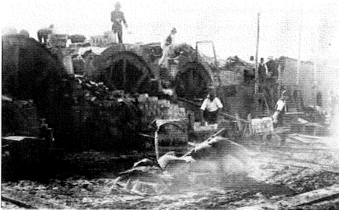
Figure 32 Constructing the transverse arches of the Staffordshire kiln, c. 1915. Source: National Library of Australia.
