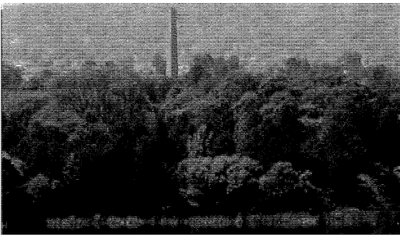
Figure 105 The Chimney stack viewed from across Yarramundi Reach, Lady Denman Drive.
