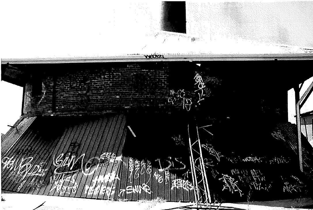
Figure 17 Hoffman kiln at the former Standard Brickworks, Box Hill (Victoria) Source: Lovell Chen, January 2010
