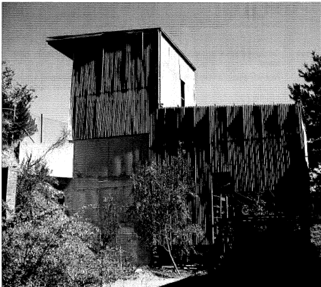
Figure 124 Small Crusher House viewed from the north.
