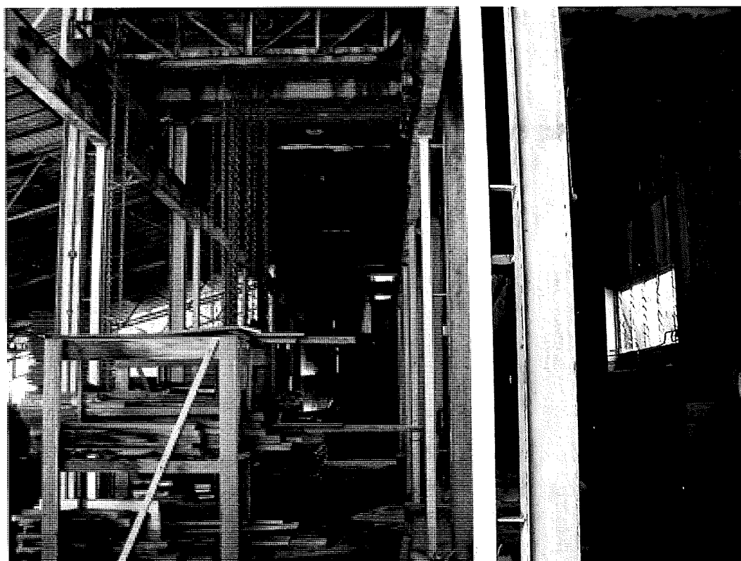
Figure 118 Interior of the Machine Bay III shop floor, looking north.
