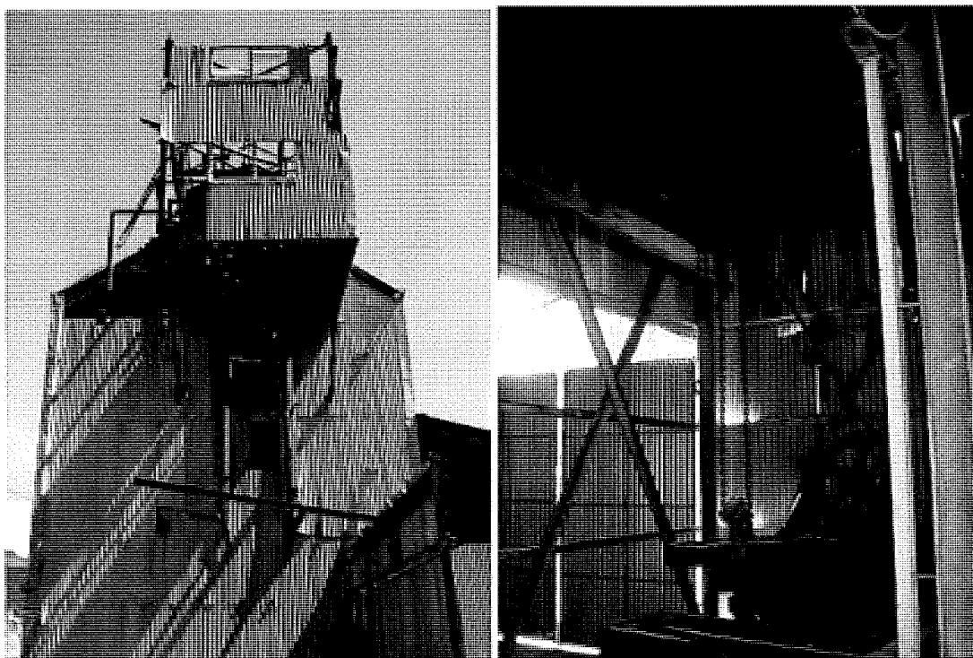
Figure 117 From left: north end Machine Bay III showing remains of headgear housing for the loft conveyor; interior with remnants of the Anderson brick machinery at north end.
