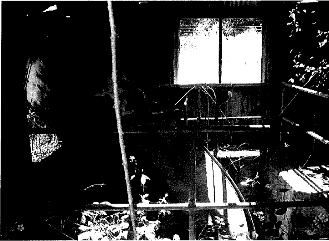
Figure 90 Interior of the 1927 fan house.
