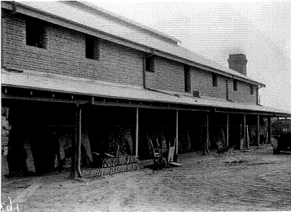
Figure 52 The north elevation, photographed prior to the rebuilding of the verandah to support a first floor enclosed verandah structure. Source: National Archives of Australia.
