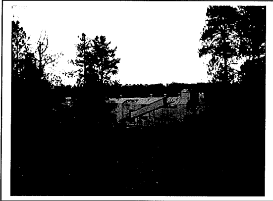
Photograph 1: West view of crusher area.
