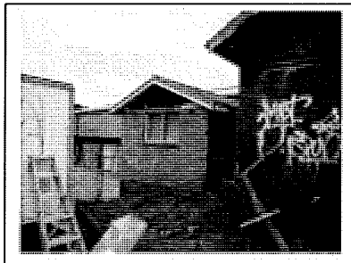
Photograph 1: Building prior to commencement of asbestos removal.
