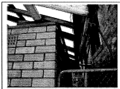
Photograph 4: Building at the completion of asbestos removal works.
