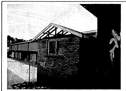
Photograph 2: Building at the completion of asbestos removal works.
