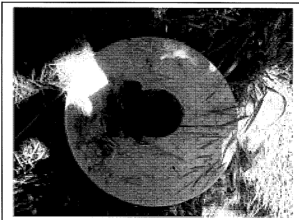
Photograph 34: Dip point to probable UST
