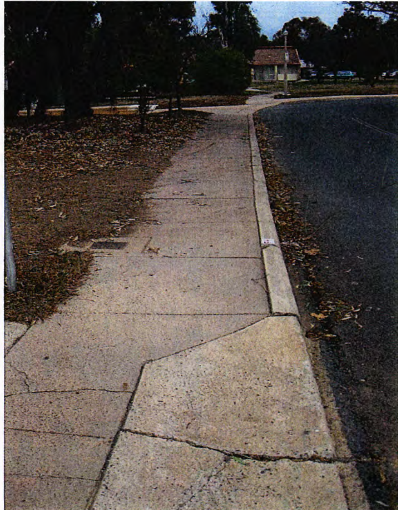
Figure 2.1: Section of Rivett Place kerb adjacent to Block 13
