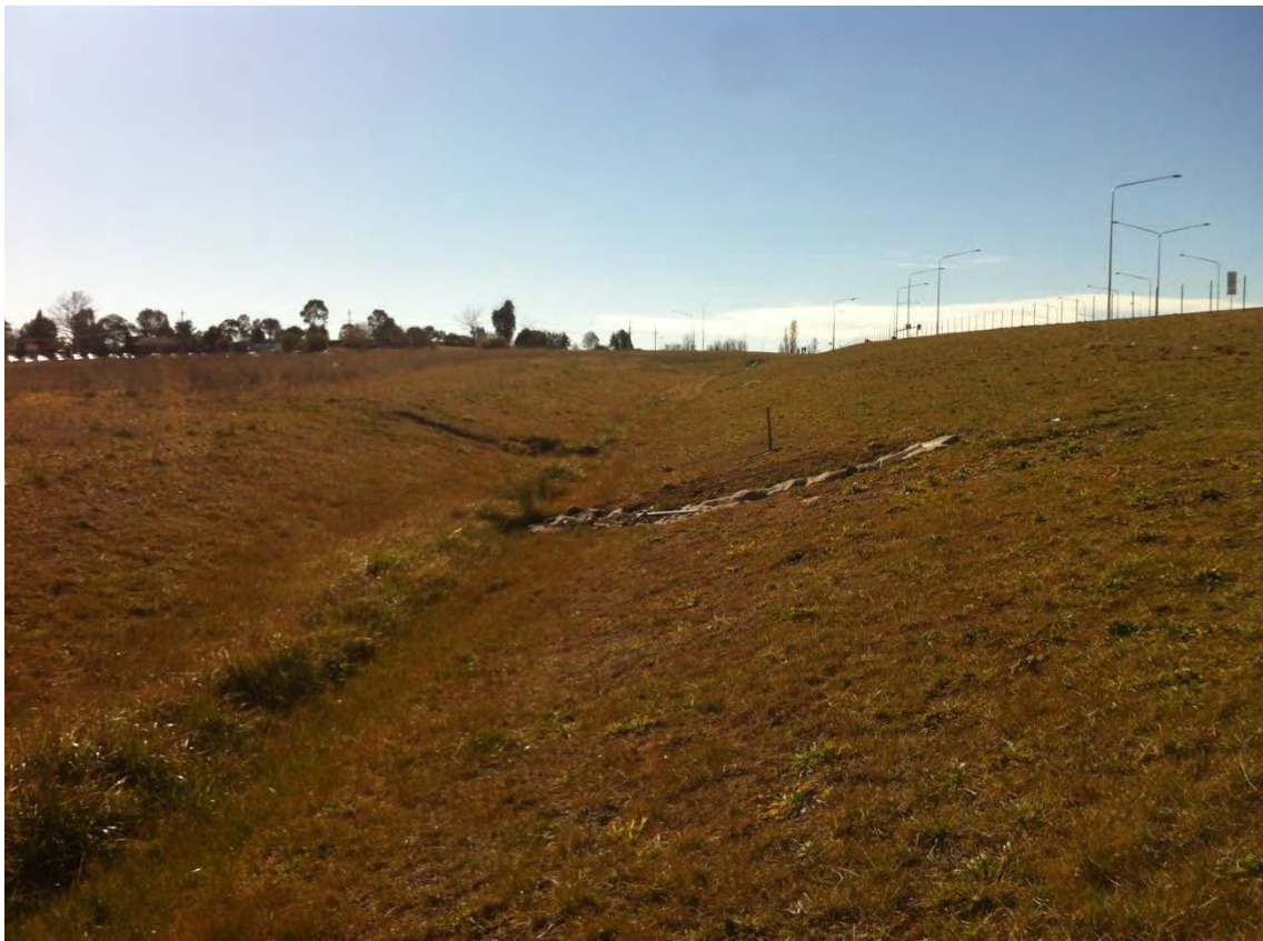
Block 1218 Existing Stormwater Outlet and Channel
