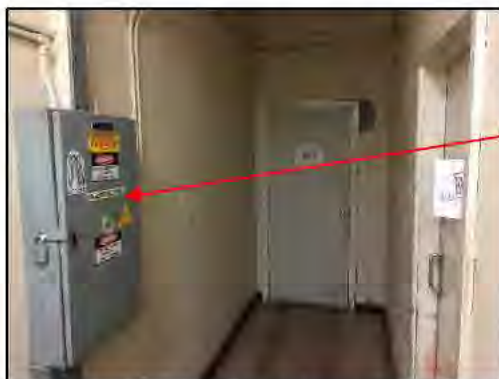
Switchboard DB13 in exit travel path
