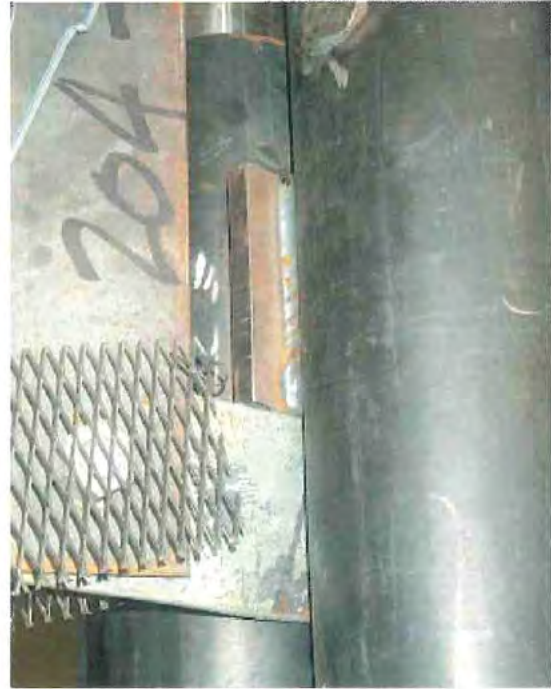
End plate during test
