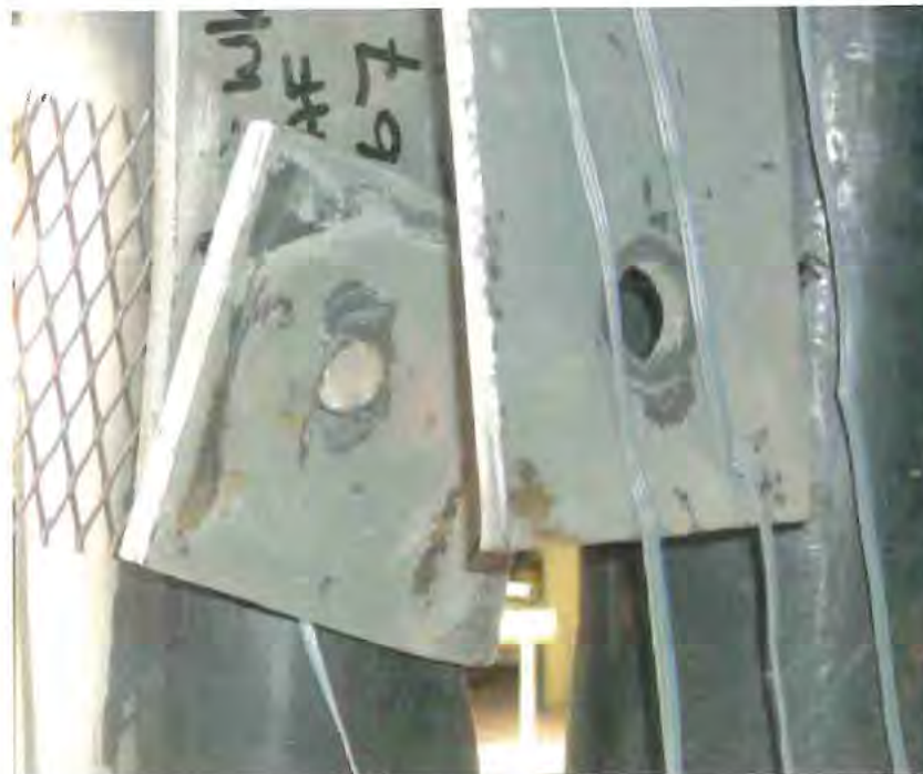
Figure 19 – Failure Mode of Specimen 1
