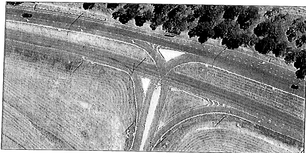
Figure 1 Coppins Crossing Road / William Hovell Drive Intersection
