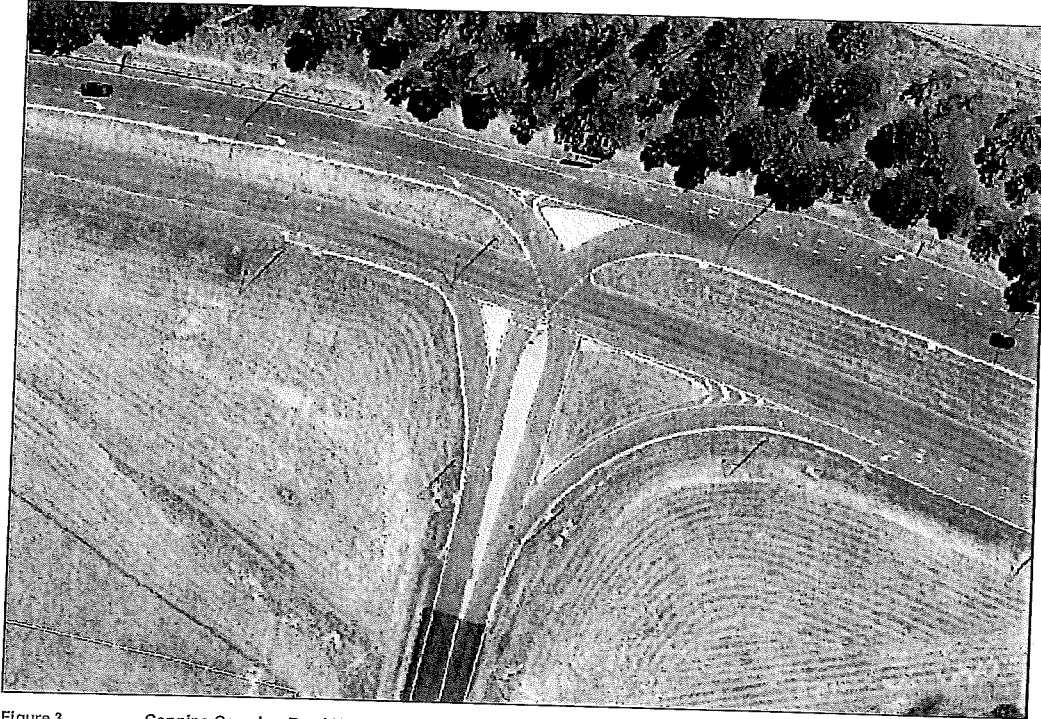
Figure 3 Coppins Crossing Road / William Hovell Drive Intersection
