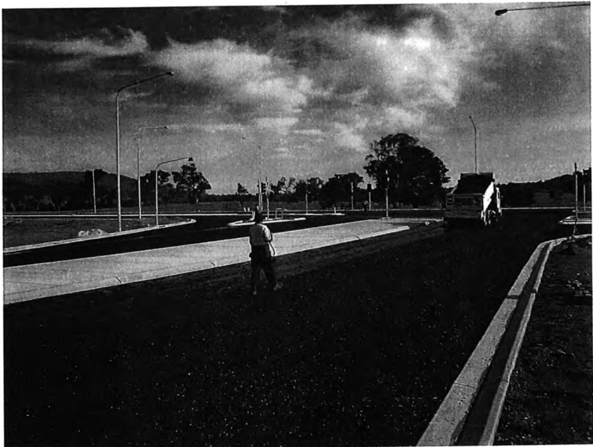
Placement of two coat 14/7 seal at Mirrabai Drive intersection
