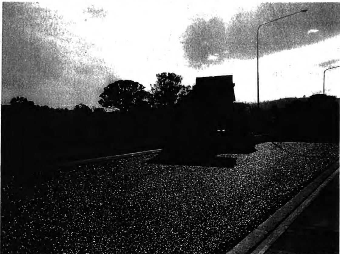
Image 02: Aggregate being spread for 14/7mm seal between Road 04 and Mirrahei Dr
