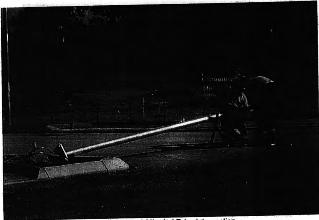
Cabling and installing street light poles at Mirrabai Drive intersection
