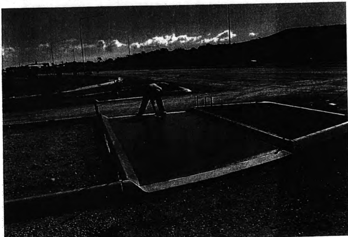
Constructing pram crossing at Road 4 intersection
