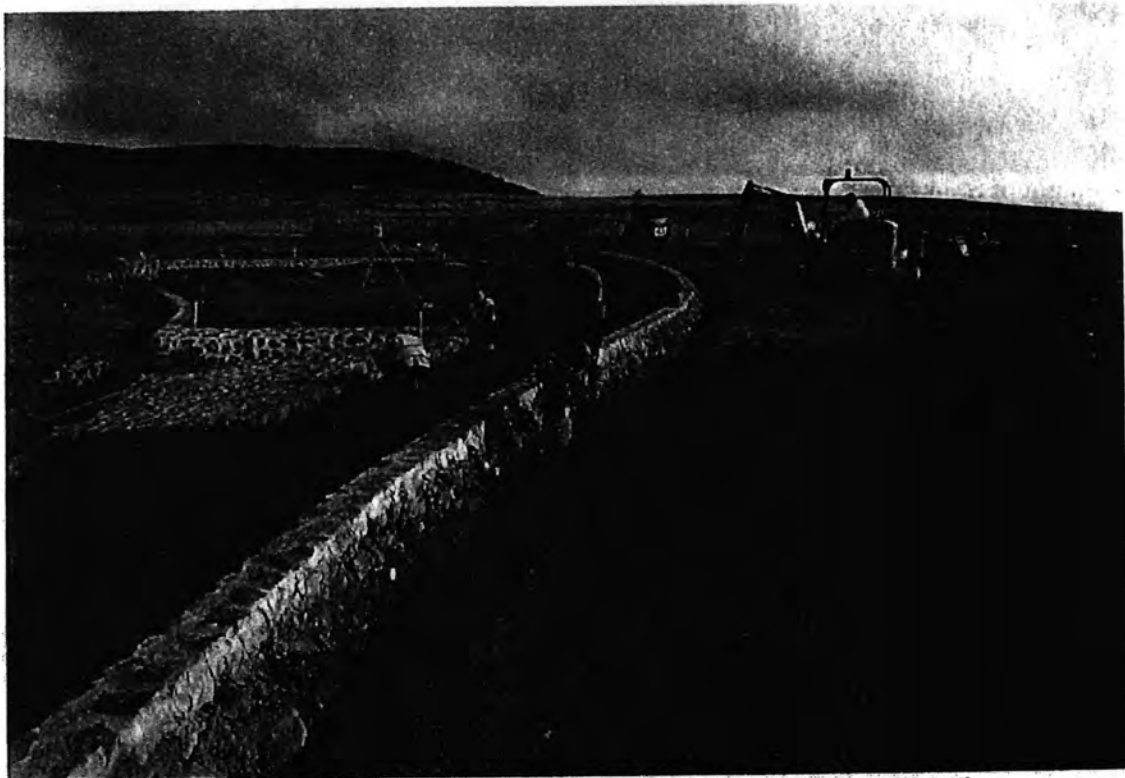
Back filling against the stone pitched retaining wall at the equestrian/shared path
