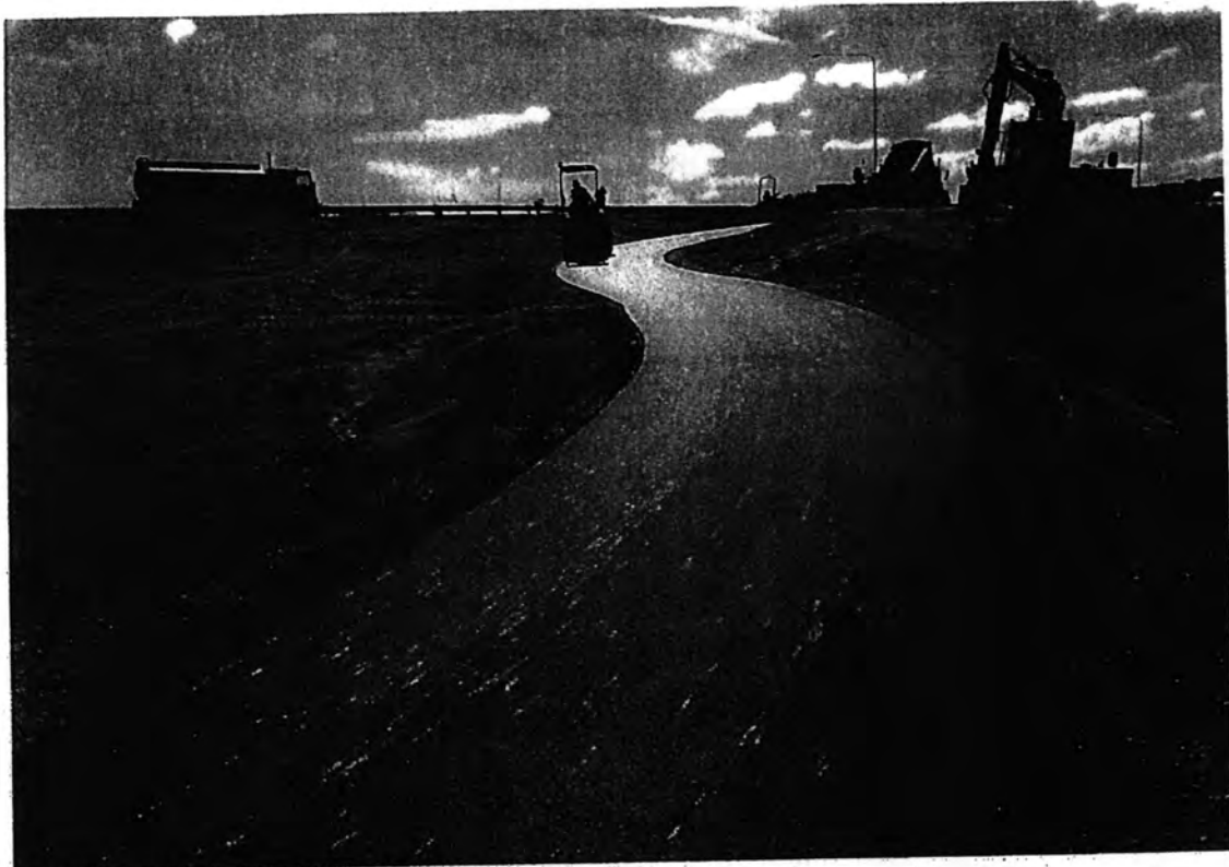
Placement FFG asphalt on the shared path
