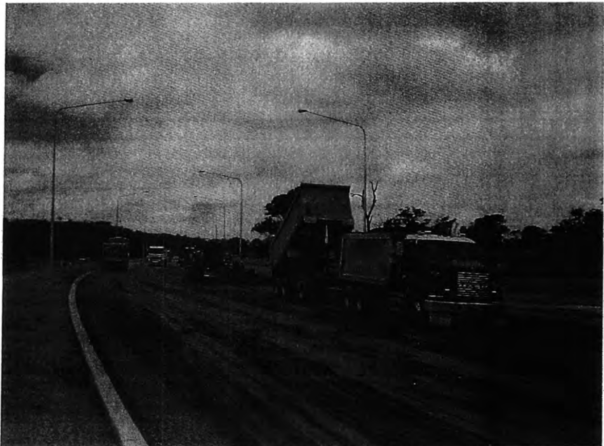
Image 02: Placement of base material
