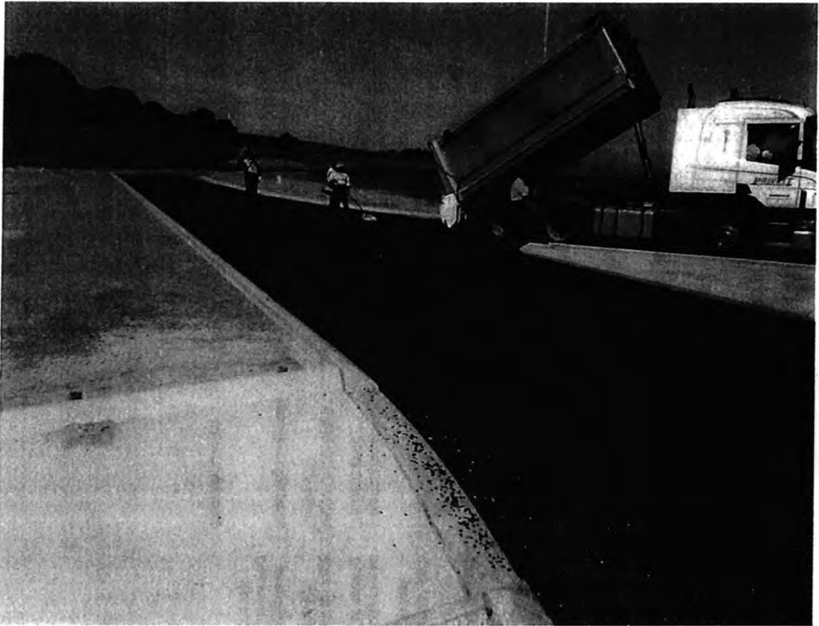
Image 01: 7mm aggregate being placed at Road 04 Intersection for two-coat seal
