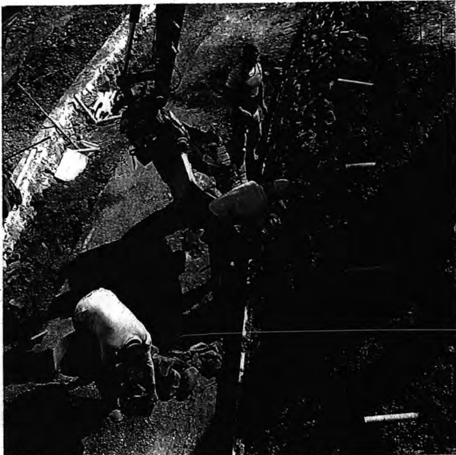
Placing stone pitching adjacent to shared path CH60
