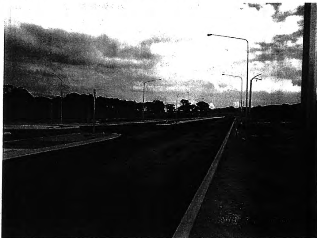
Image 02: Priming completed from HPD1 to Road 04 Intersection
