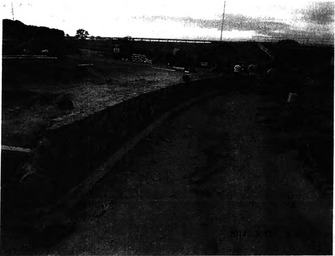
Image 01: Stone pitched wall dividing shared and equestrian path
