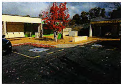
Accessible car parking spaces with shared pram ramp compliant with earlier codes
