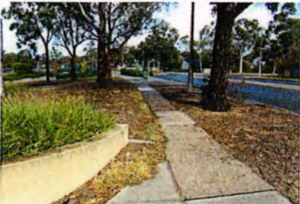
Bangalay Crescent footpath access to bus stop/shelter (in middle of photo).
