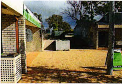
Gap between shops leading to bus stop/shelter, with an option of steps or a ramp leading to a pathway connecting to the footpath along Bangalay Crescent
