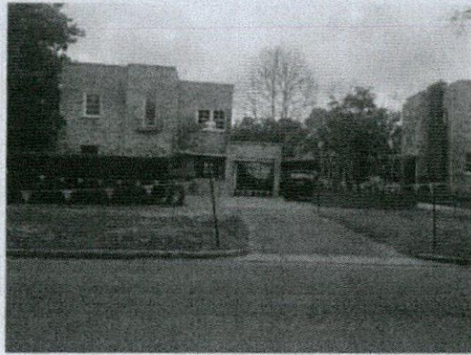
4: Photograph of property post removal of original fence and installation of rendered fencing - June 2013 (prior to windows being replaced).
