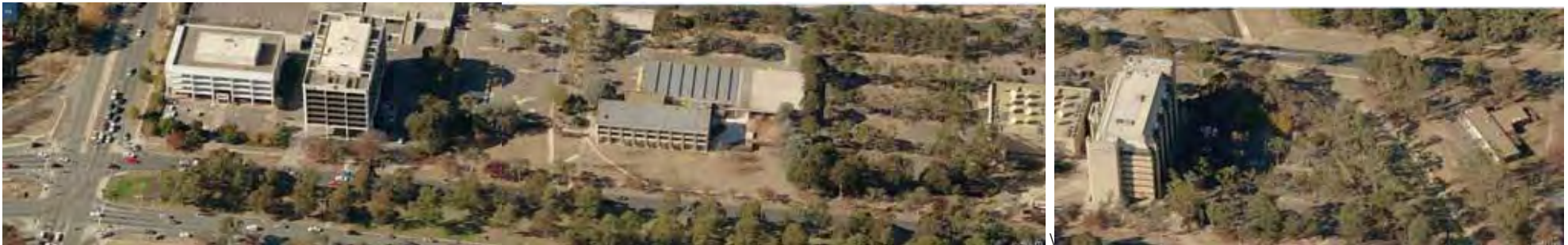
Dickson Centre 'edge' along Northbourne Avenue showing large building masses with substantial separation between buildings
