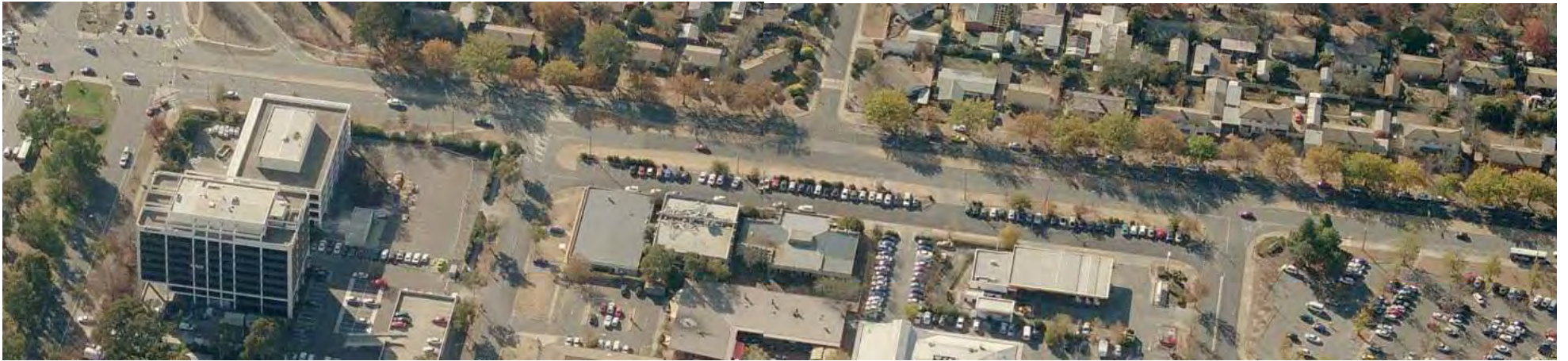
Dickson Centre 'edge' along Antill Street showing the interface between the centre and residential dwellings in Downer (Note: photo taken before demolitions of buildings on former ACTTAB site)
