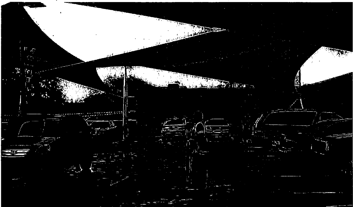
Figure 8: Roof top shaded parking at Aldi's Auburn store. The parking deck could be designed to accommodate other mixed use developments as land economics change over time.
