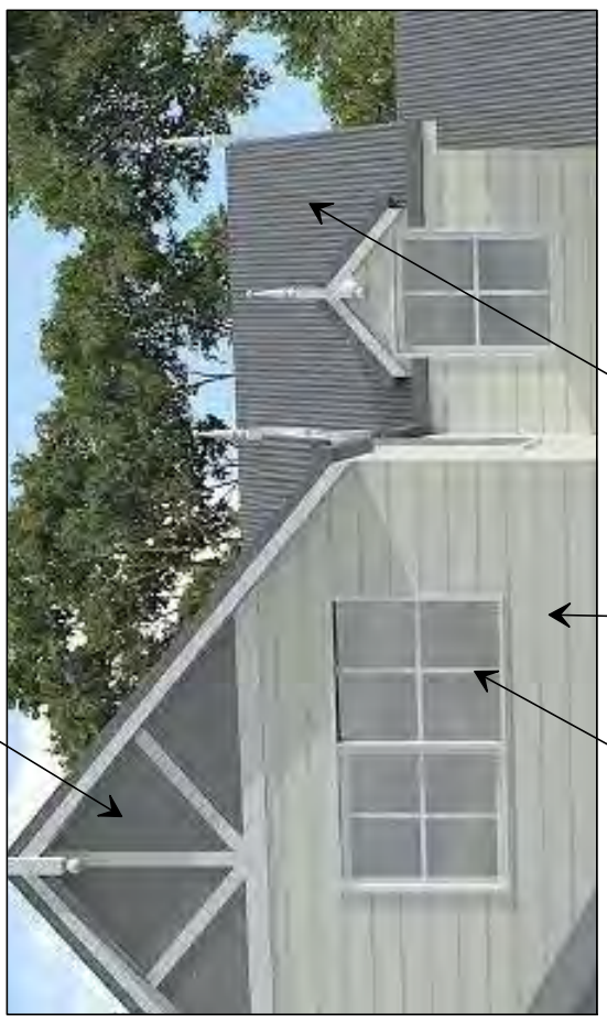
WHITE WINDOWS CEMENT SHEET - PAINTED MID-GREY WITH WHITE STRAPPING LIGHT - MID GREY COLOURBOND ROOF.
