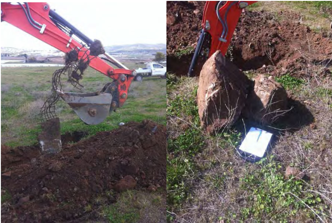
Figures 2 & 3: Wire and concrete (left) and oversize boulders (right) excavated from Pit 7.
