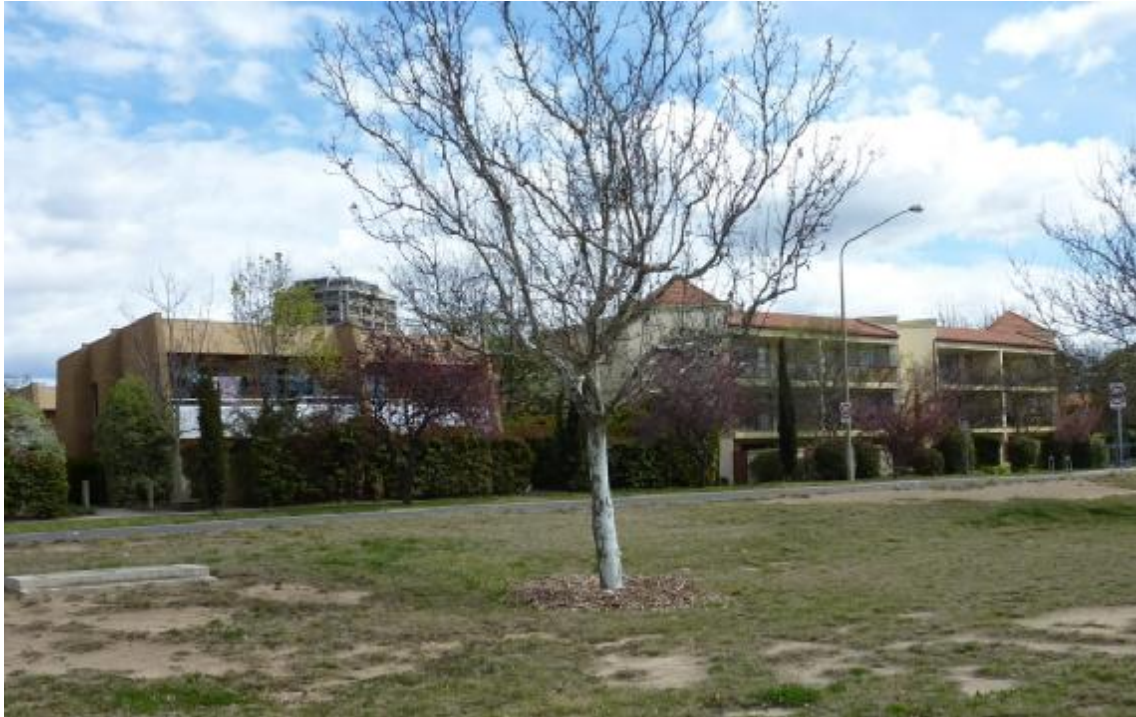
Figure 38 View of the west side of Wentworth Avenue from the median strip.
