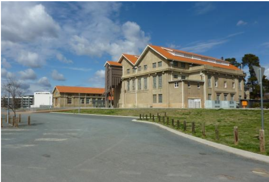
Figure 42 View of the Power House and Fitters' Workshop from the north-east.
