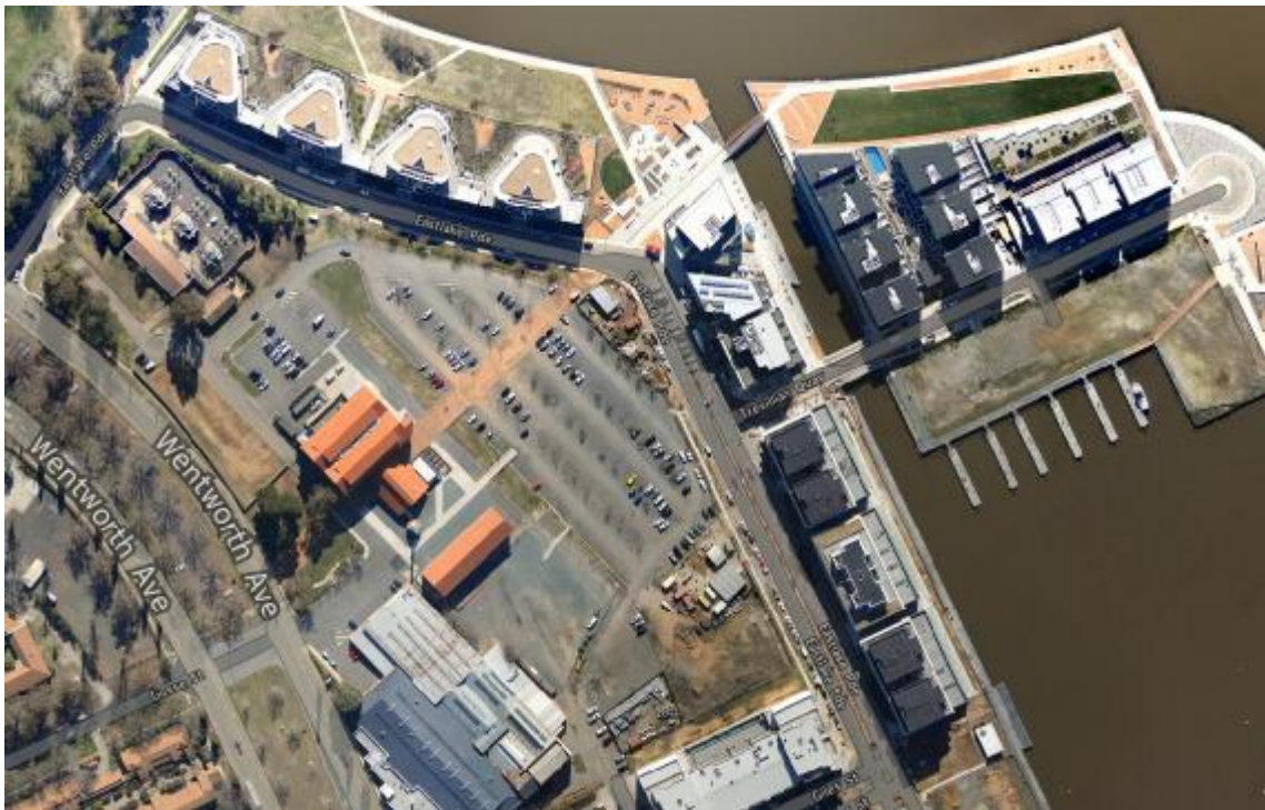
Figure 37 Aerial view of Kingston Section 49, July 2013. Source: www.nearmap.com
