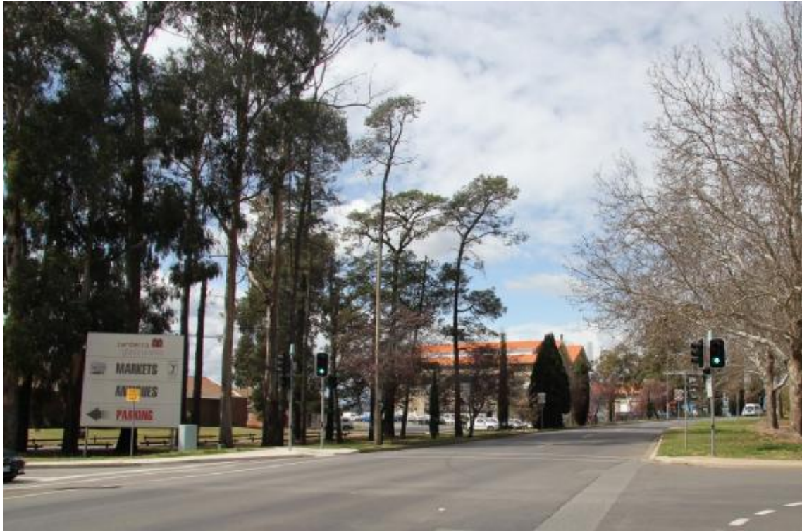
Figure 41 View of the Power House looking south along Wentworth Avenue.
