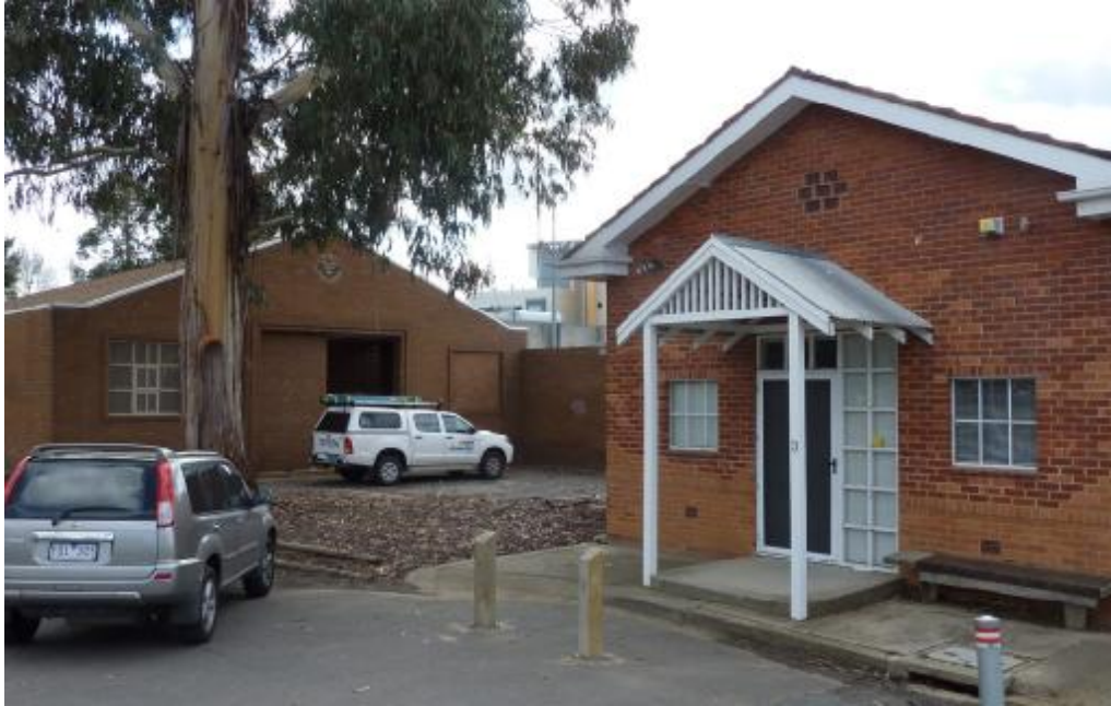
Figure 40 The non-original south-west elevation of the 1948 switch room, pictured right.
