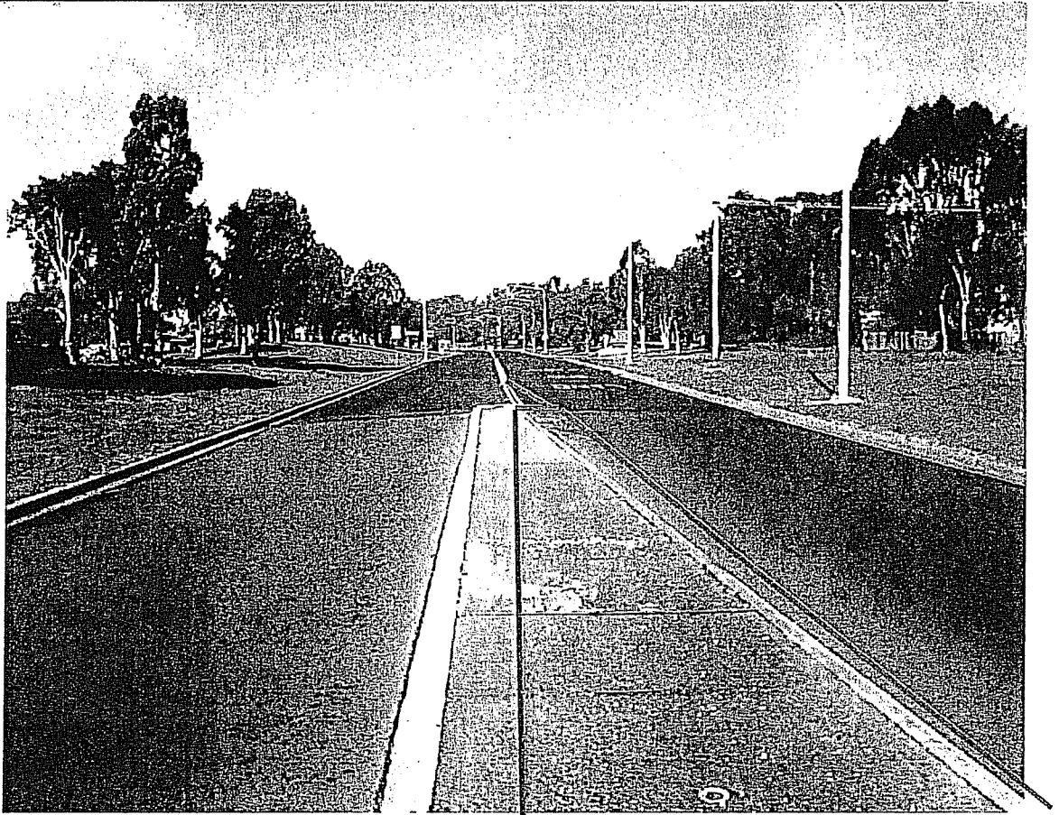
Figure 4 The median on the southern approach could be reconstructed to permit two southbound lanes
