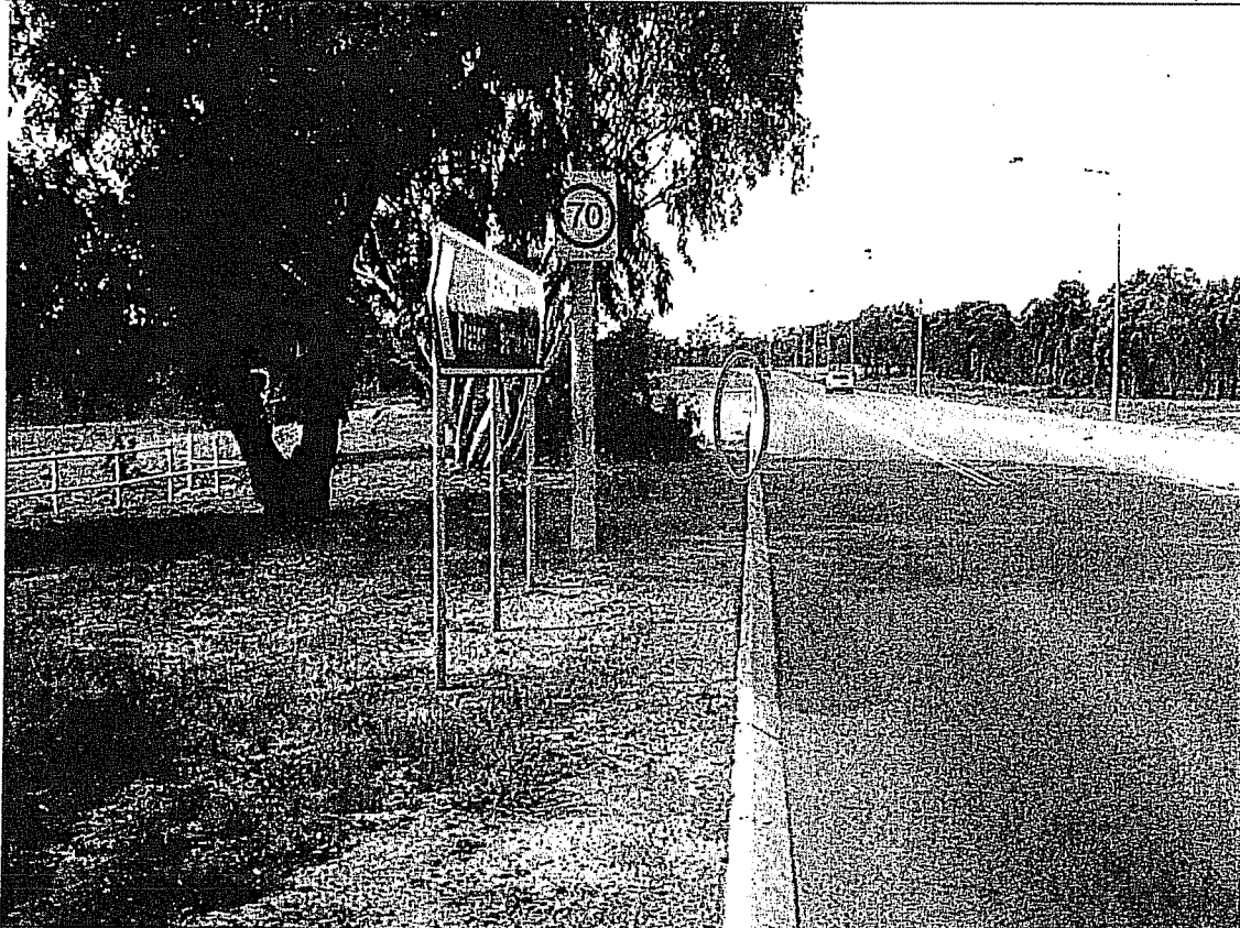
Figure 6 Lack of grass & loss of backfill behind Kuringa Drive eastbound kerb indicates possible use of verge by heavy vehicles
