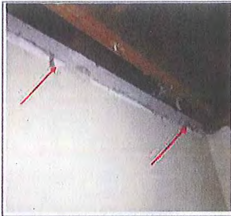
Photograph 9: Ceiling area with cornices removed
