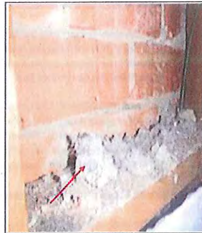
Photograph 2: West Gable end wall
