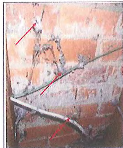
Photograph 8: East gable end on wiring
