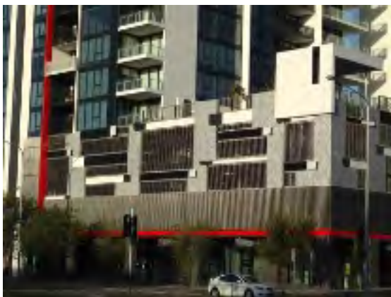
Picture 11: The Sentinel residential development with its car park occupying the lower floors
