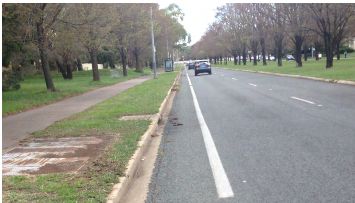
Narrow on-road cycle lane, Benjamin Way, looking south
