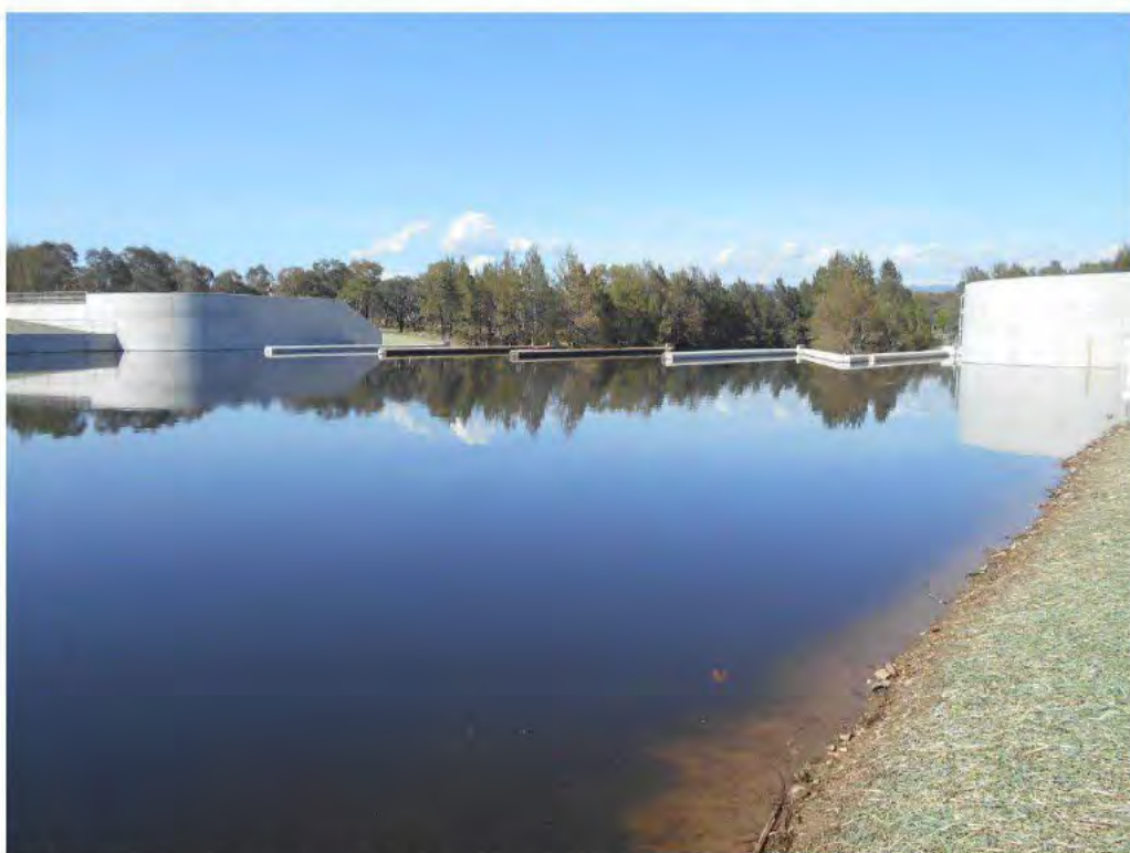
Photograph 2 – General view of the upstream pool and the weir.
