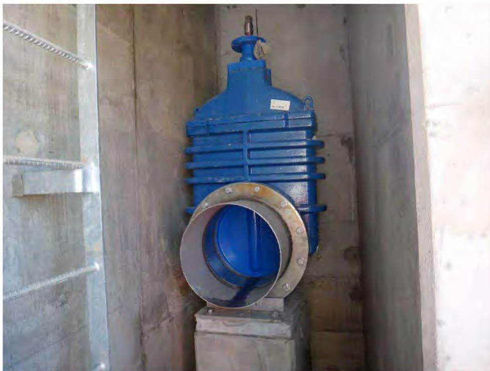
Photograph 41 - Overview of the gate valve located in the outlet valve chamber.
