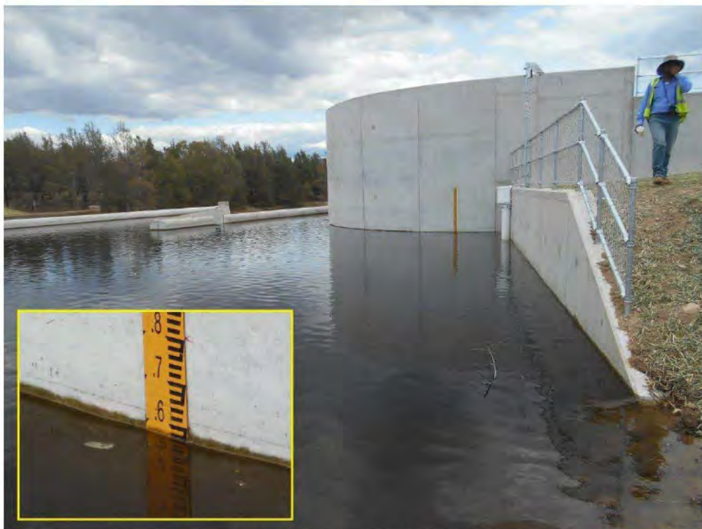
Photograph 7 – General view of RHS training wall and the gauge board.
