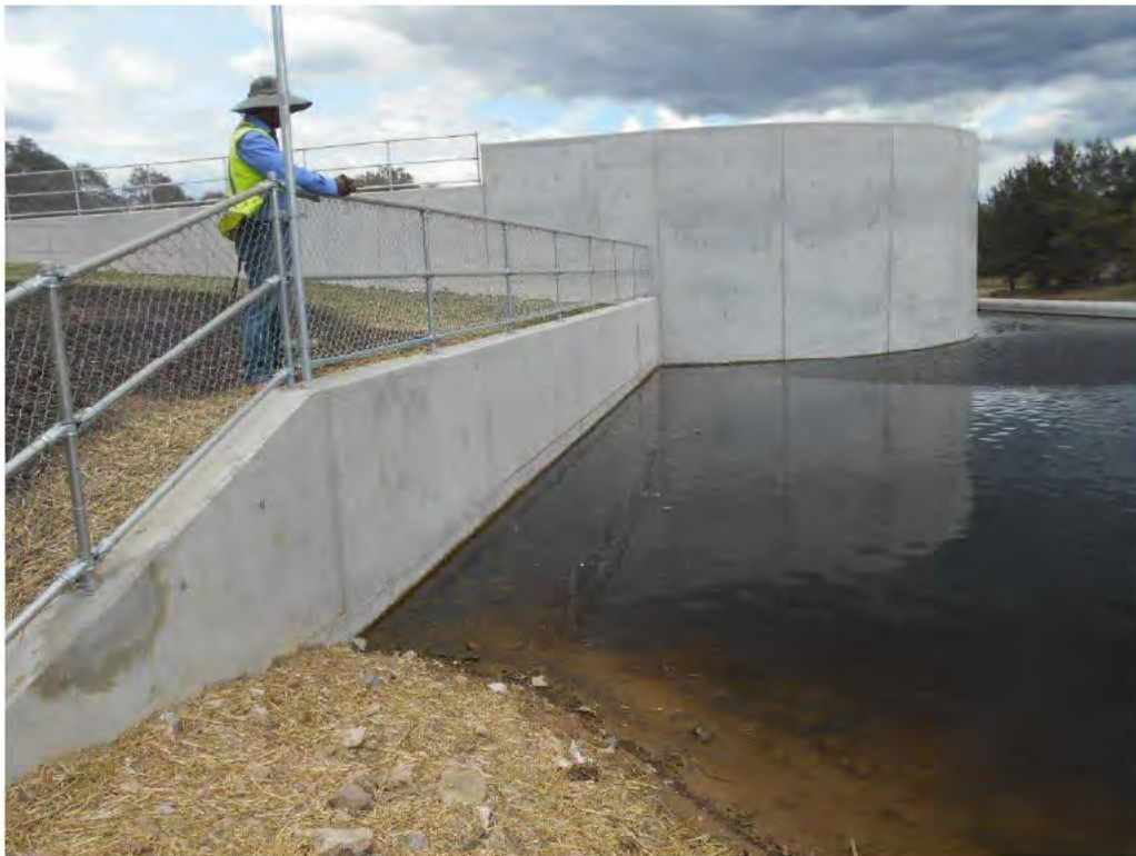
Photograph 34 – General view of the LHS training wall.
