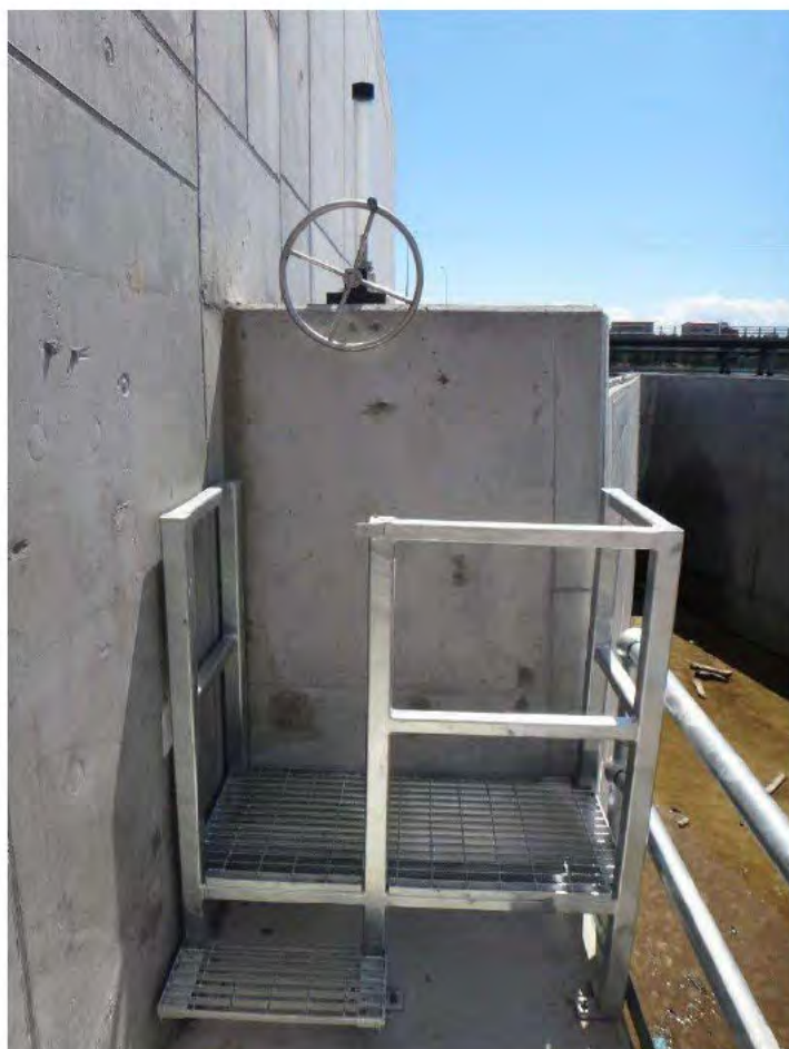
Photograph 41 - Overview of the gate valve located in the outlet valve chamber.
