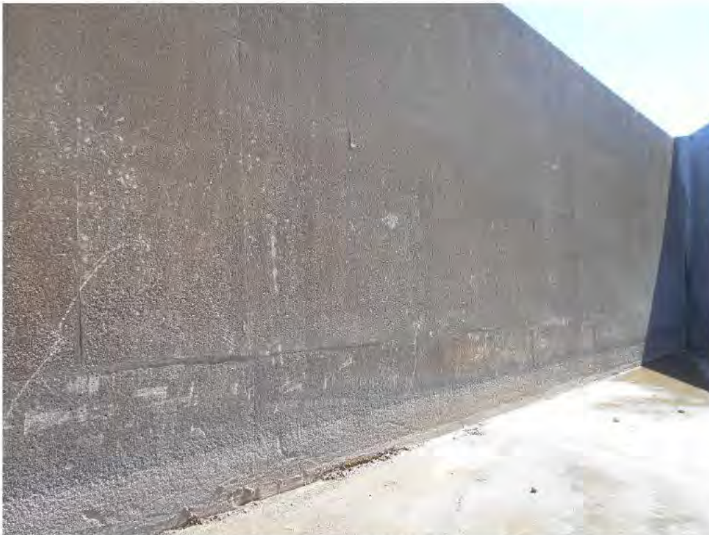
Photograph 24 – General view of the RHS wall of the Bay 2.
