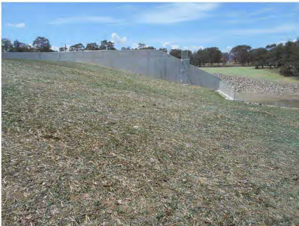
Photograph 9 – Downstream face of the RHS embankment.
