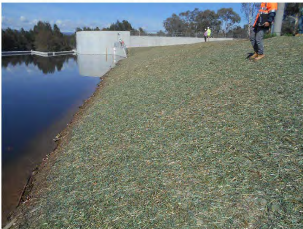
Photograph 6 – View of the RHS batter immediately upstream of the weir.
