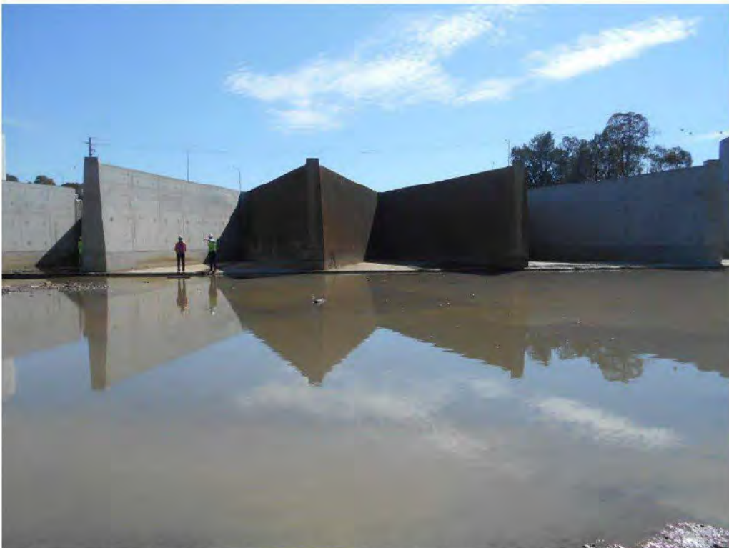
Photograph 4 – General downstream view of the weir and downstream pool.
