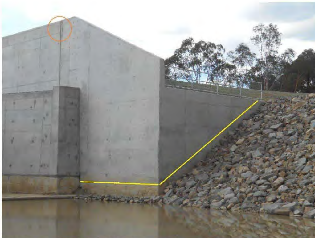
Photograph 31 – General view of the LHS wing wall.
