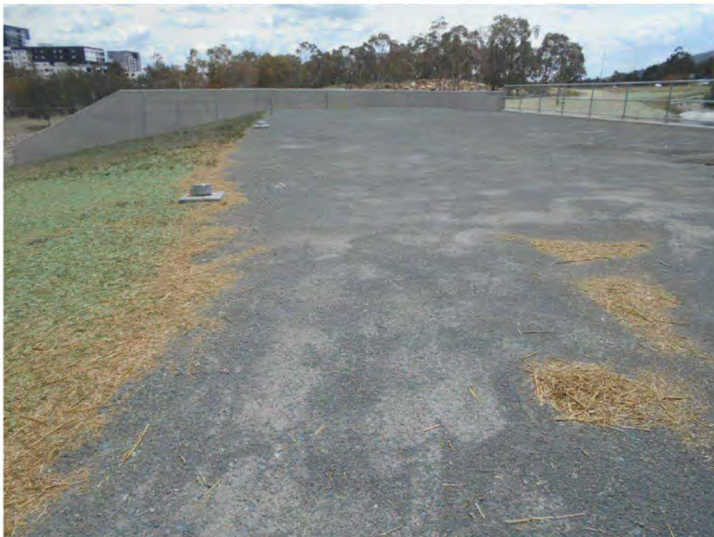
Photograph 35 – General view of the crest of the LHS embankment dam.
