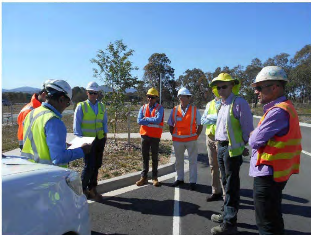
Photograph 1 – Job Safety Assessment (JSA) and briefing session undertaken prior to the commencement of the inspection.
