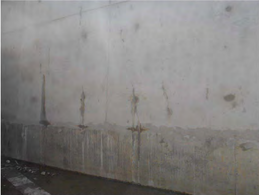
Photograph 27 – General view of the LHS wall of the Bay 2.
