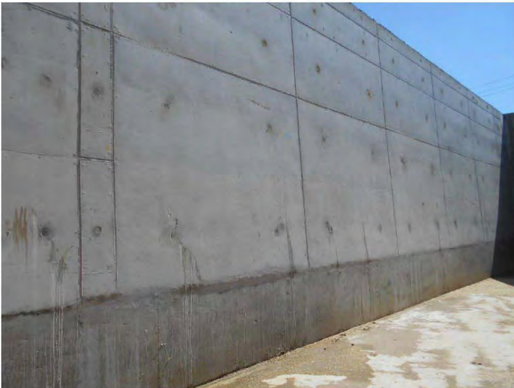
Photograph 28 – General view of the RHS wall of the Bay 1.
