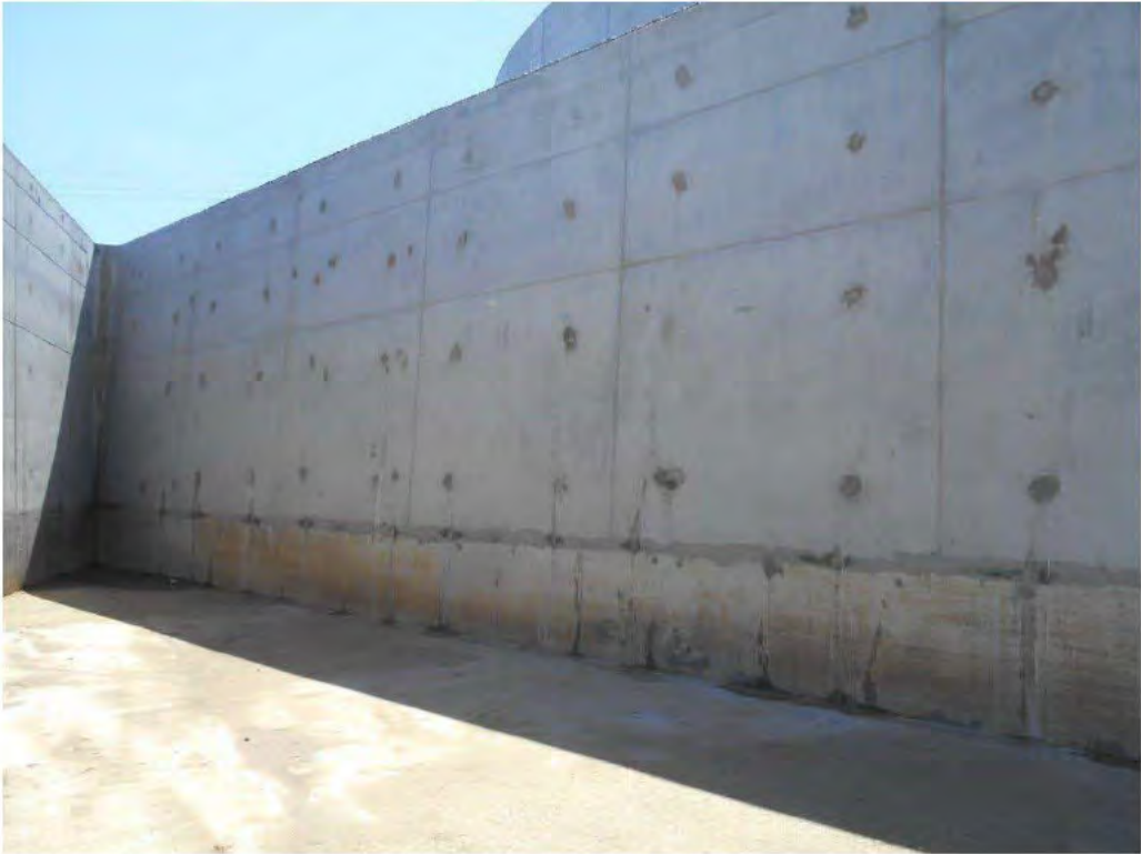
Photograph 30 – General view of the LHS wall of the Bay 1.
