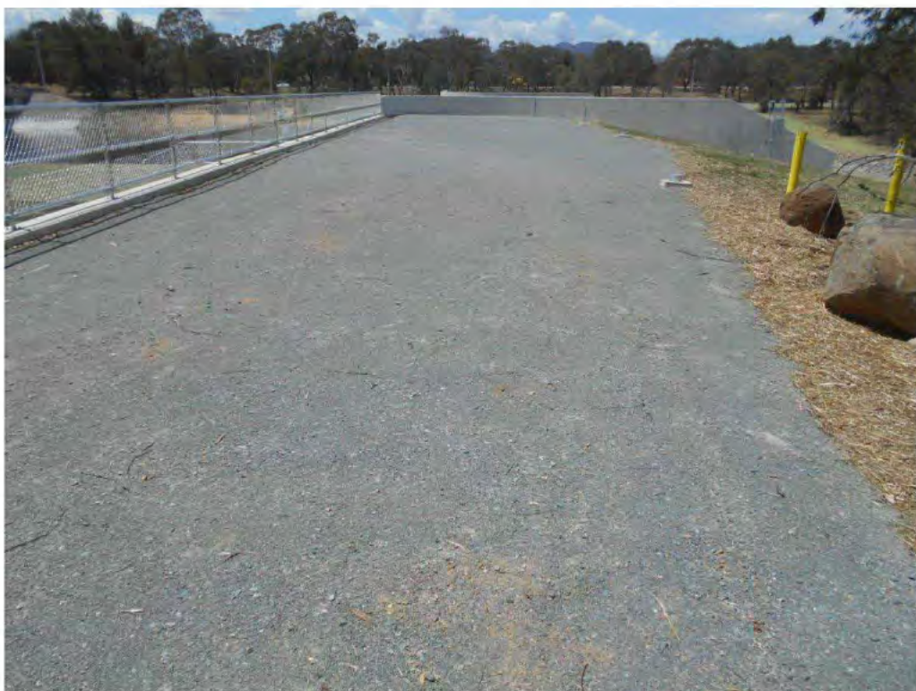
Photograph 8 – General view of the crest of the RHS embankment.
