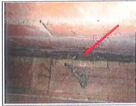
Photographs 7 and 8: Wall cavity and clump of asbestos insulation collected from cavity resting on stud wall timber base plate.
