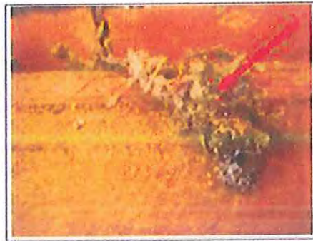
Photographs 7 and 8: Wall cavity and clump of asbestos insulation collected from cavity resting on stud wall timber base plate.
