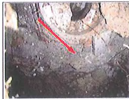
Photographs 11 and 12: Clumps of loose asbestos resting on the floor of the sub-floor space adjacent sewer and in the perimeter wall cavity.
