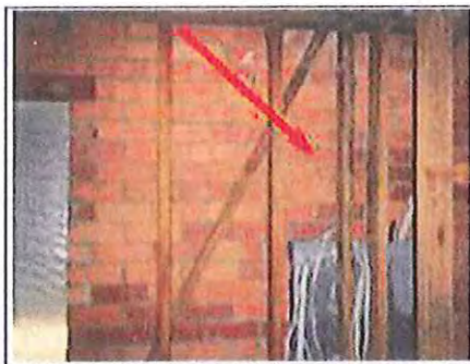
Photographs 5 and 6: Southern side brick wall, surface dust to smooth bricks adjacent electrical switchboard recess. Surface dust sample location – sample J0711
