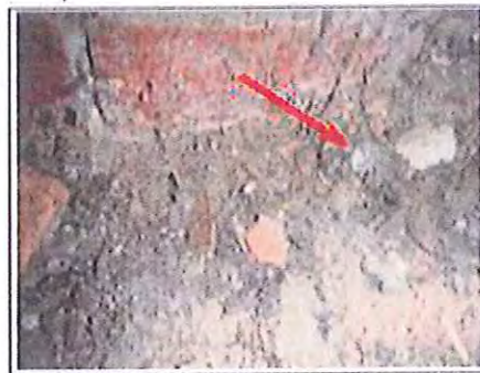
Photographs 9 and 10: Clumps of loose asbestos resting on the floor of the sub-floor space and in the perimeter wall cavity.
