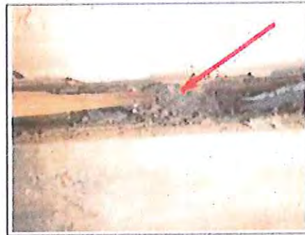
Photographs 9 and 10: Clumps of loose asbestos resting on the floor of the sub-floor space and in the perimeter wall cavity.
