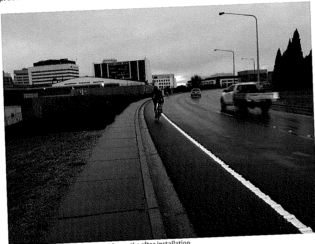
Figure 14. Screed applied ATLM – 12 months after installation
