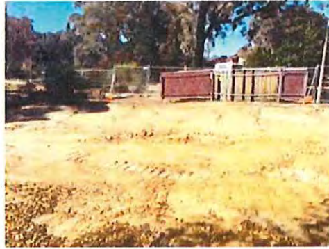
Cleared area of the demolition zone
