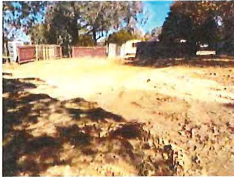
Cleared area of the demolition zone
