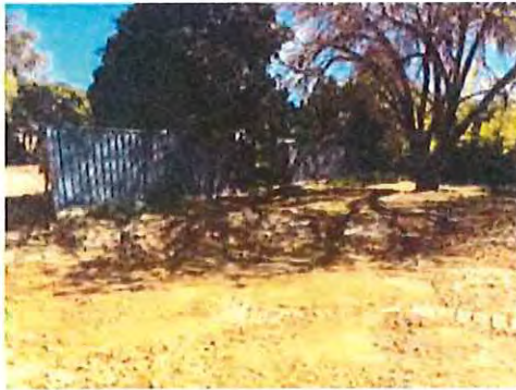
Cleared area of the demolition zone
