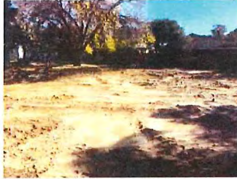
Cleared area of the demolition zone
