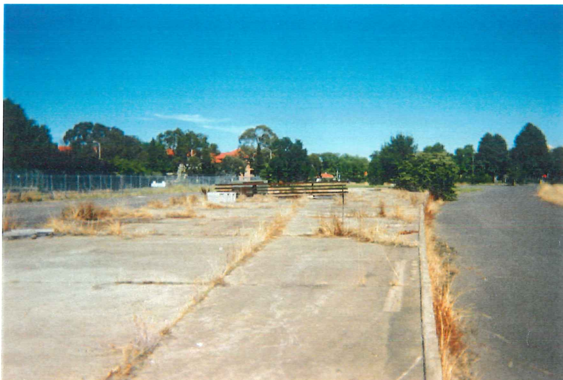
Photo 1: No evidence of asbestos sheeting on surface soils or slabs.
