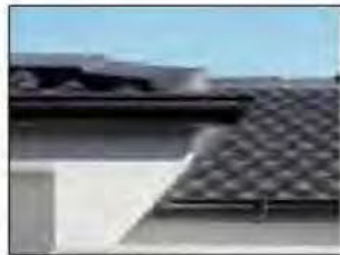
RF2 PAINT EXISTING ROOF - MONUMENT
