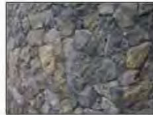
SW1 STONE WALL DRY STACK - BLUE STONE
