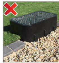
Incorrect box level
