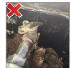
No clearance for Ball valve
