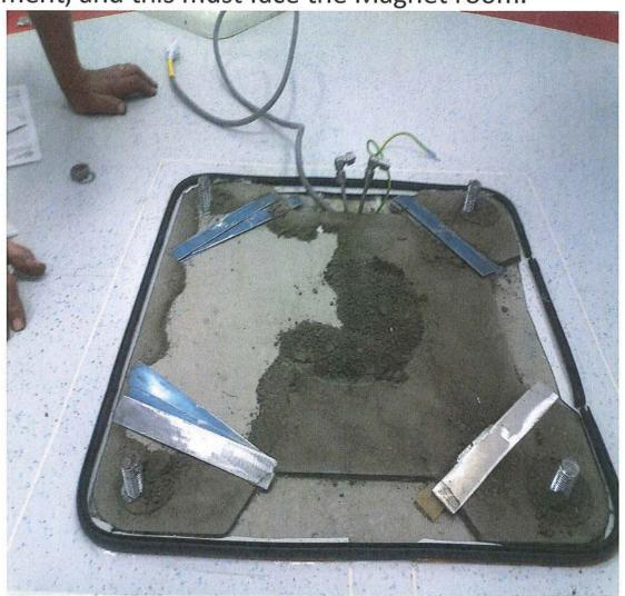
Do not move the packing strips, fit plastic tubes over studs to reduce chance of damage by bed base.
