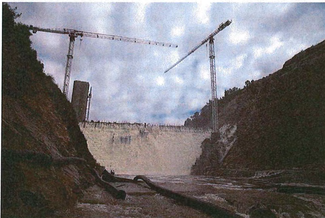
Figure 6 - View of Dam from downstream - 6 March 2102
