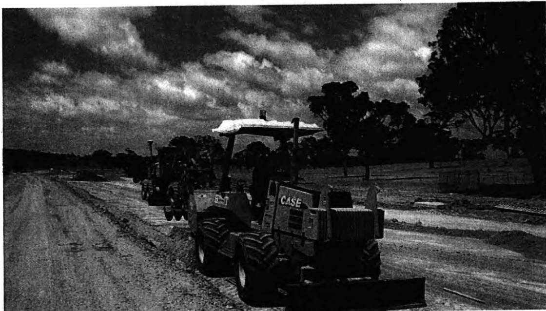
Image 02: Trenching for subsoils east of Road 04 Intersection
