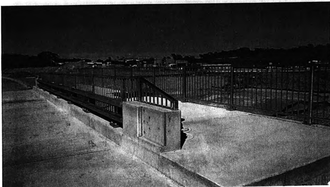
Image 02: Guardrail and handrail installation on bridge
