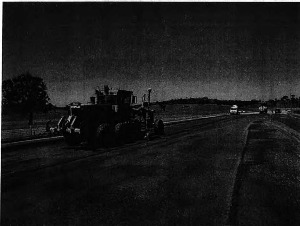
Image 02: Placement of sub-base material and preparation of kerb foundations
