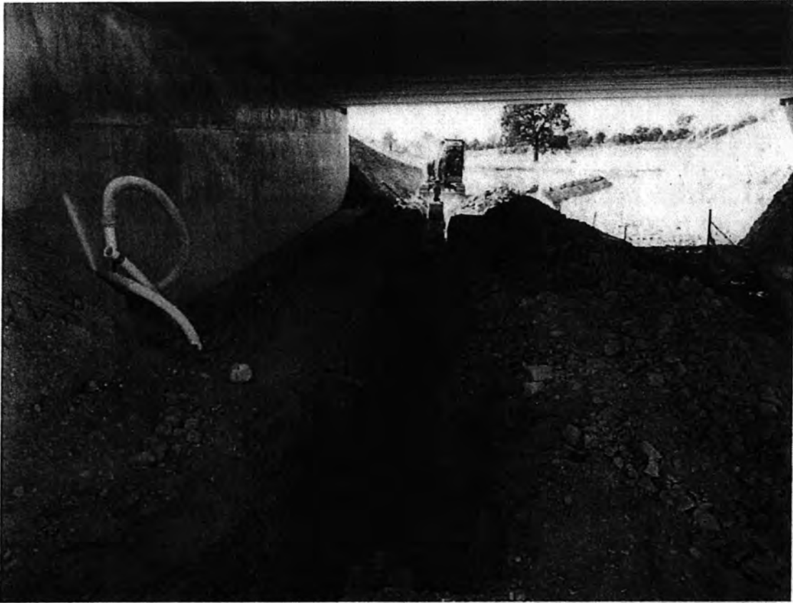
Excavation for storm water line B
