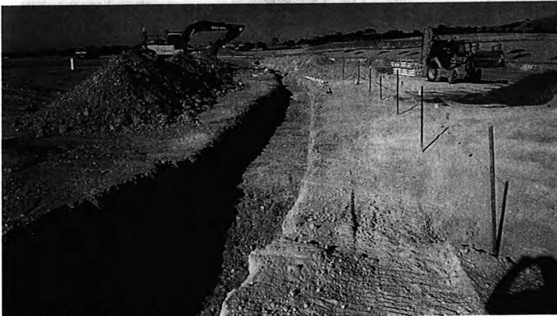
Image 01: Shared trench construction at CH 900
