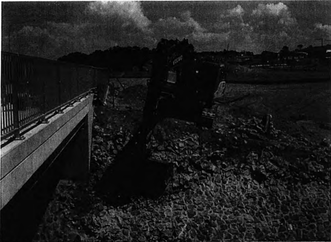
Removing stone pitching at the south west batter of the bridge
