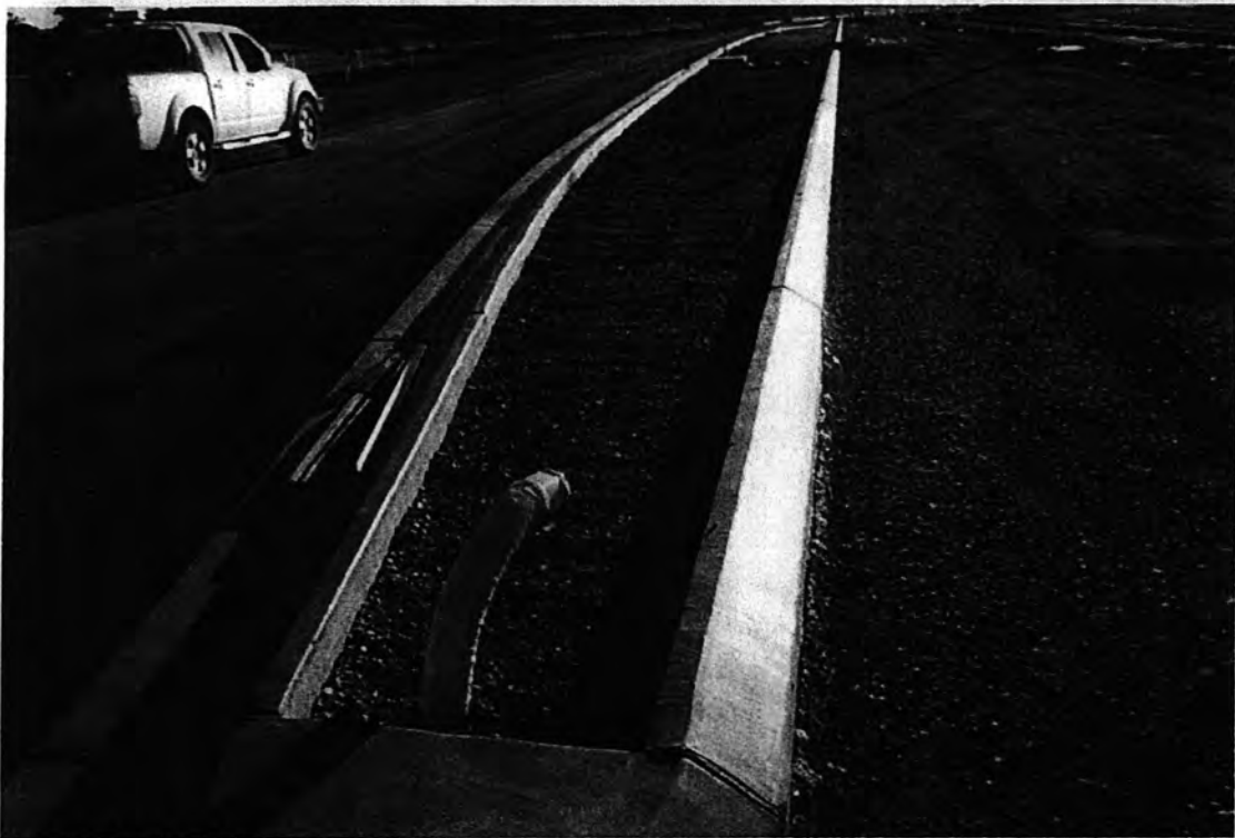
Kerb and gutter, traffic island - CH1200
