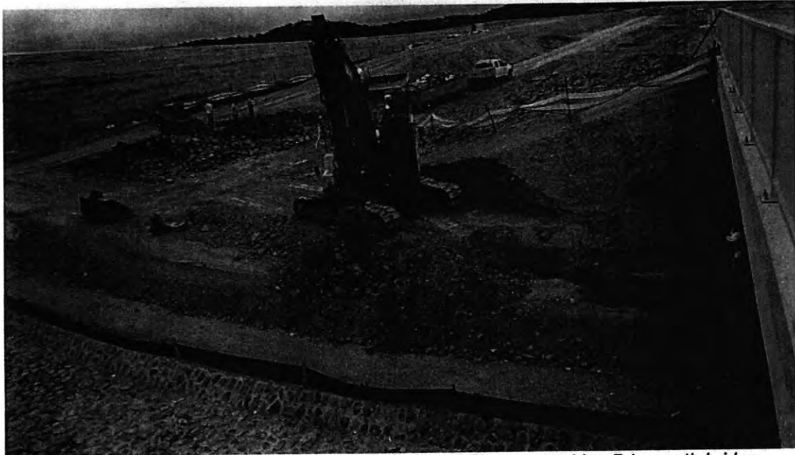
Image 01: Excavations commenced for installation of Stormwater Line B beneath bridge.
