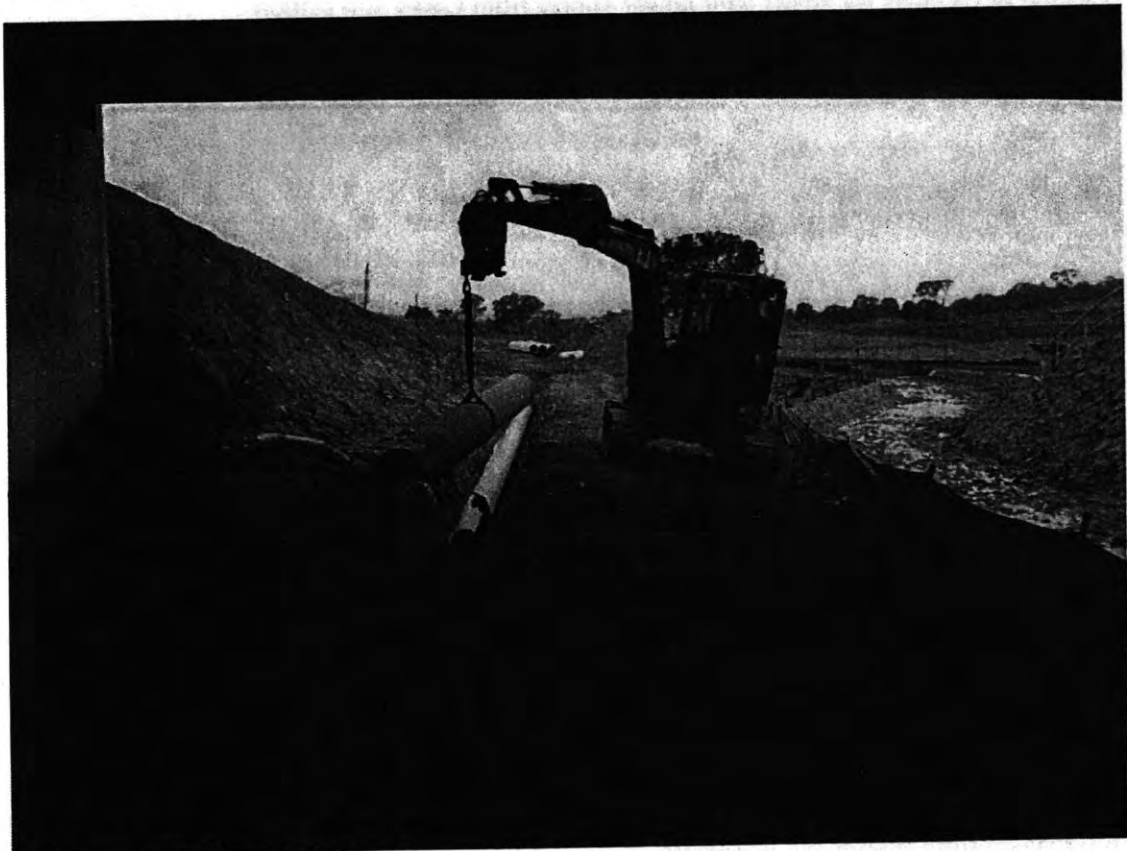
Laying pipe in storm water line B
