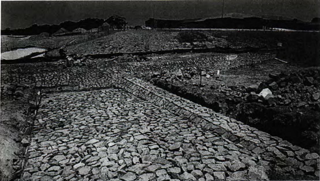
Image 03: Stone pitching at western side of bridge
