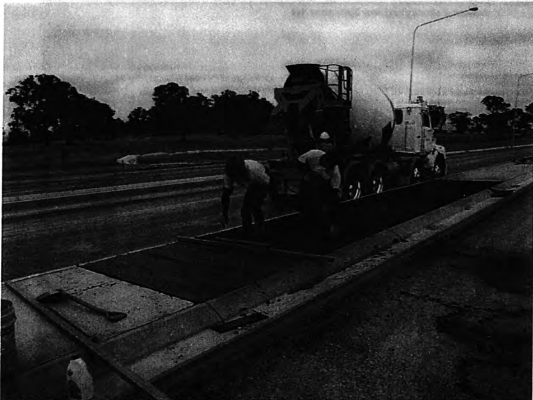
Image 04: Placement of concrete for islands west of Mirabei Dr.
