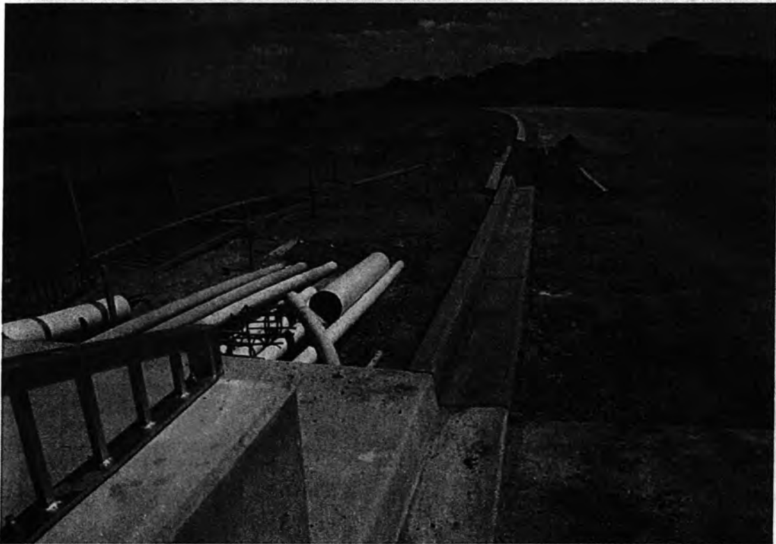
Kerb transition from bridge SFK at CH410
