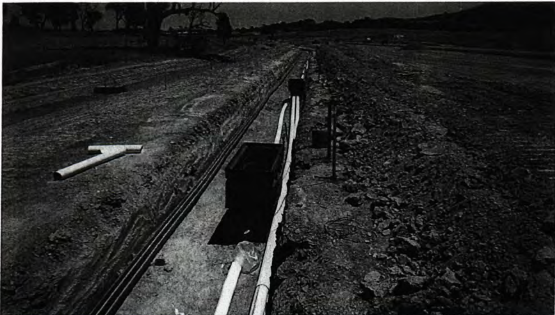
Image 04: Gas pipe and NBN conduits, CH 1200
