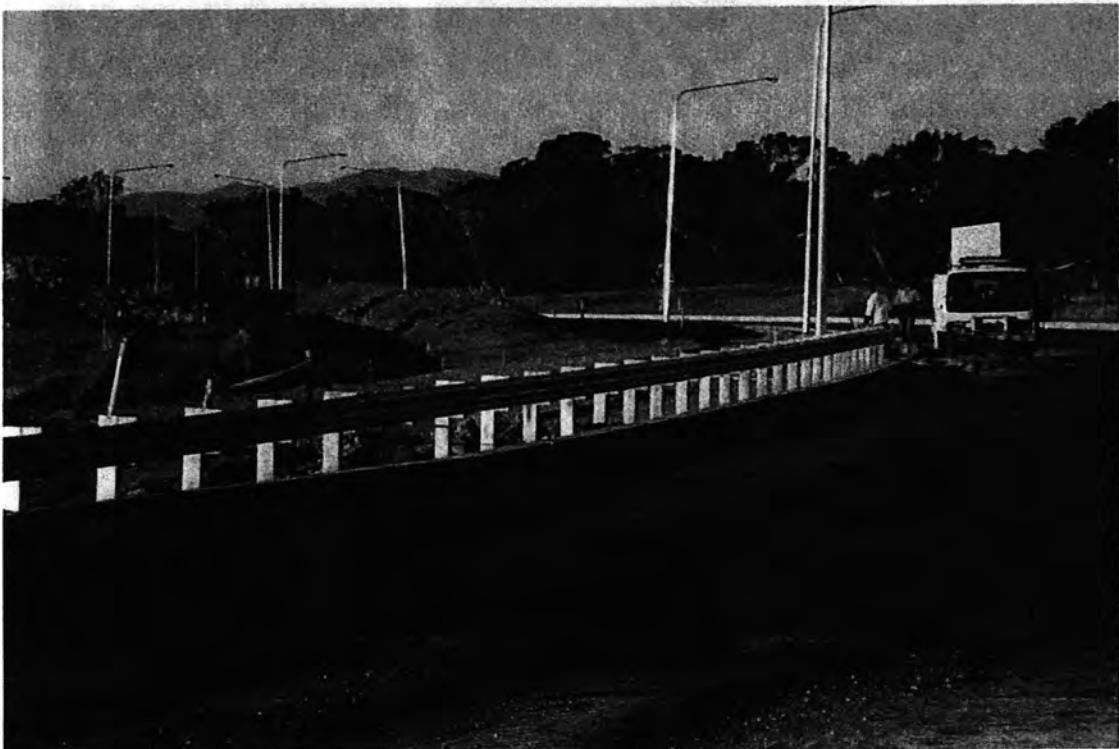
W-Beam guardrail installation at southern approach to the bridge
