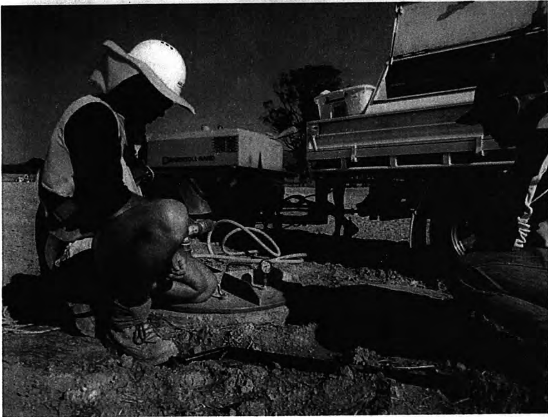
Sewer manhole vacuum test at S19
