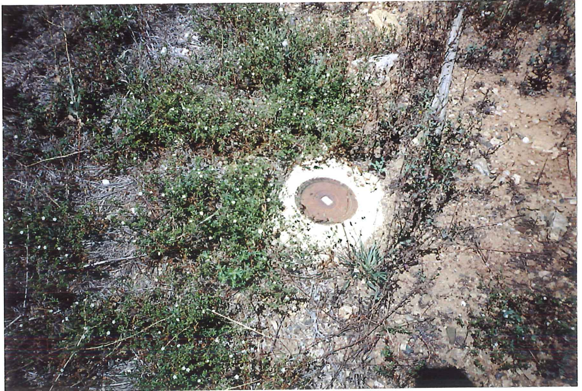
Photo 5: Groundwater well Opposite Mobil Depot
