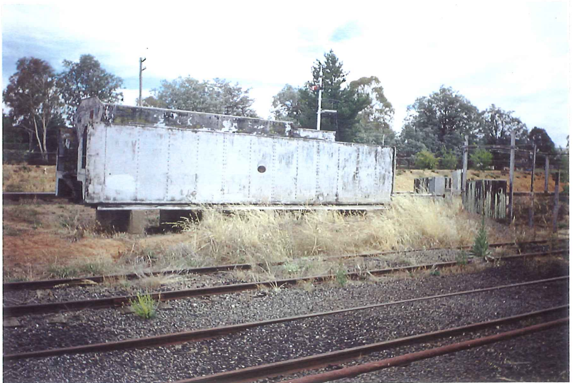
Photo 6: Old Fuel Storage Tank in Canberra Yard
