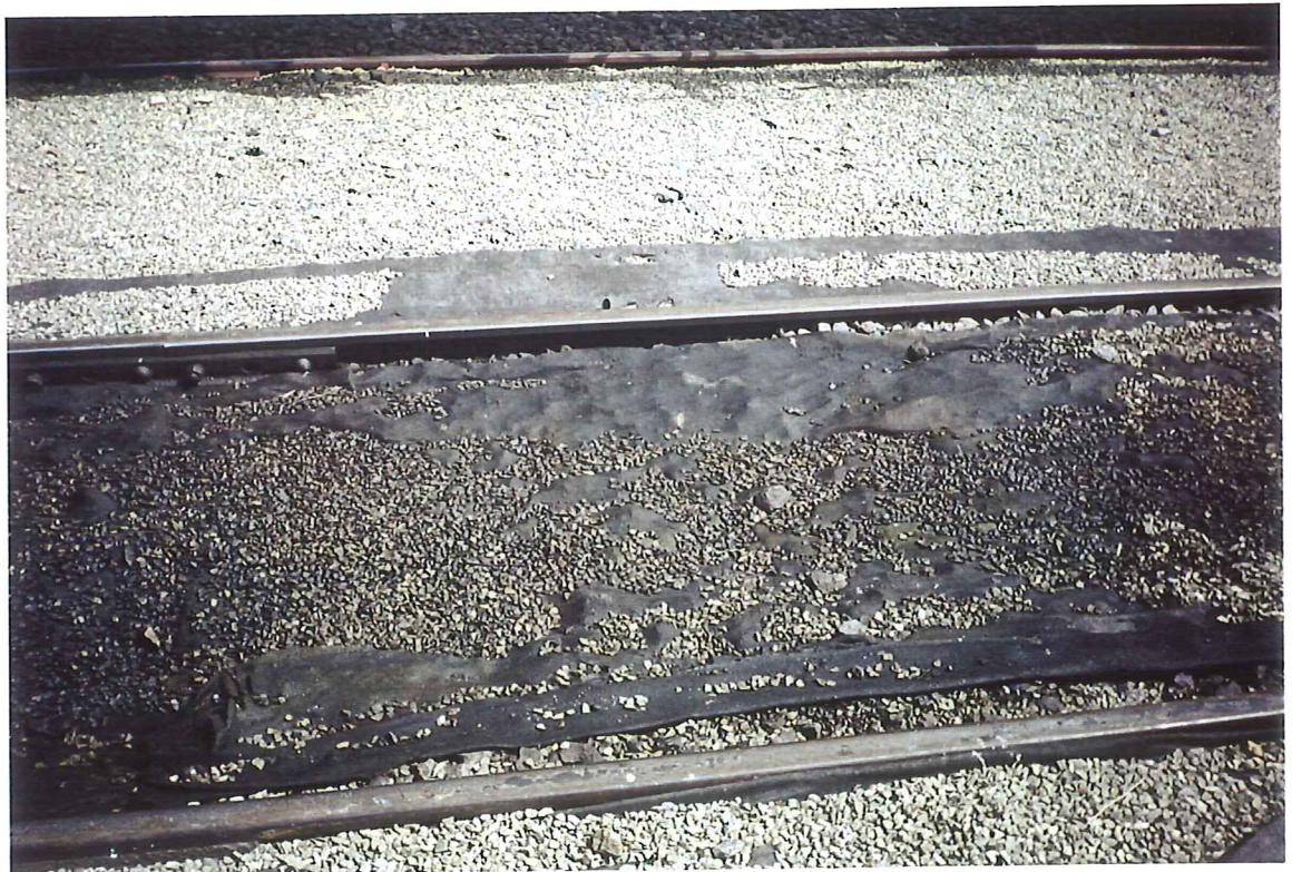
Photo 24: Membrane Layer Underlying Ballast
