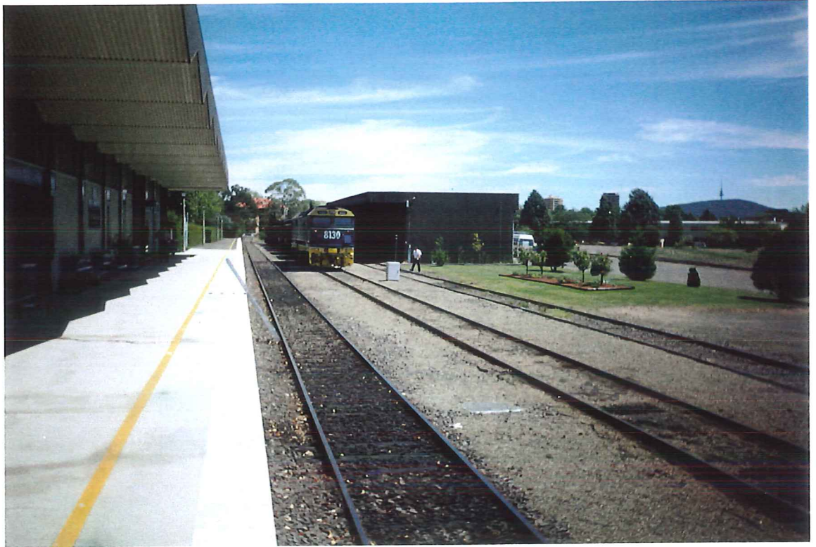
Photo 23: Hydrocarbon Staining Next to Platform
