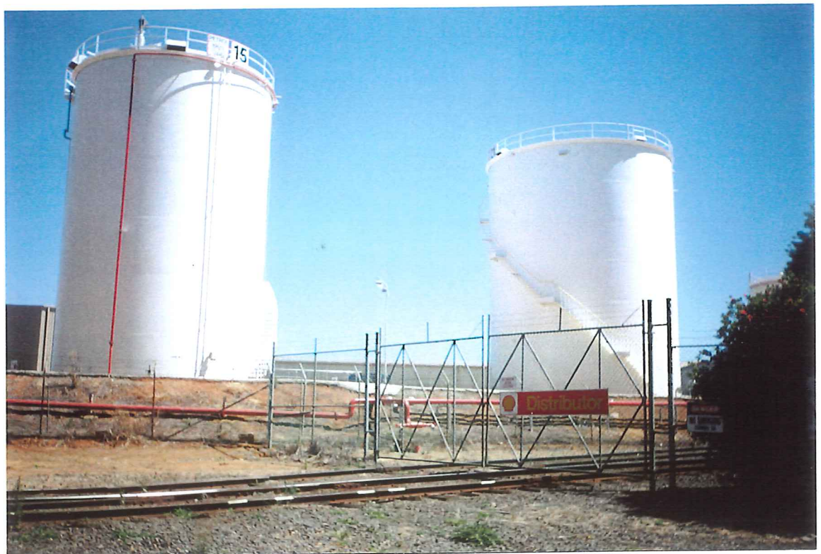
Photo 4: Shell Depot South of Main Line
