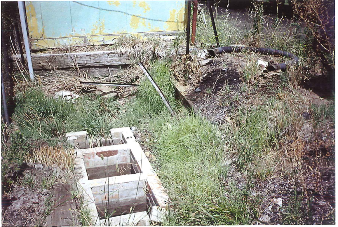
Photo 11: Stormwater Drain in ARHS Area
