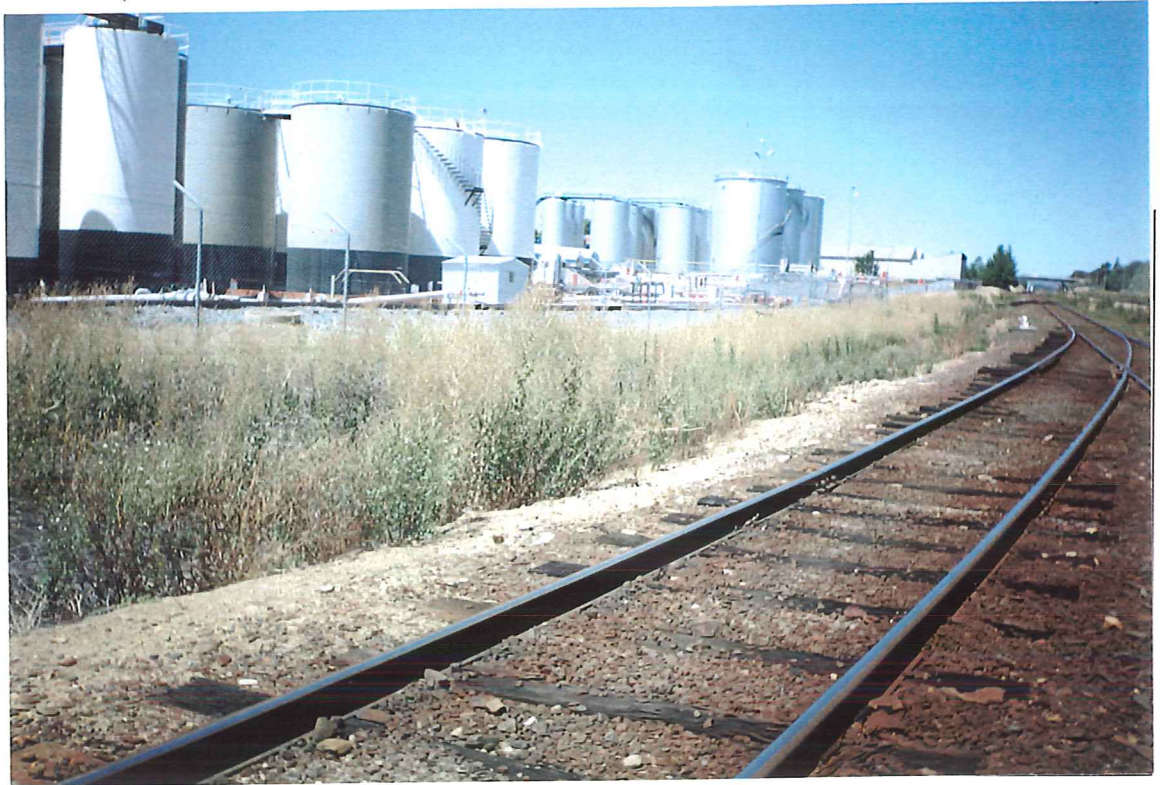
Photo 1: Fuel Depots North of Main Railway Line
