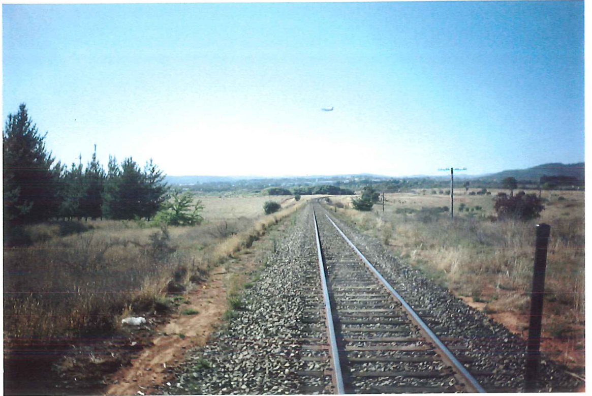
Photo 25: Rail Corridor East of Fyshwick
