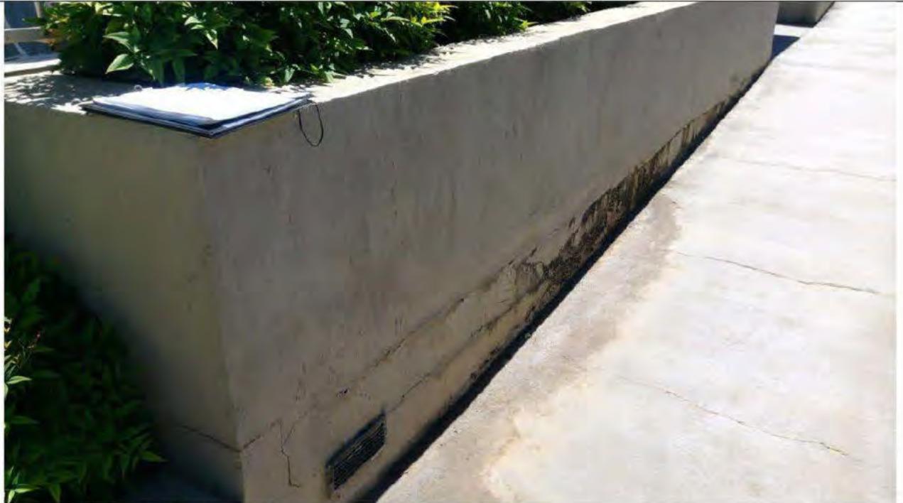
Typical render repair required after planter box repaired
