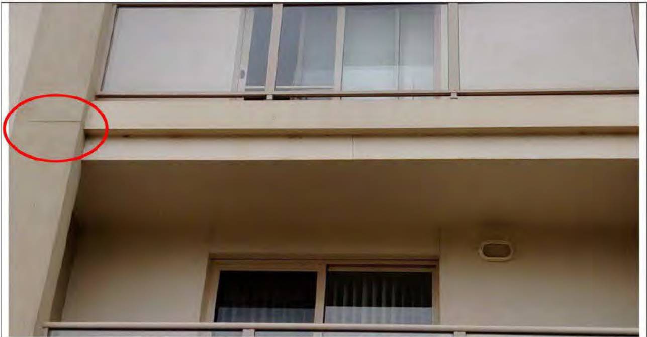
1- Typical minor articulation joint issue
