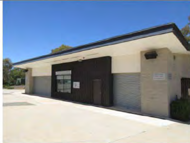
General view of East Ticketing Office.
