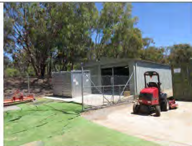
Main Maintenance Shed.
