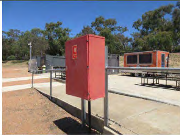
Hardstand and Fire Hose Reel Cabinet to 'Slab' Area.
