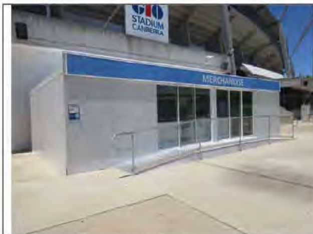
West Merchandise Structure.
