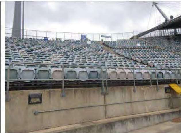
General view of South Terrace
