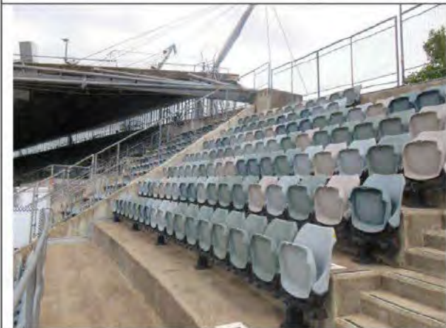
General view of North Terrace
