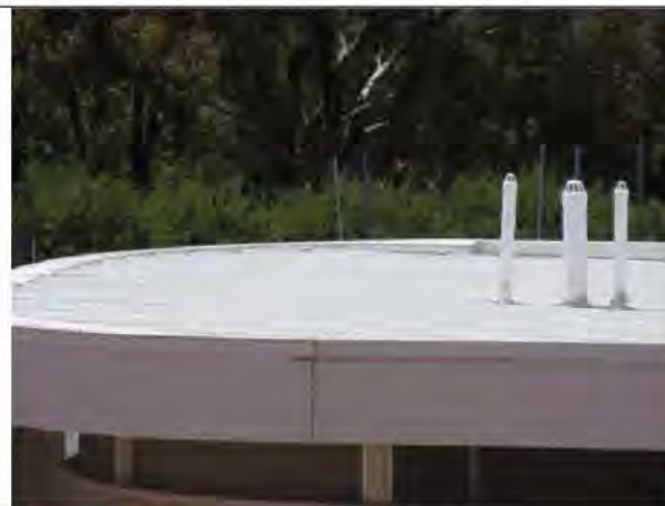
Typical fibre-cement cladding and sheet metal roofing to Toilet Blocks.
