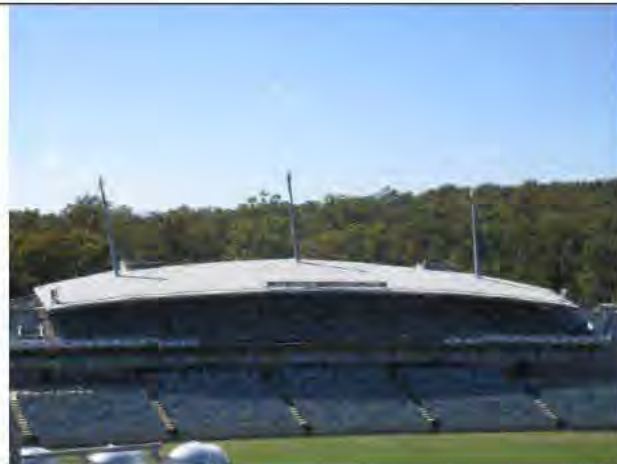
General view of East Gregan-Larkham Stand.
