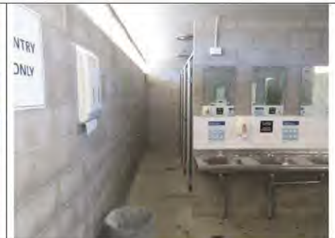
Typical Interior view of Female WC's
