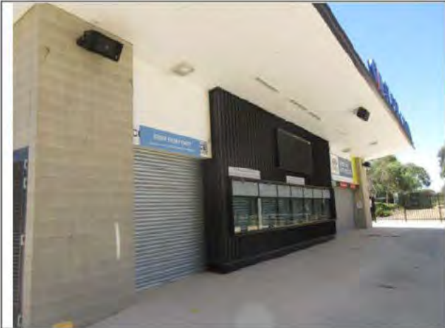
General view of West Ticketing Office.
