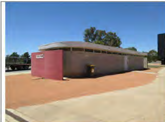
General Photo of North-West Toilet Block
