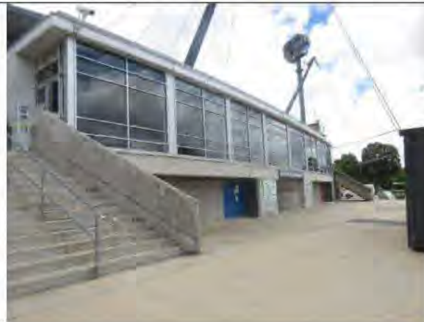
General view of east elevation to East Stand.
