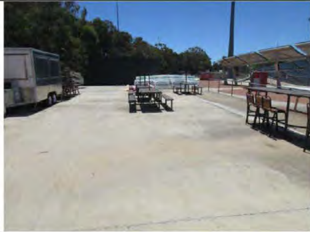
Hardstand to 'Slab' Area.
