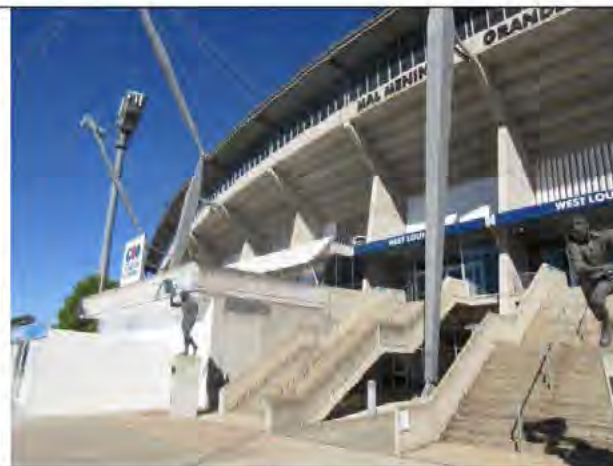
General view of west elevation to West Stand.
