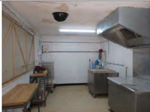
Interior of Slab Box.
