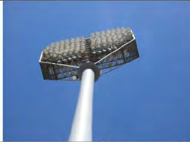
Typical light tower.
