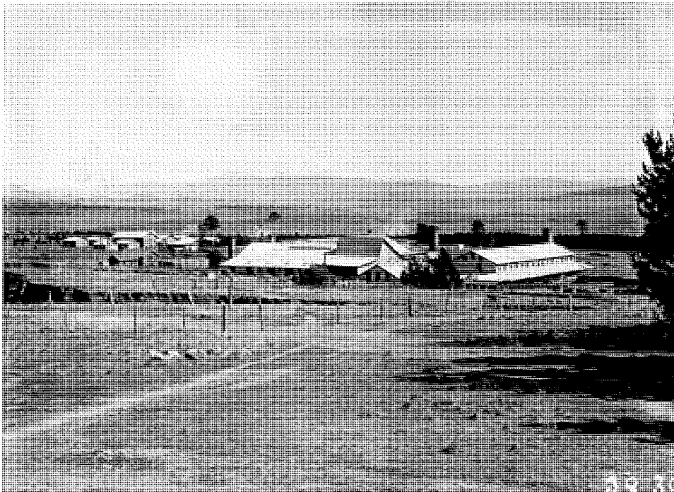
Figure 196 View west of the complex in 1929, including part of the quarry, the kilns and their stacks (albeit the Staffordshire kiln obscured), and the office and Power House (on left). The original crushing and pressing buildings (now demolished) are in the centre of this view, to the left of the Hardy patent kiln and in the background (far left) is the Brickworks Camp complex, now demolished. Source: National Library of Australia.
