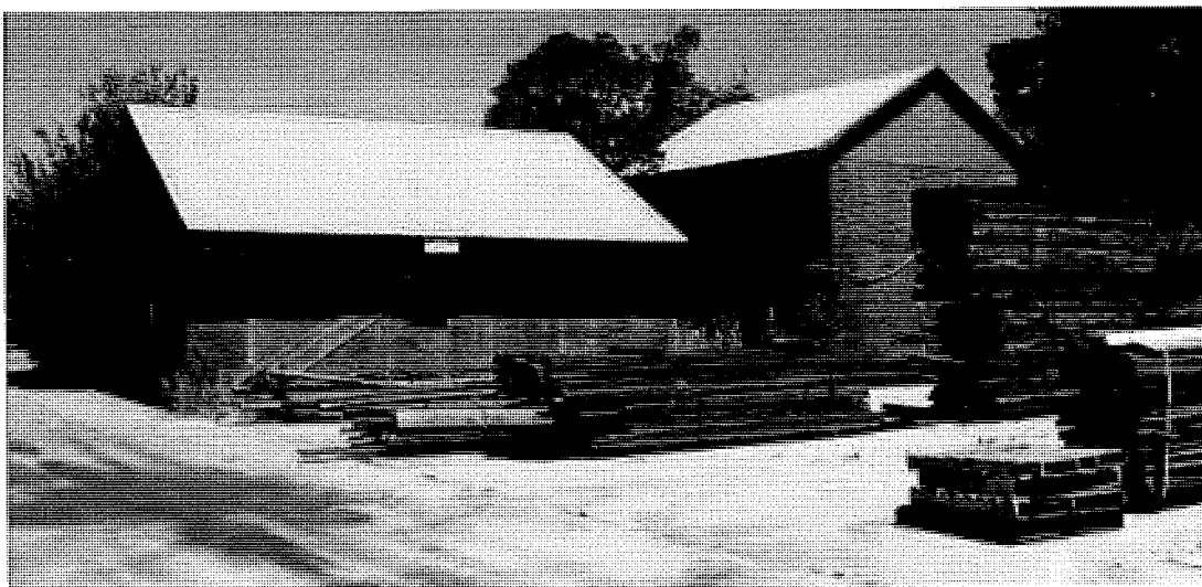
Figure 147 The former boiler house and adjoining substation/control room, viewed from the site of the former extrusion plant. The boiler house is at right.
