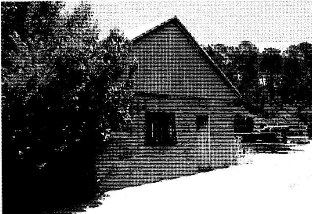
Figure 144 Substation/control room building, showing north elevation.
