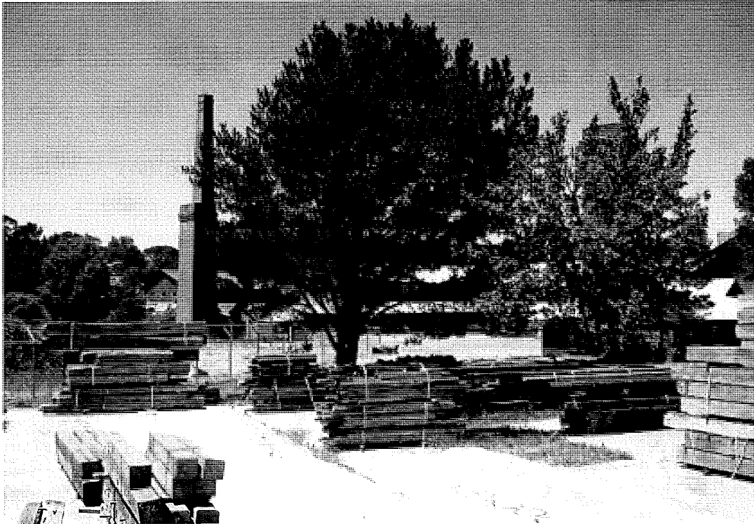
Figure 150 Brick extrusion plant site, looking north-east.
