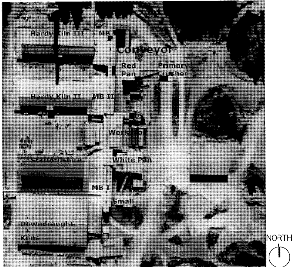
Figure 131 1976 aerial photograph with major site elements in the vicinity of the machine bays labelled. The Conveyor is indicated by a larger font. Source: ACT Heritage Library, Woden ACT.
