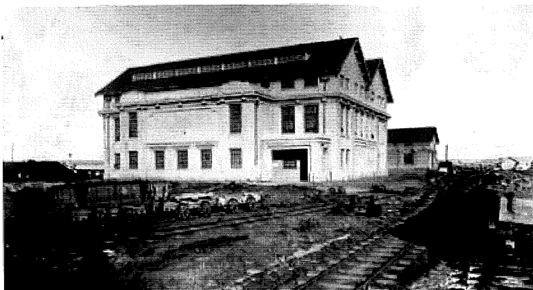
Figure 186 Kingston Power House, with brickworks railway in foreground. Source: NAA.
