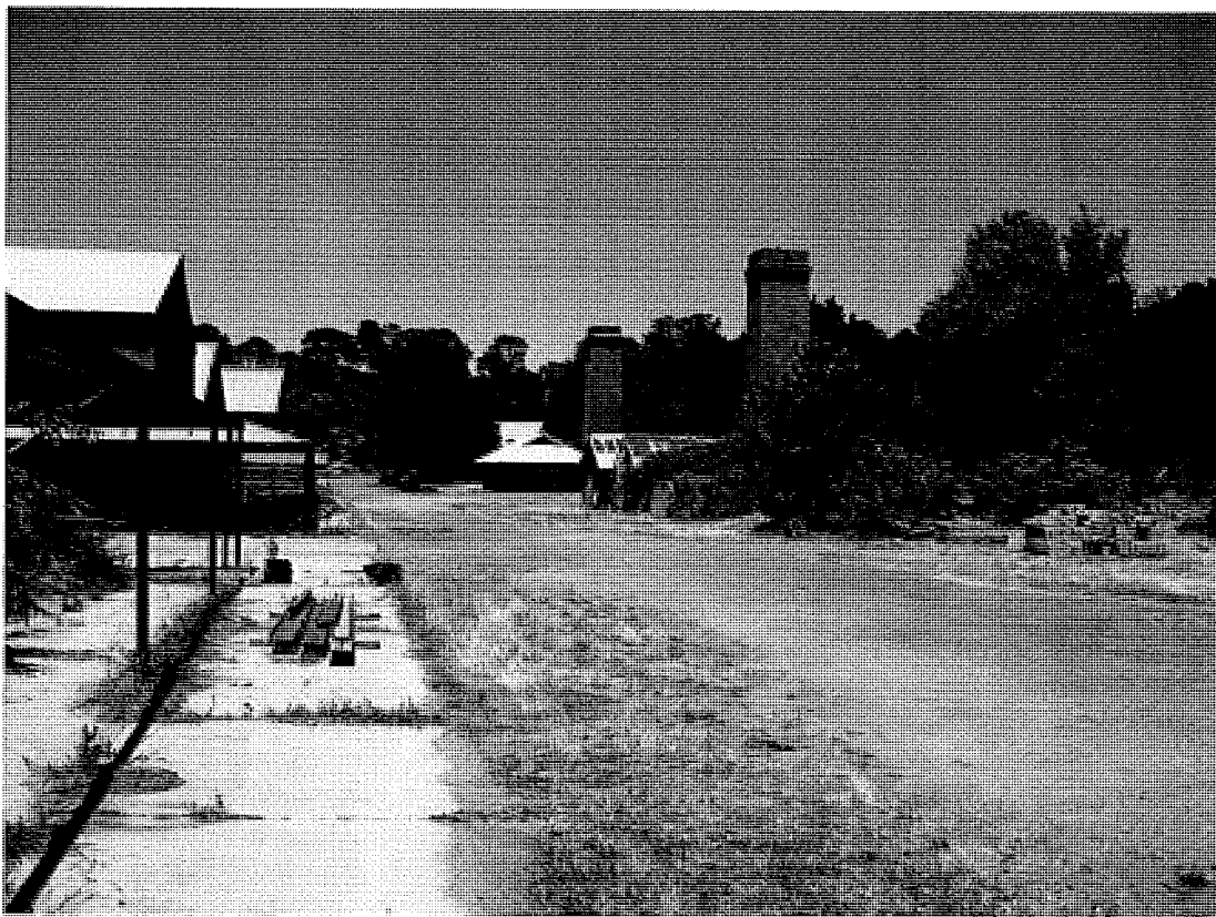
Figure 203 View southward between the kilns and their associated fan houses.
