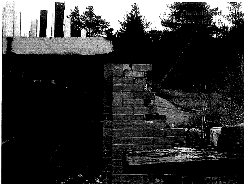
View on Brick Pier
