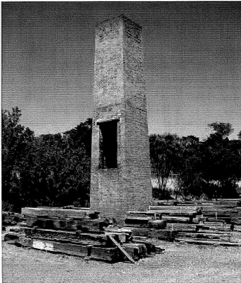
Figure 141 Chimney stack viewed from the north-west.
