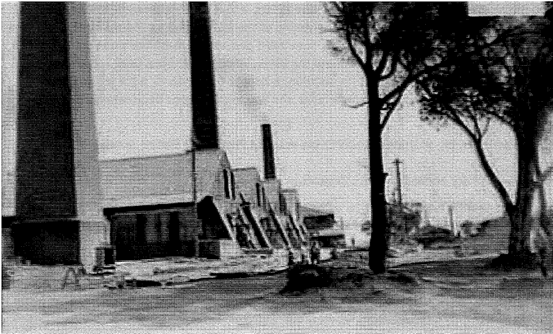
Figure 169 Continuous kilns at State Brickworks, pictured 1957. Source: NSW Heritage Register.
