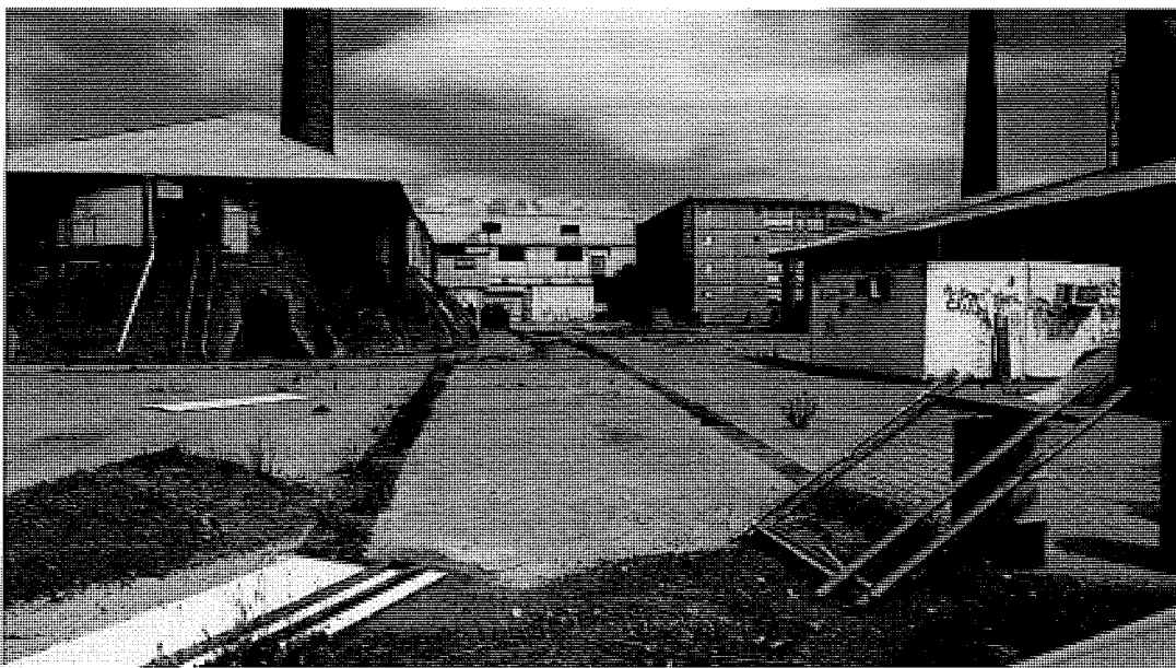
Figure 179 Former Hoffman works at Brunswick, pictured January 2010. Source: Lovell Chen.
