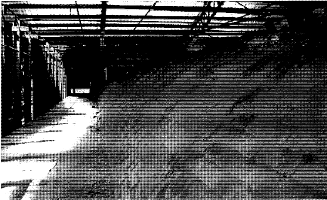
Figure 136 Kiln roof with brick walkway to sides.
