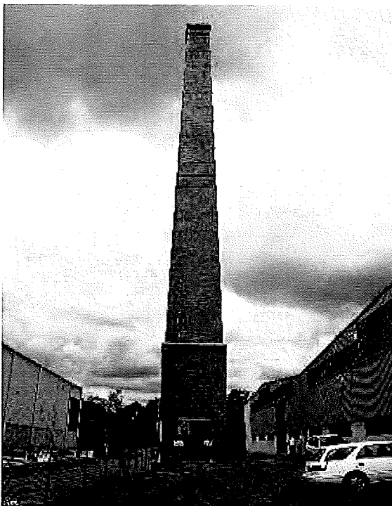
Figure 174 Hoffman stack at the former Newmarket Brickworks. Source: Queensland Heritage Register.
