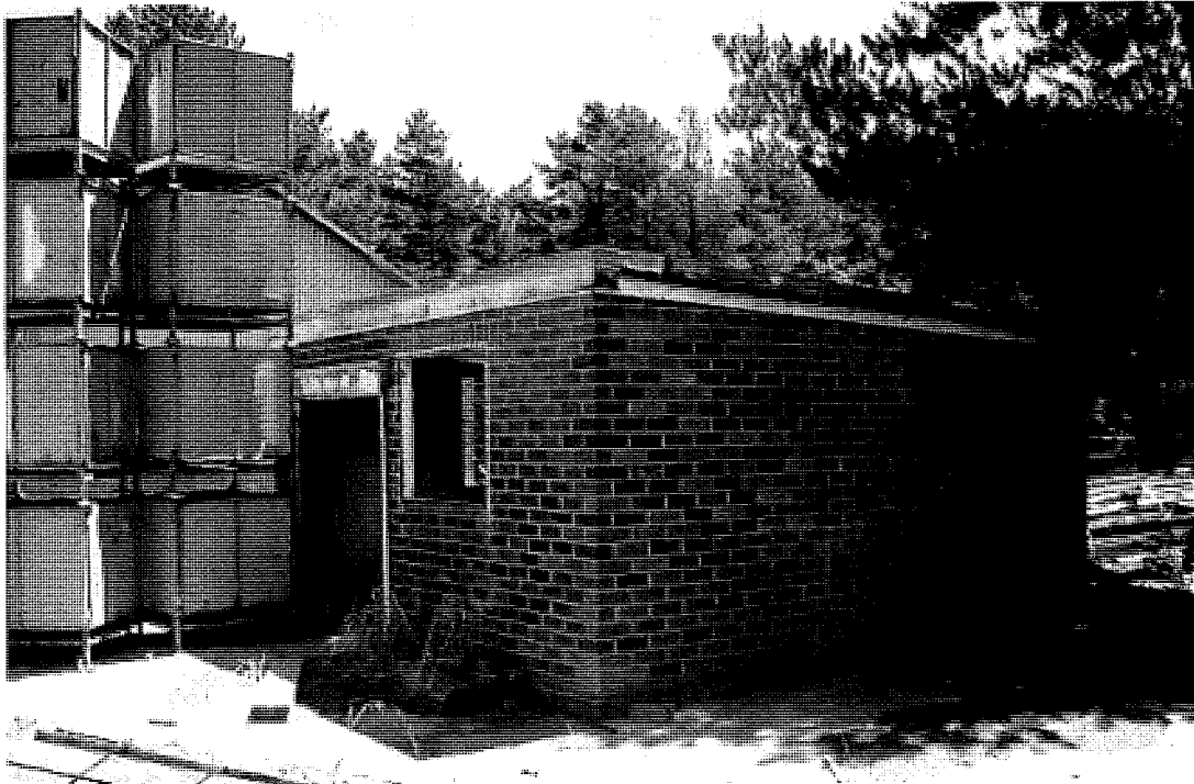
Figure 148 The storage building, adjoining the site of the brick extrusion plant site.
