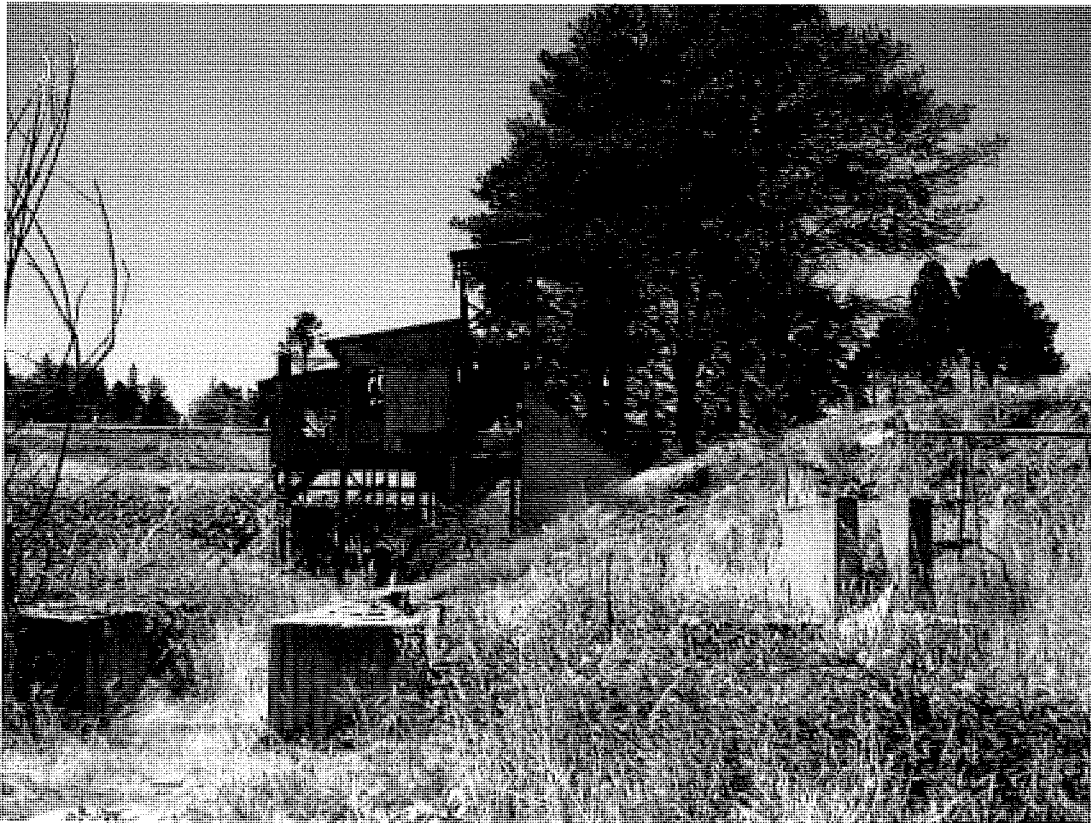
Figure 130 The Primary Crusher House viewed from the west. The concrete footings in the foreground supported the now demolished conveyor which transported crushed material to the Red Pan Room (also demolished) for further refining.
