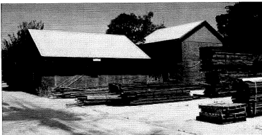
Figure 145 The former boiler house and adjoining substation/control room, photographed from the site of the former extrusion plant. The substation building is at left.
