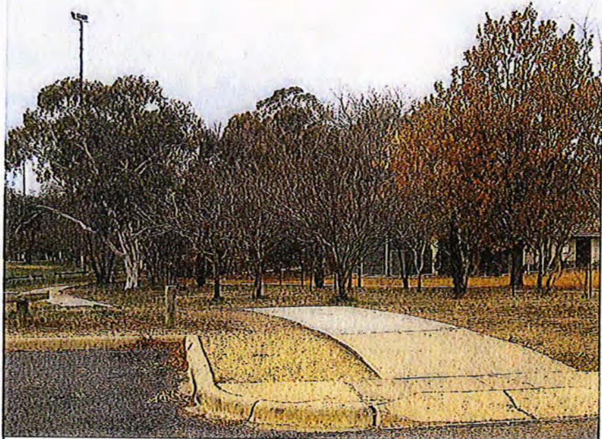
Figure 2.2: Existing path through Block 13 - connection to Rivett shops carpark
