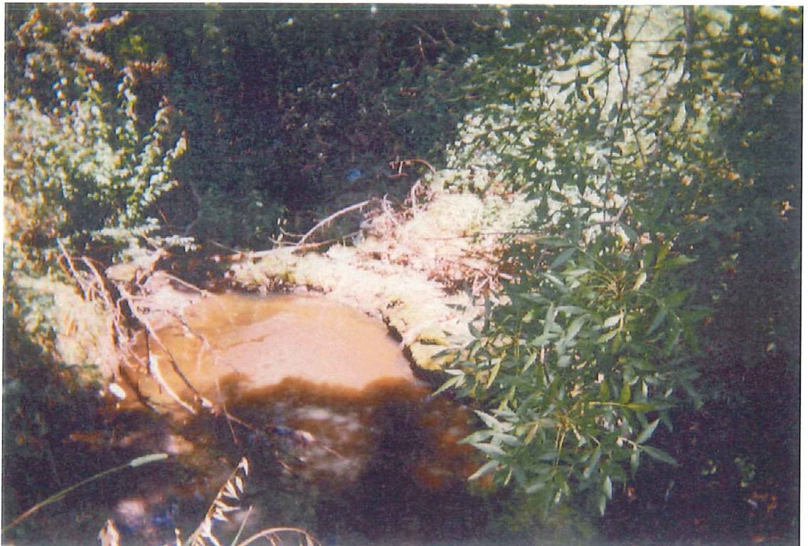
Photo 3: Stormwater drain – no evidence of oil or oil staining.
