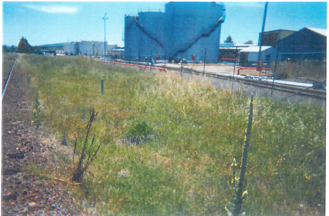
Photo 5: Revegetated areas adjacent to fuel depot sidings. No visual evidence of staining.
