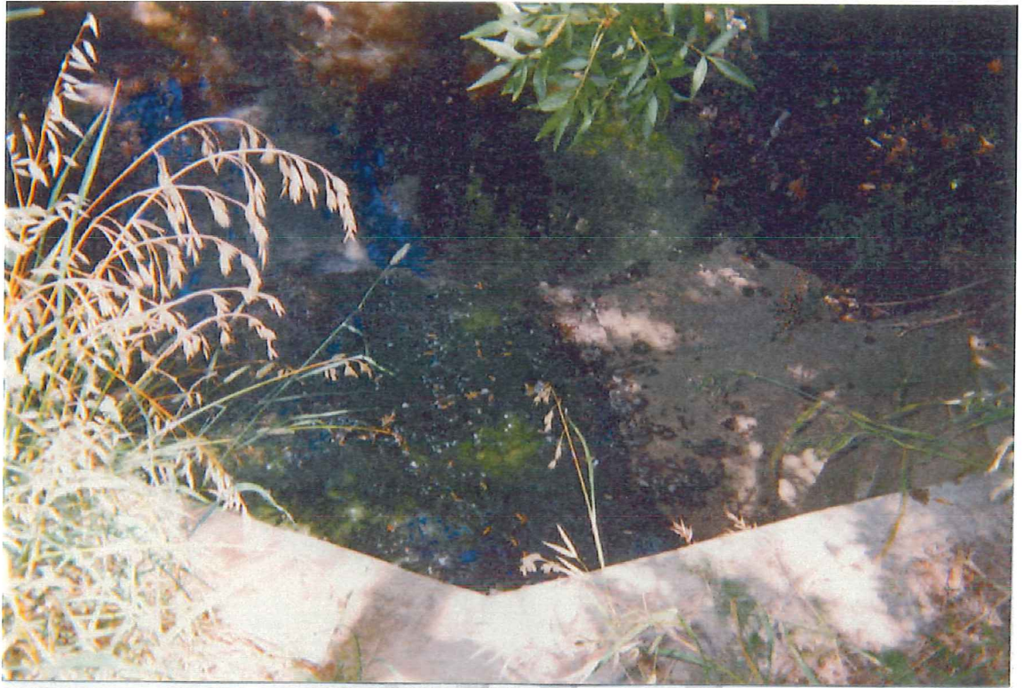
Photo 2: Stormwater drain – no evidence of oil or oil staining.
