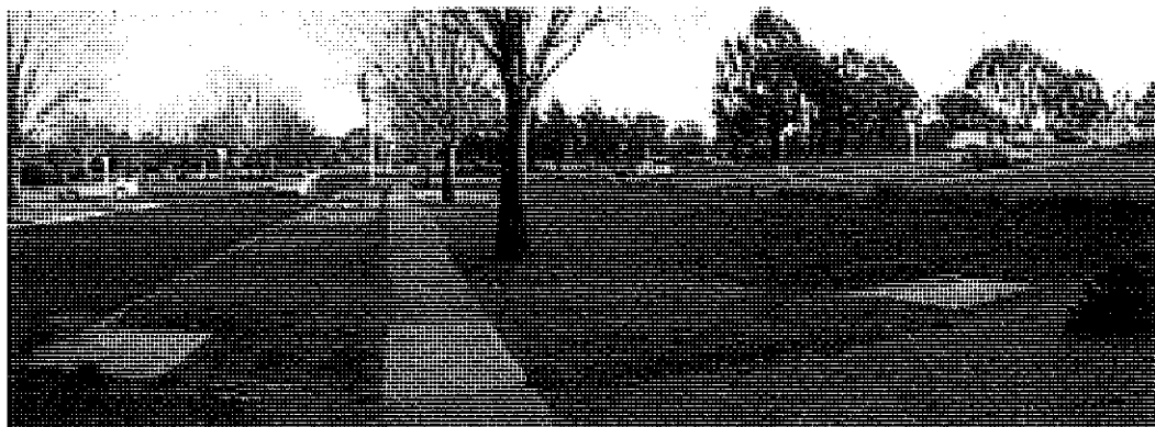
Photograph No. 6a View of Benjamin Way verge. Note the plantation strip to right of photo which collects runoff from the block via the grassed swale along the eastern side of the block. The Benjamin Way verge has a footpath, street trees and street lighting. The proposed sewer connection point is visible to left of photo - refer to sewer maintenance hole located in the pavement of Benjamin Way left of photo.
