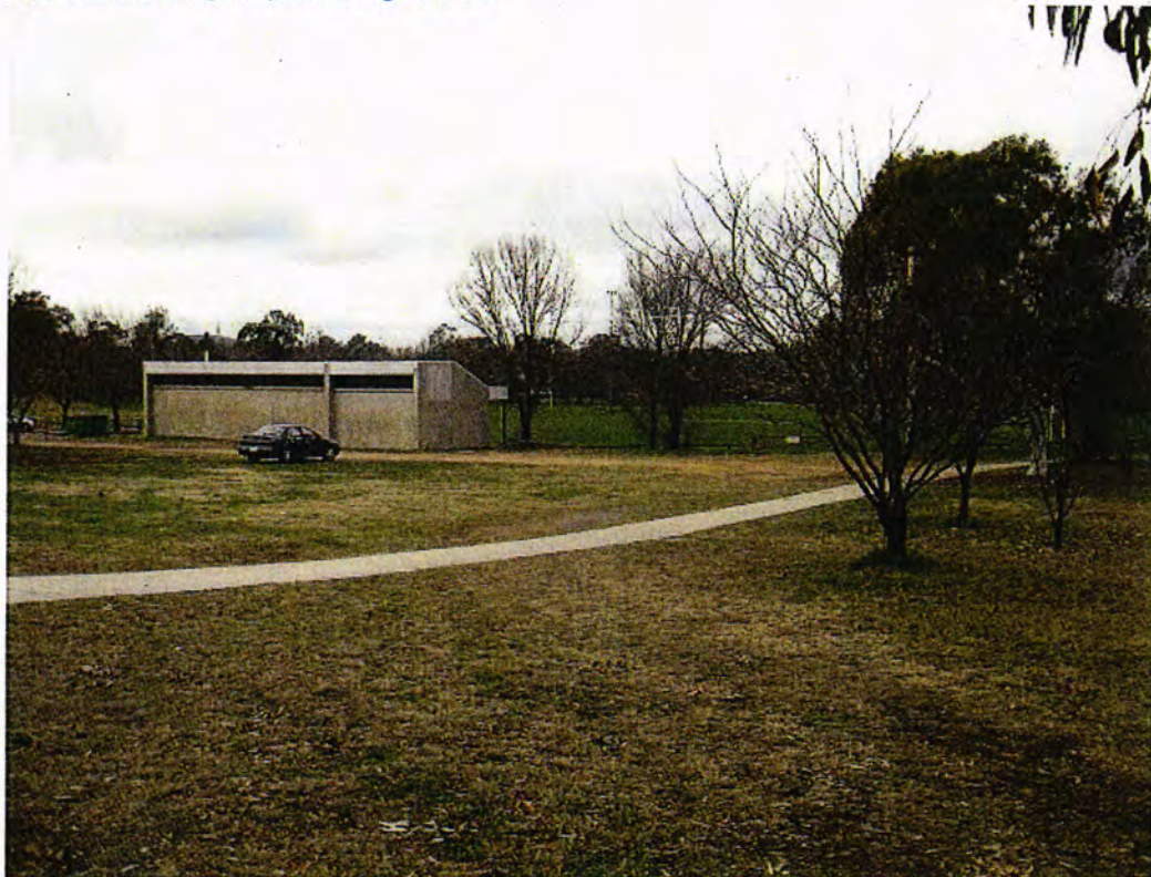
Figure 2.1: Existing footpath through the Site
