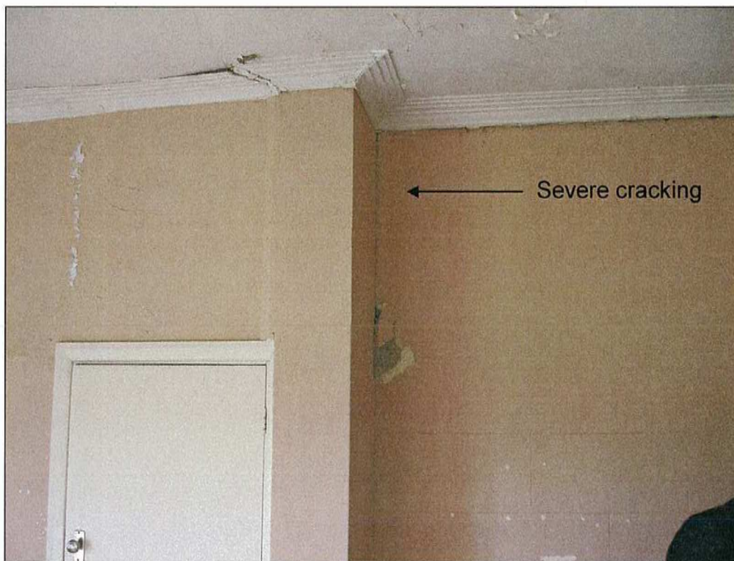
Bed 3 wall as viewed from Bed 4
