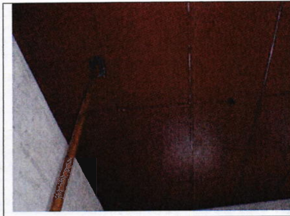
Photograph 19: BH & SS2 - Ceiling sheet Refer Sample: RA M0102
