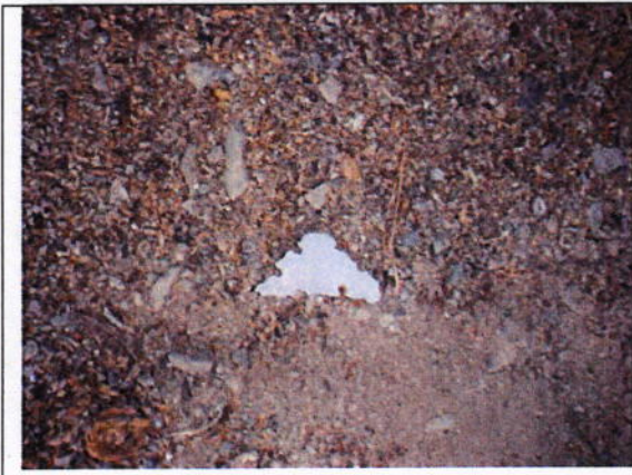
Photograph 15: K2 - Top floor, debris to top floor (small amount left post removal) Refer Sample: M0100
