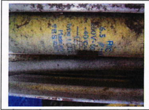
Photograph 33: Former canteen RIC – LE 1 EB
