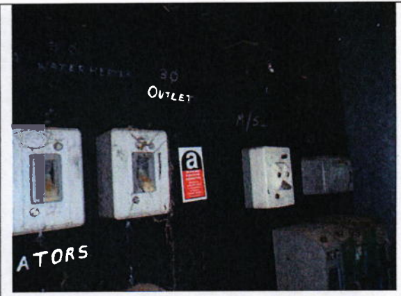
Photograph 20: All switchboard backing sheets throughout site Refer Sample: 7504 – 23 - VA12
