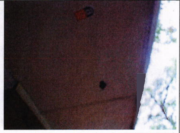
Photograph 6: A4 - Perimeter eave & soffit sheet Refer Sample: 2810 – 40 – A9
