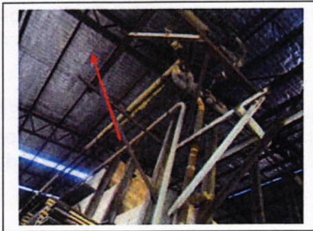
Photograph 25: To underside of roofs throughout Refer Sample: 3617 – 103 – S2
