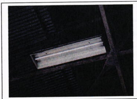
Photograph 32: Building H Inaccessible
