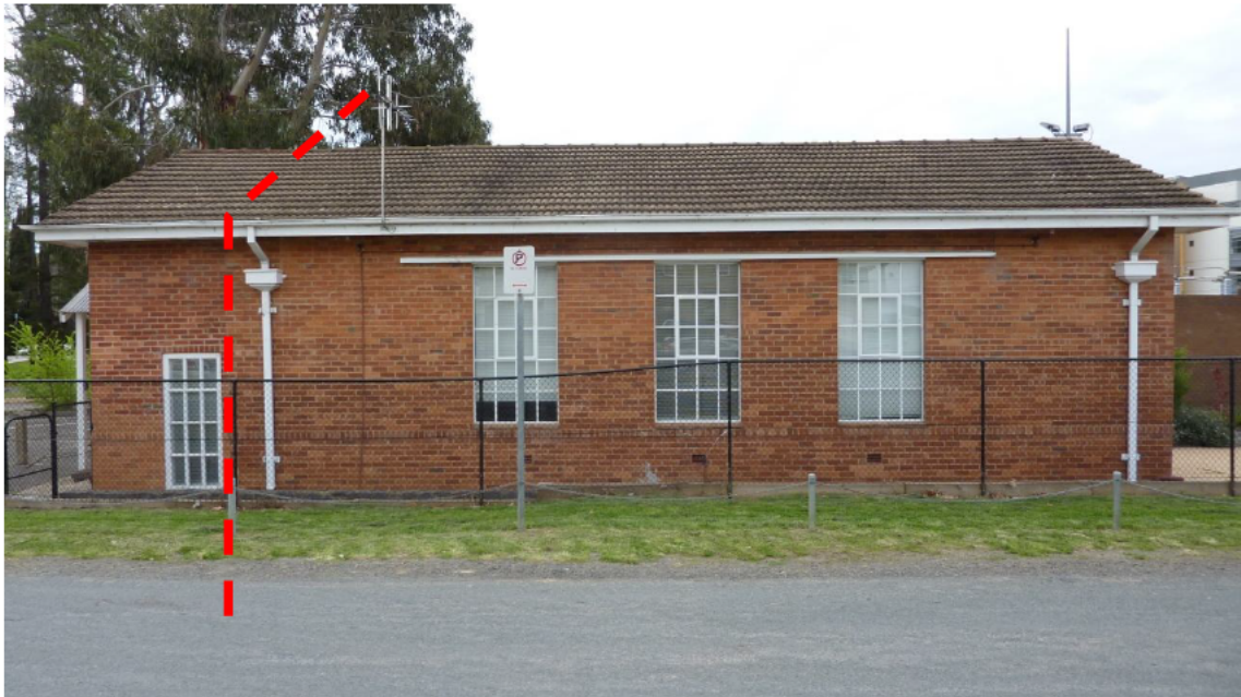
Figure 6 South-east elevation: the later addition is indicated.
