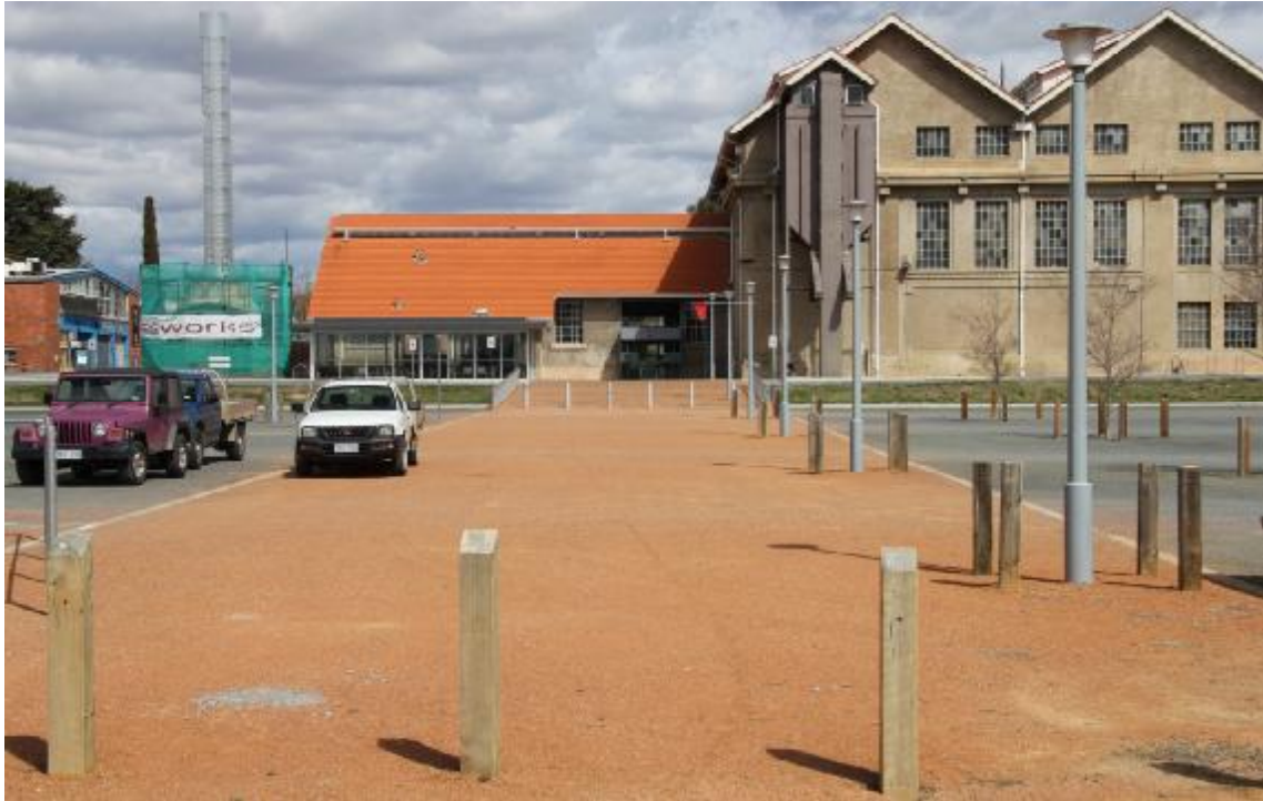
Figure 7 North-east elevation of the Power House 2012.
