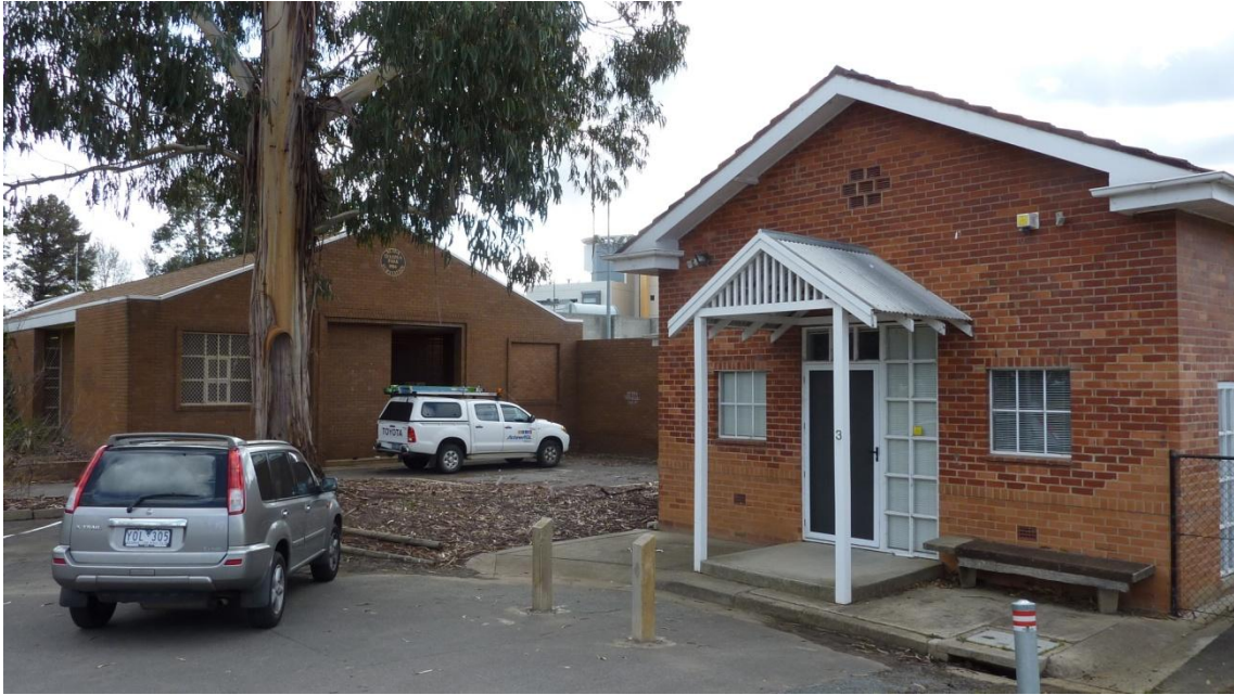
Figure 7 View looking north from the entrance to the '1948 Switch Room': the entry to the Telopea Park Substation is to the rear.
