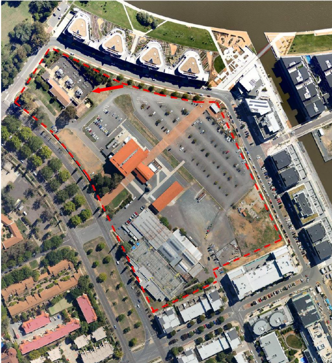
Figure 1 The Kingston Section 49 Master Plan area with the Switch Room arrowed.
