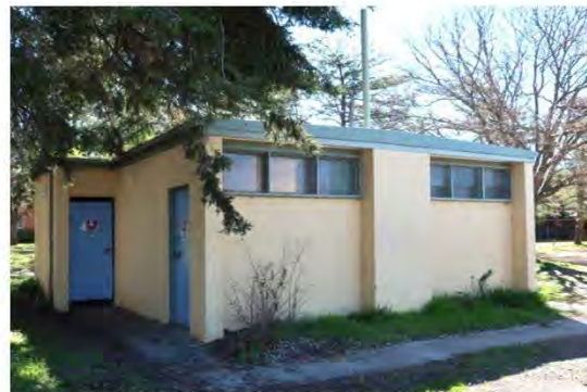
Figure 43: East part of toilet block
