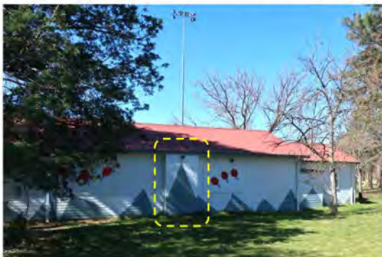
Figure 35: West elevation, south end with brick chimney breast (indicated)
