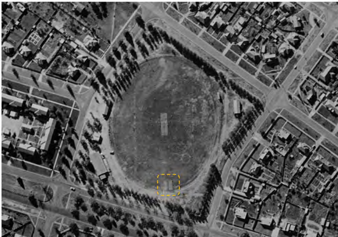
Figure 15: Aerial showing the Kingston Oval with a gable building to the east corner (1958) An area which may have been used as cricket nets is indicated (Source: Geoscience Australia , CA145, frame 5118)
