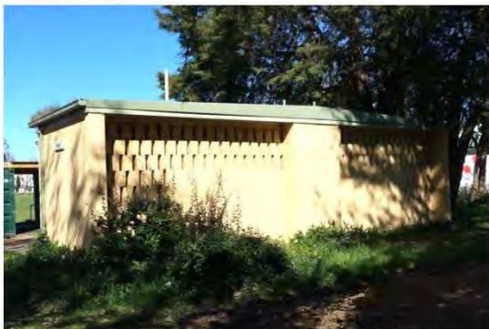
Figure 42: West part of toilet block with open blockwork
