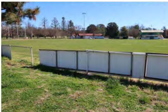
Figure 46: Pipe rail fence with advertising signage to east side
