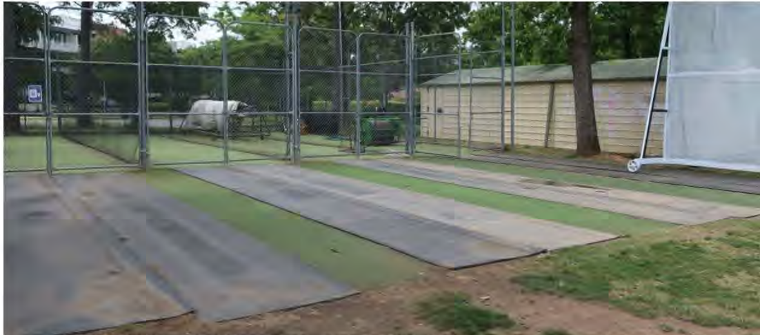
Figure 63: Cricket nets with stored covers and roller. There is rubber matting leading to the nets with wear and tear evident to the adjacent turf
