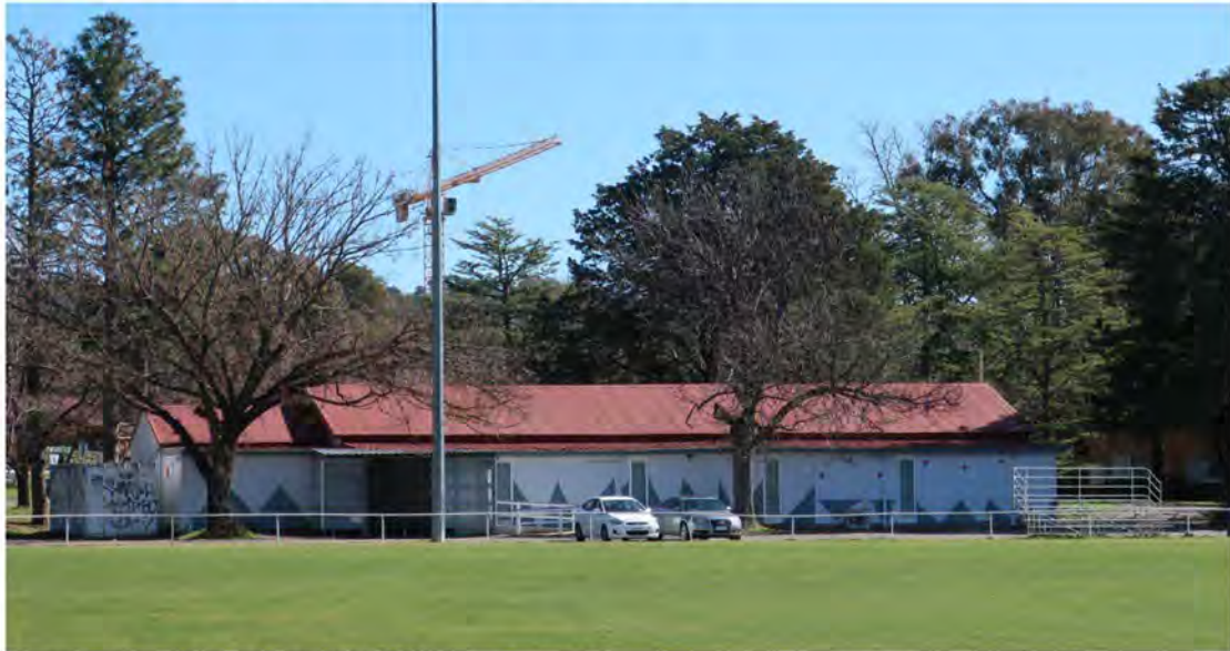
Figure 34: View of Table Tennis Centre from oval, east elevation
