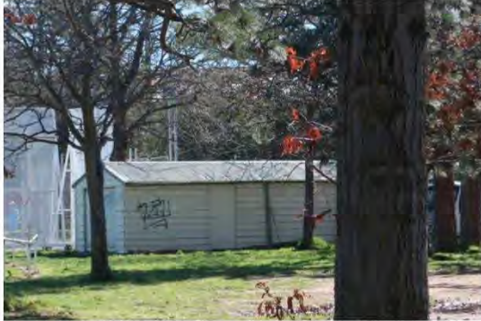
Figure 44: West part of toilet block with open blockwork
