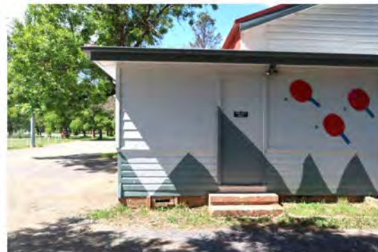
Figure 39: Part north elevation with skillion roof returning partway across the gable end
