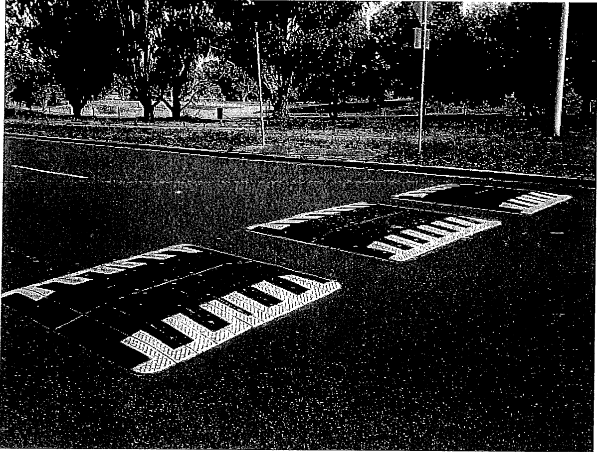
A set of speed cushions on Spofforth Street
