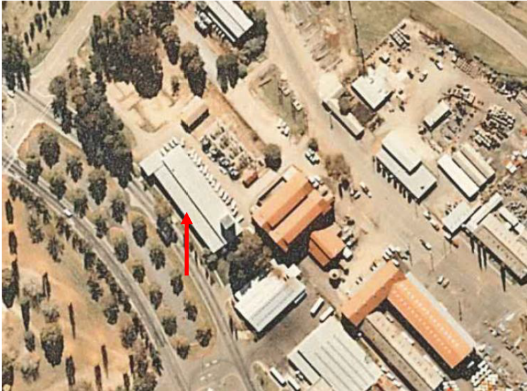
Figure 23 Aerial 1975. The Engineering Services Workshop (1963) is indicated. Source: ACTPLA.
