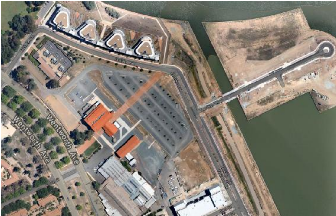
Figure 36 Aerial view of Kingston Section 49, January 2010. Source: www.nearmap.com
