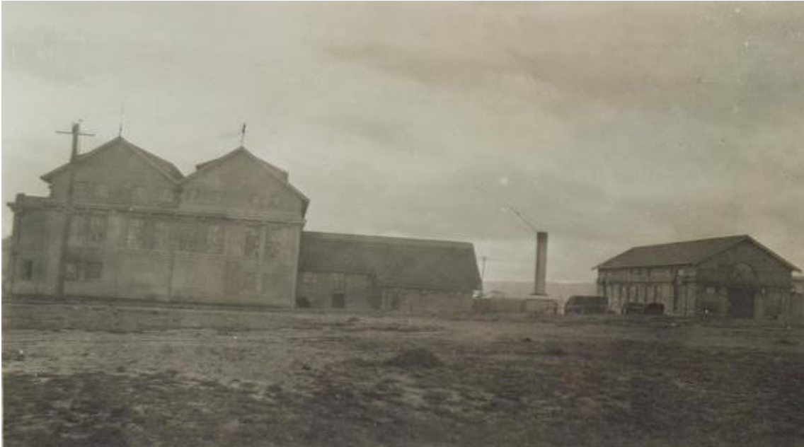
Figure 14 The Power House and Fitters' Workshop viewed from the west, c. 1916. Source: National Library of Australia.
