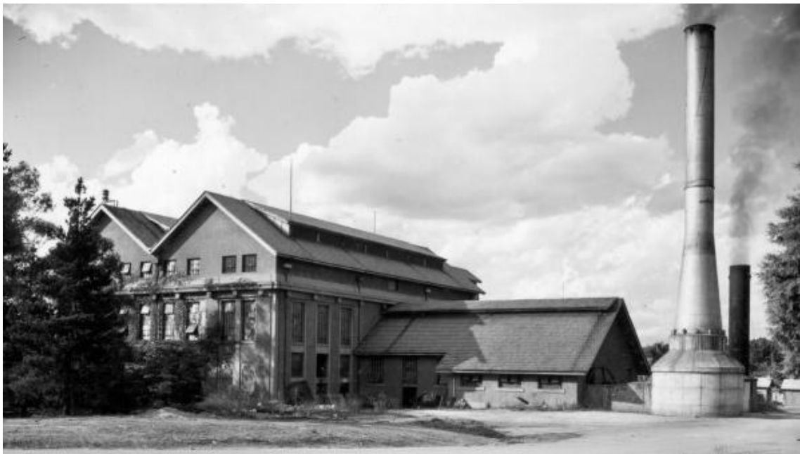
Figure 20 The Power House viewed from Wentworth Avenue, 1951. The 1940s stack is in the foreground. Source: ACT Heritage Library.
