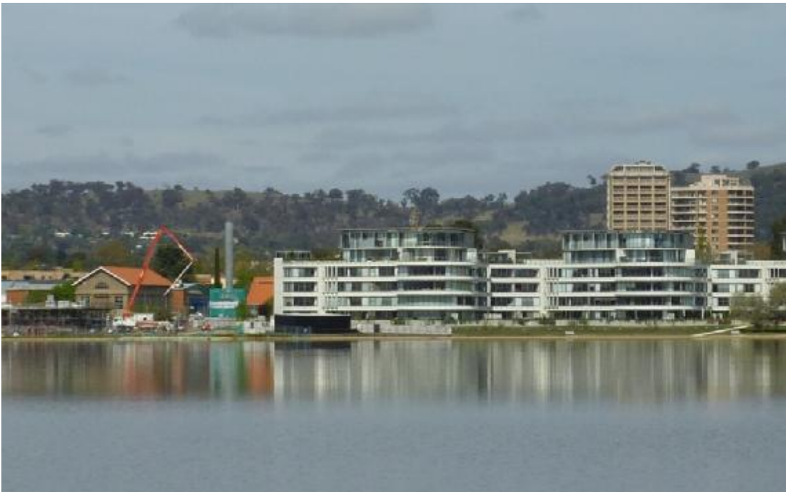
Figure 35 View of Kingston Section 49 from Grevillea Park, on the north bank of Lake Burley Griffin (October 2011).
