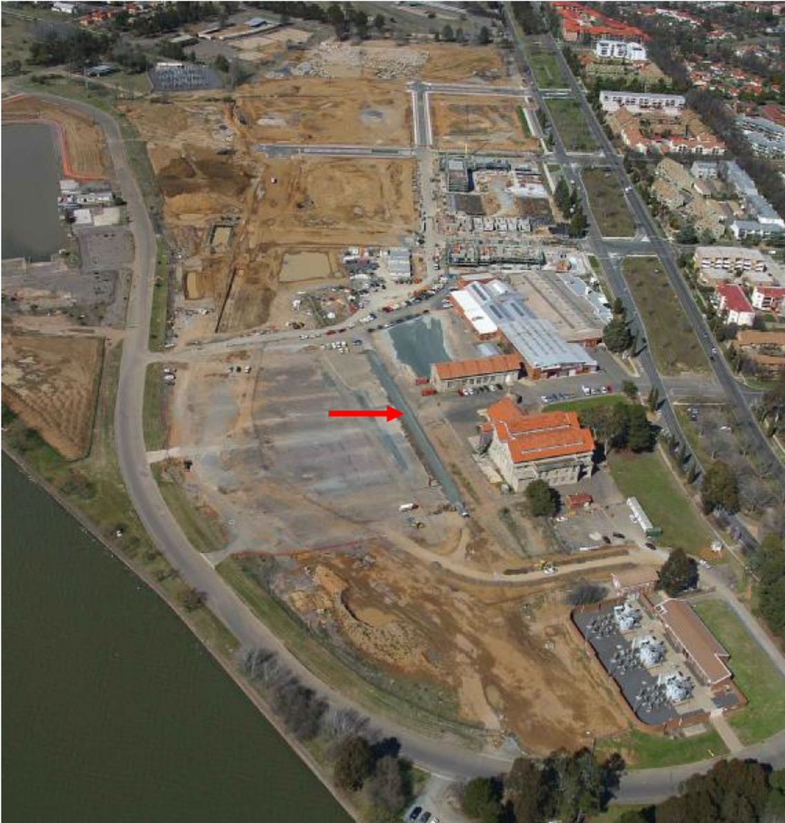
Figure 27 Oblique aerial looking south across Kingston Section 49 (c. 2003). The alignment of the 132kV cables is indicated. Source: LDA.
