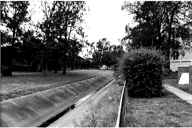
Figure 6.81 Landscaped open channel to the north of the overall site
