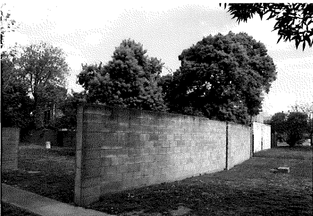
Figure 6.31 Curved walls facing Northbourne Avenue which serve to screen the Paired Houses
