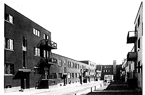
Figure 3.21 Bornheimer Hang Siedlung, Frankfurt, 1927 Source: Quiring, Ernst May
