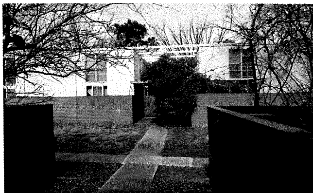
Figure 6.25 View of Paired Houses showing the courtyards and internal pathway network through the site
