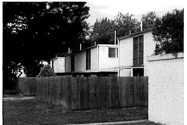
Figure 6.32 View of Paired Houses grouping
