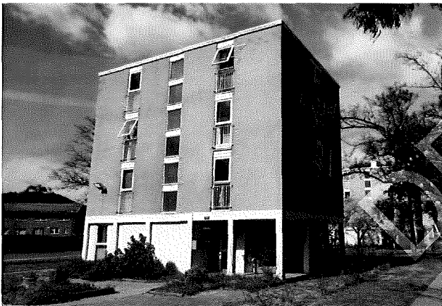
Figure 6.14 Exterior of Bachelor Flats, showing building entrance
