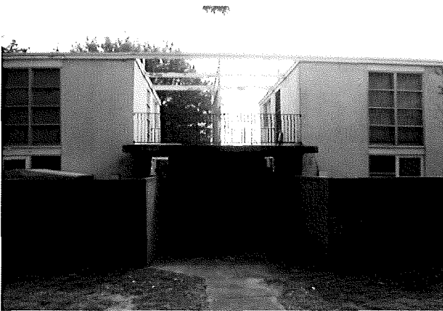
Figure 6.29 Carport space adjoining Paired Houses
