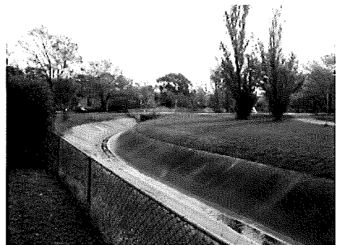
Figure 6.2 The stormwater drainage channel fringing the Northbourne site
