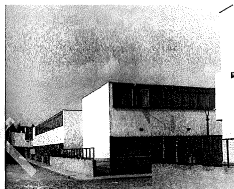
Figure 3.11 JJP Oud, Kielhoek Workers' Housing, Rotterdam, 1925
