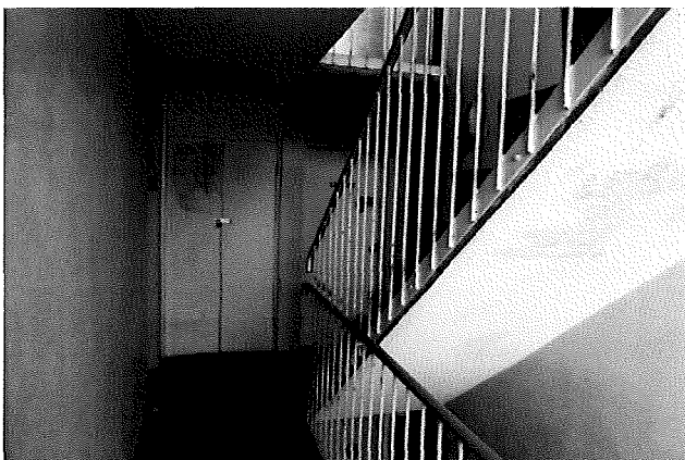
Figure 6.49 Owen Flats: Internal stairs and landing
