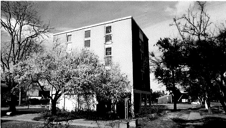
Two of the three buildings were built in close proximity to the Northbourne Avenue frontage, reinforcing the "gateway" nature of their role.
