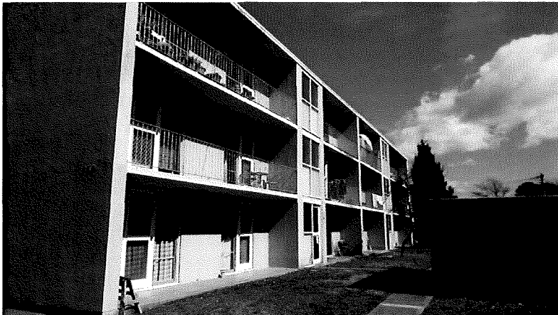
Figure 6.34 The north facing elevations are enlivened by a regular pattern of deep horizontal balconies and vertical stair wells.
