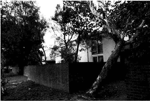
Figure 6.75 Some of the major trees are in poor condition
