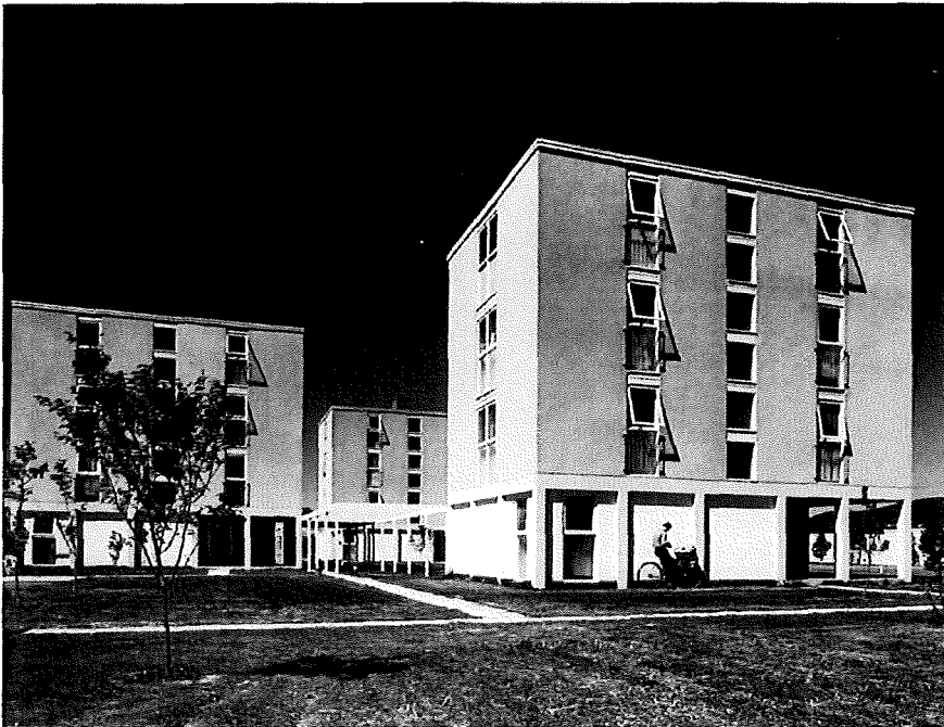
Figure 5.12 Bachelor Flats Source: National Archives of Australia
