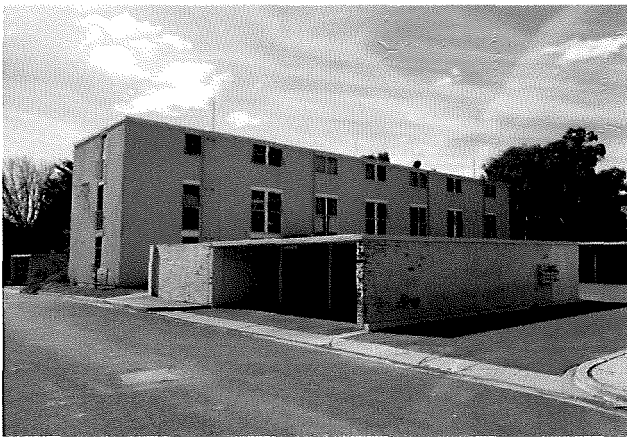
Figure 6.38 Freestanding separate carport for each flat, located behind the southern elevation of the dwellings
