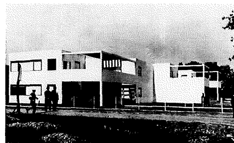
Figure 3.9 Pessac housing estate (1926), Le Cobusier Source: Le Corbusier, 1910-1929
