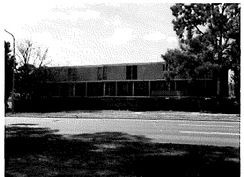
Figure 6.7 The Karuah Maisonettes on the eastern side of Northbourne Avenue screened the rows of single storey Garden Flats from Northbourne Avenue.
