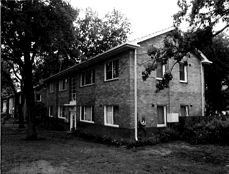
Figure 4.4 Griffith Flats, showing the building articulation with its regular window pattern, the building entry and glassed stairwell
