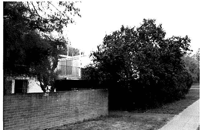
Figure 6.72 Landscaping and garden wall around Paired Houses
