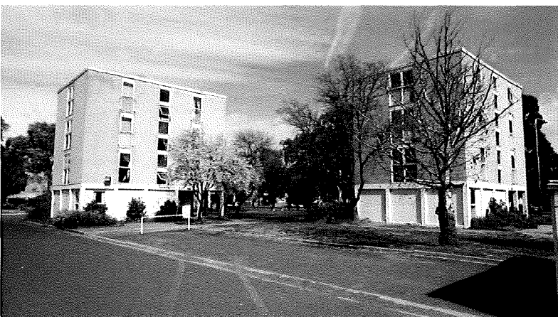
Figure 6.11 View of the group of three flats buildings from the internal access driveway
