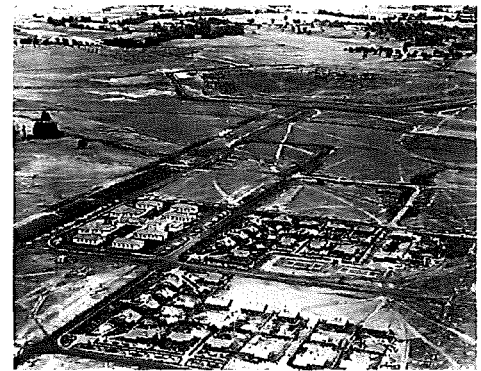
Figure 2.5 The first group of permanent homes in Braddon, early 1920s Source: Wright, Cornerstone of the Capital
