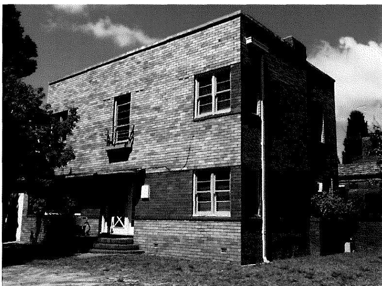
Figure 4.2 Forrest Fire Station
