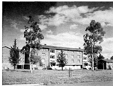
Figure 4.38 Stuart Flats, 1966 Source: National Archives of Australia
