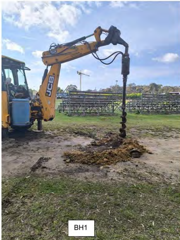
Plate 2-1: Drilling of BH1 and BH2
